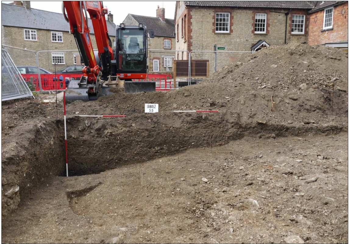
Figure 12. Overview of Section 5, facing SW
