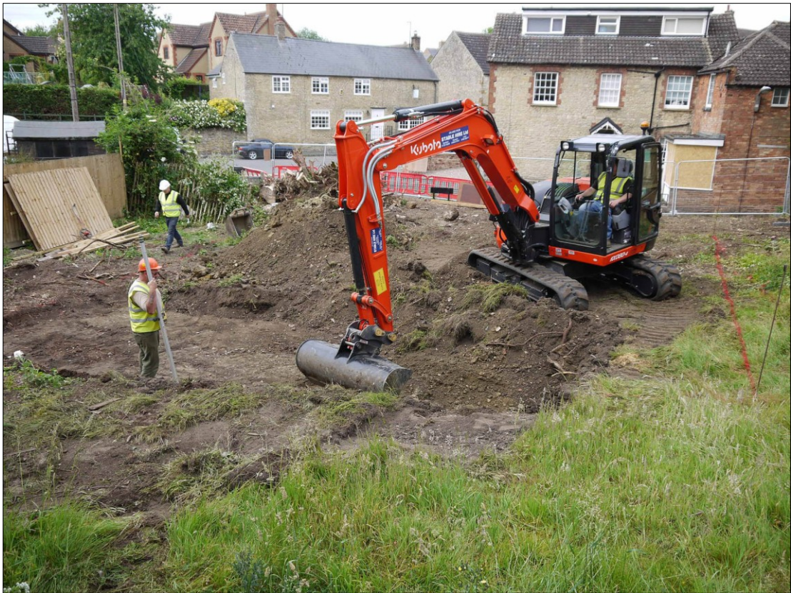
Figure 3. Overview of the site at commencement of soil strip, facing S
