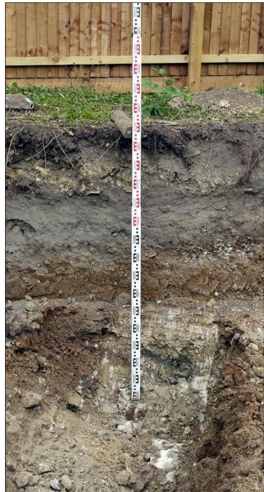
Figure 4. Geotechnical test pit in W corner of site, showing depth to bedrock. Facing NW
