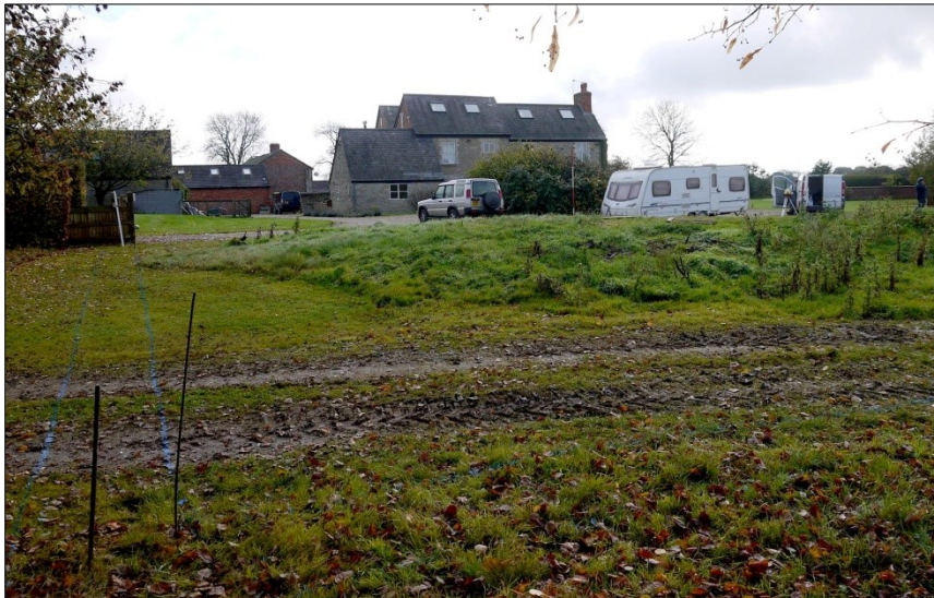
2. Pre-excavation, facing SE
