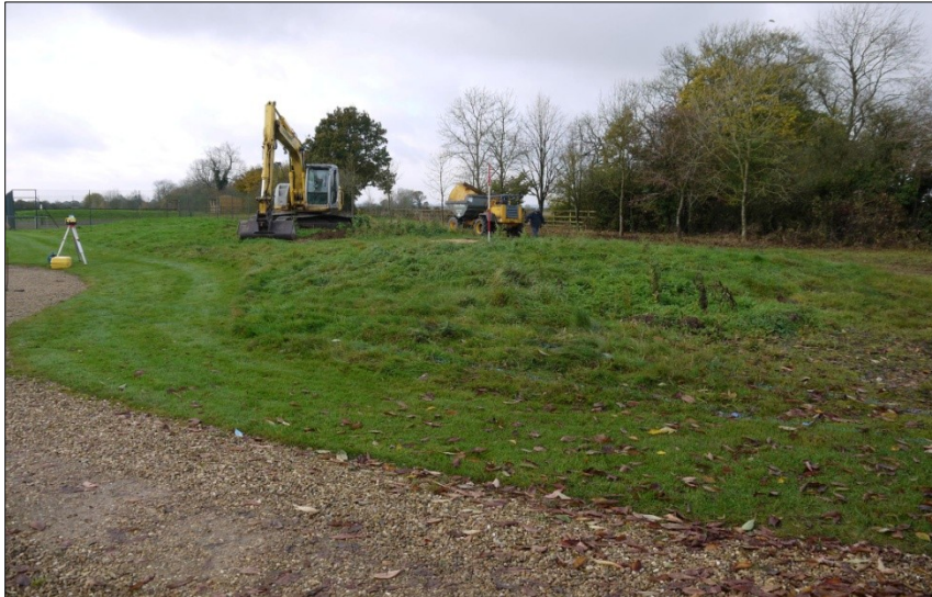
1. Pre-excavation, facing W
