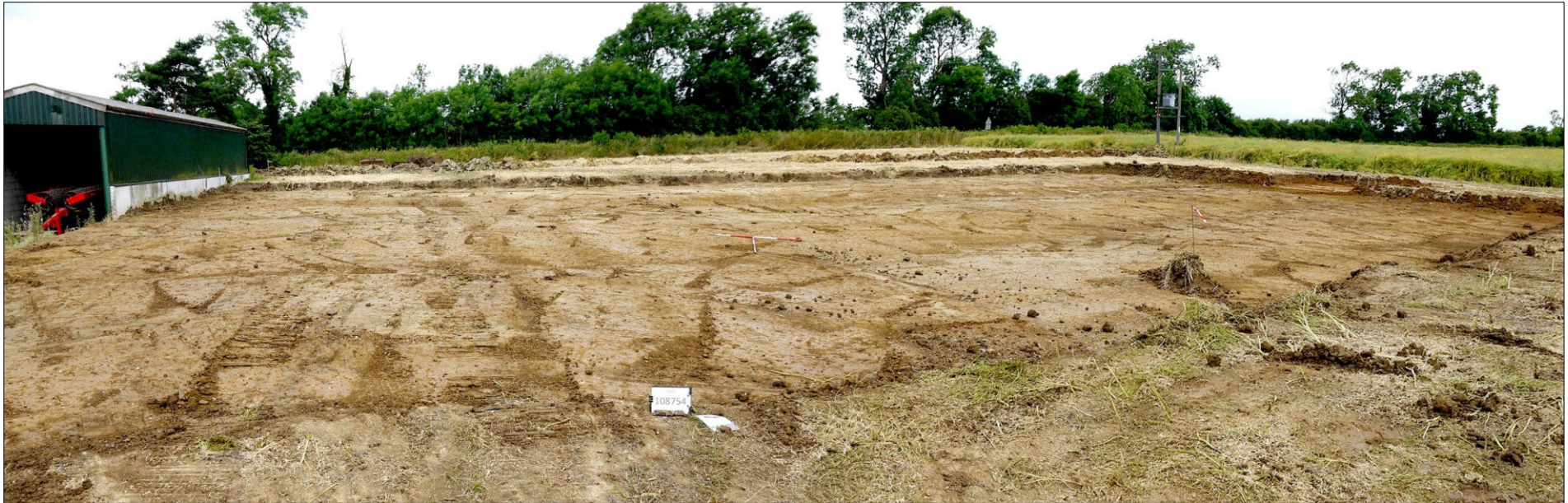
7. Overview of site after soil strip. Facing NW
