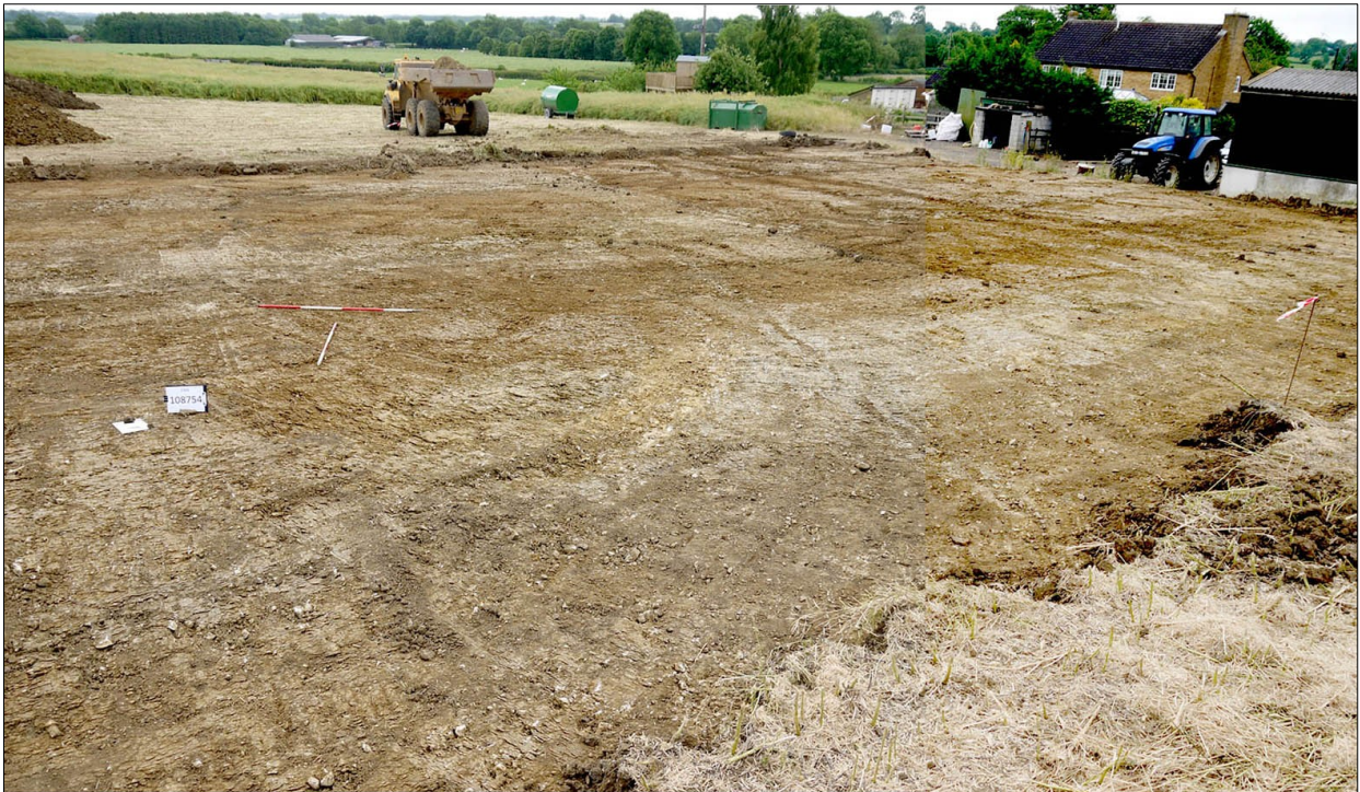
3. Overview of site after soil strip. Facing SE
