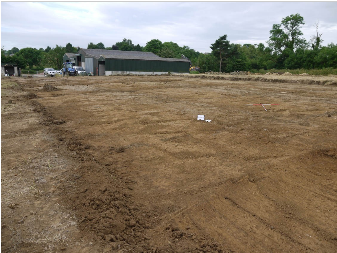
6. Overview of site after soil strip. Facing SW
