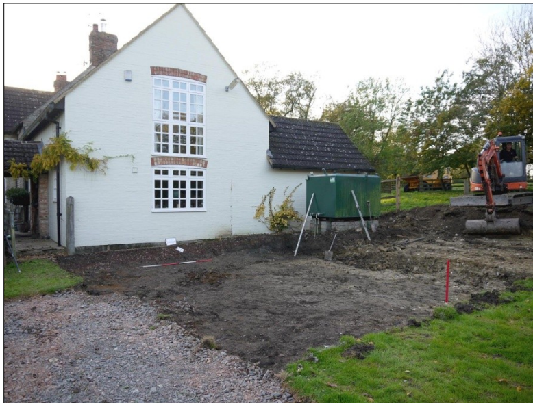
Figure 4. Area of ground reduction. Facing southwest
