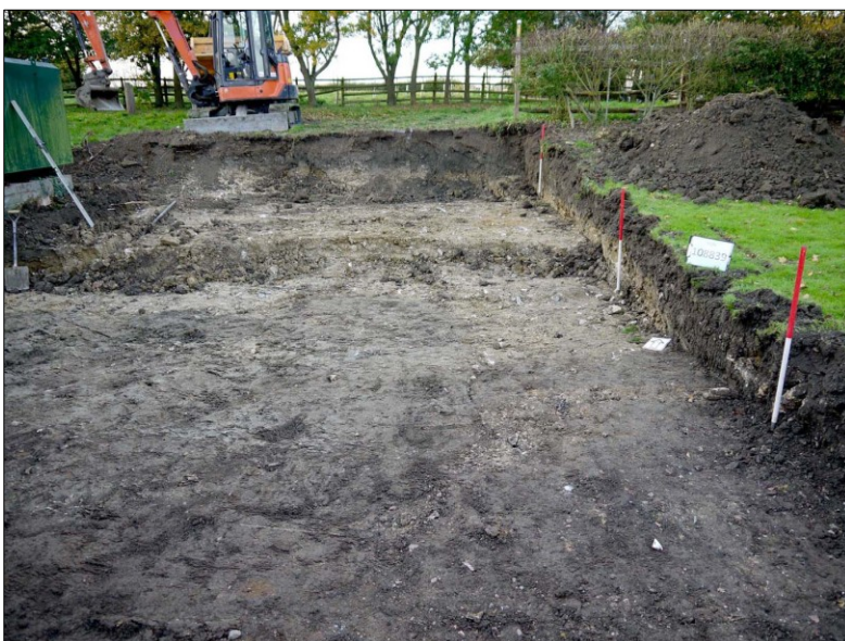
Figure 5. Area of ground reduction. Facing northwest
