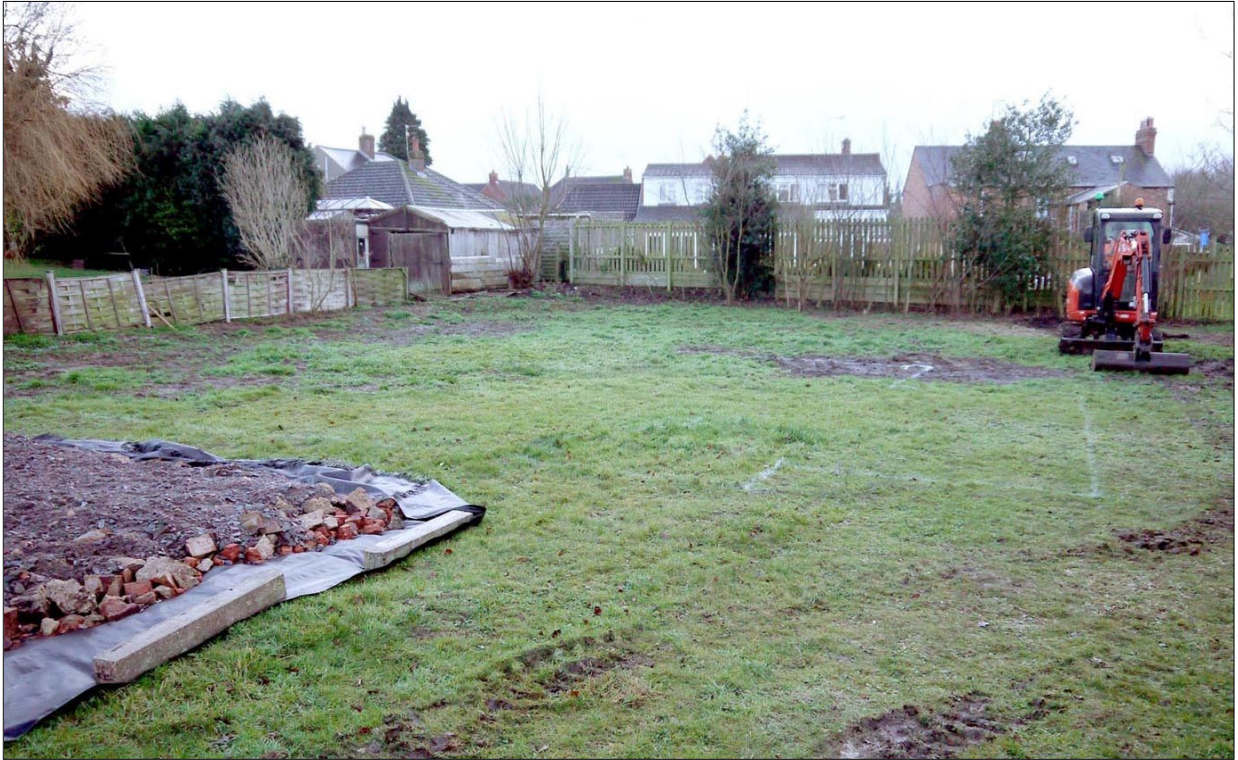
1. Overview of the site prior to ground reduction. Facing ESE
