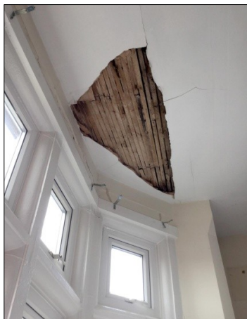
118. Room 15. Lathwork exposed above window bay
