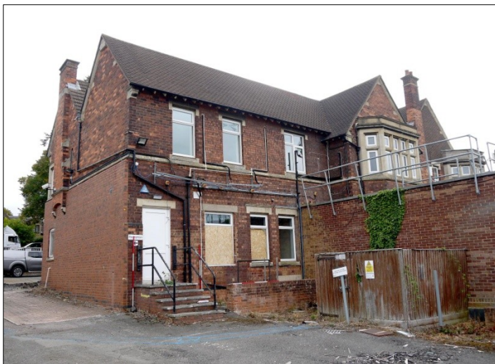
42. Rear aspect of the west elevation (northern end). Facing SE
