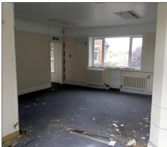
104. E-W Wing. Room 12. Facing NW
