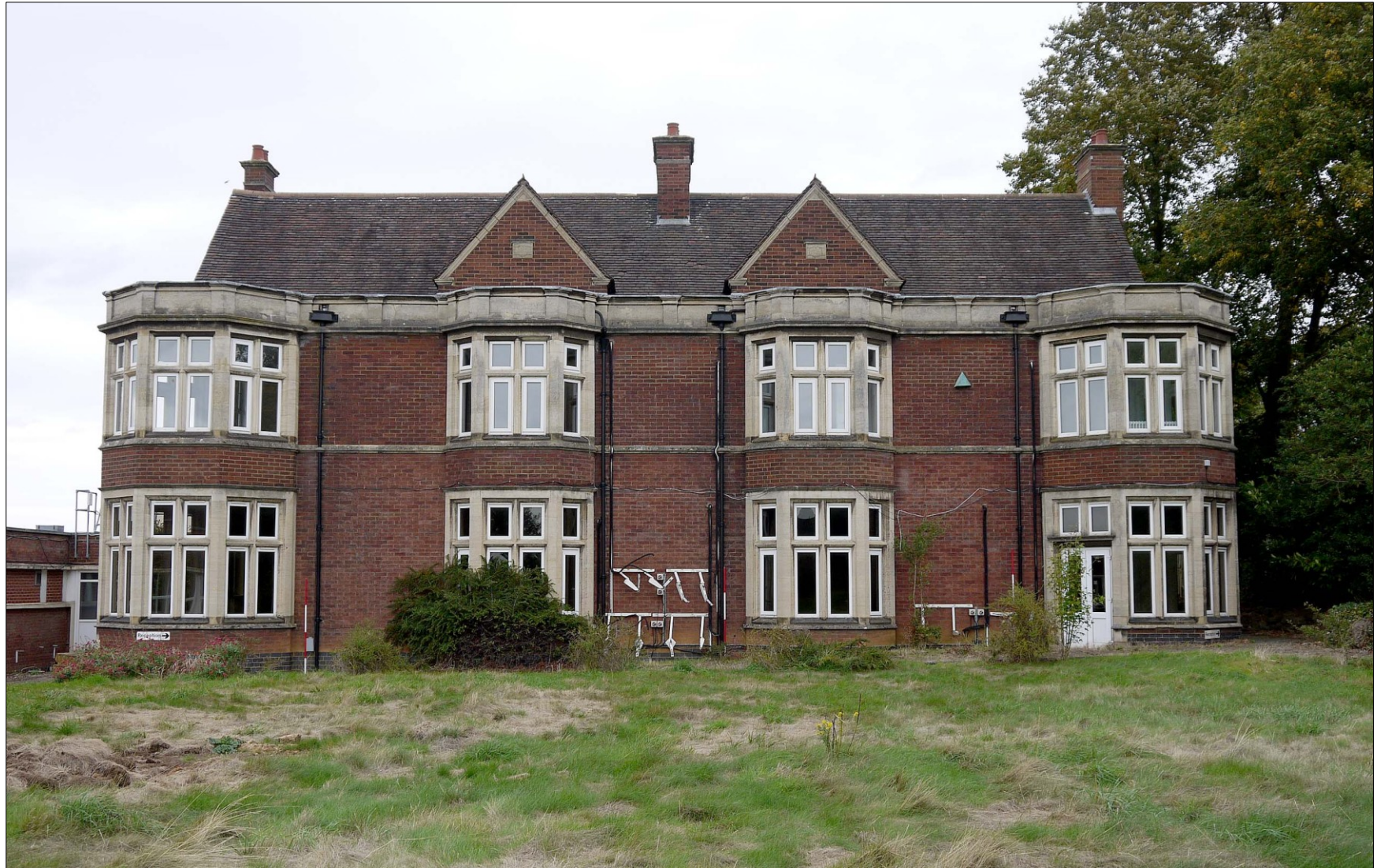
14. E-W wing. Overview of the rear (S) elevation. Facing N
