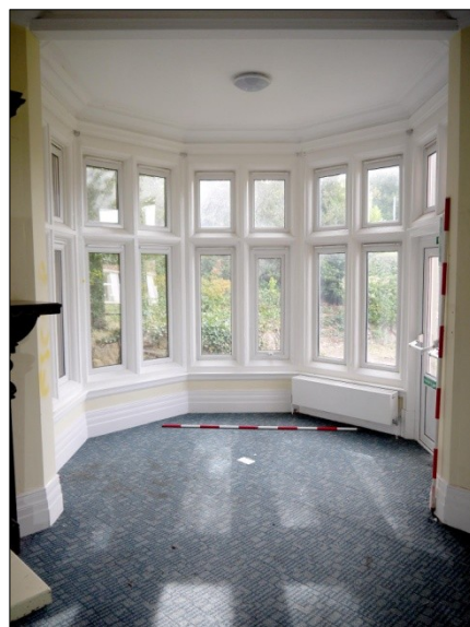
56. E-W Wing. Room 2. 5-sided bay window (SE turret) overlooking rear garden. Facing SE
