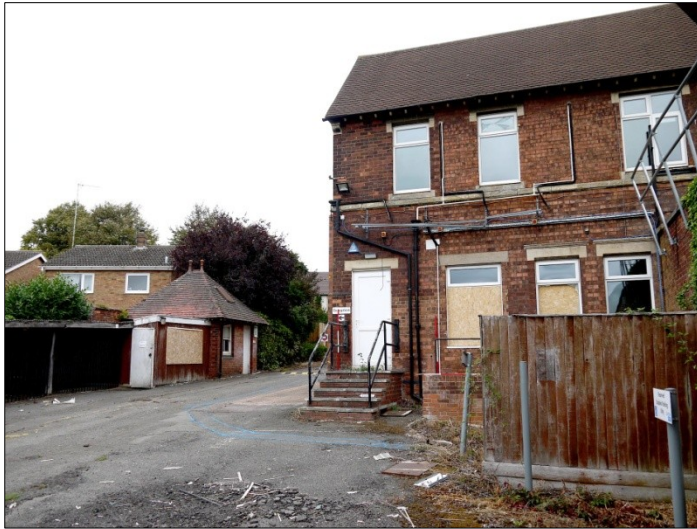
41. Rear aspect of the west elevation (northern end). Facing NE
