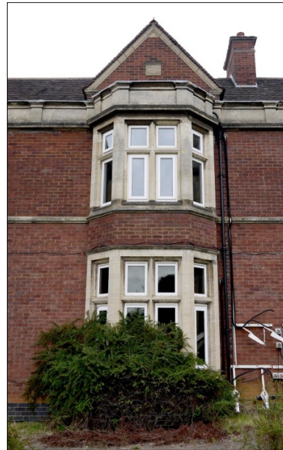
17. Two-storey bay window (W half of wing)
