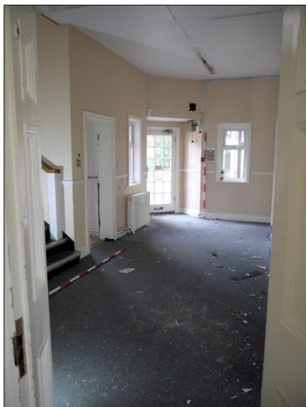
53. E-W Wing. Room 1. Vestibule. Facing E
