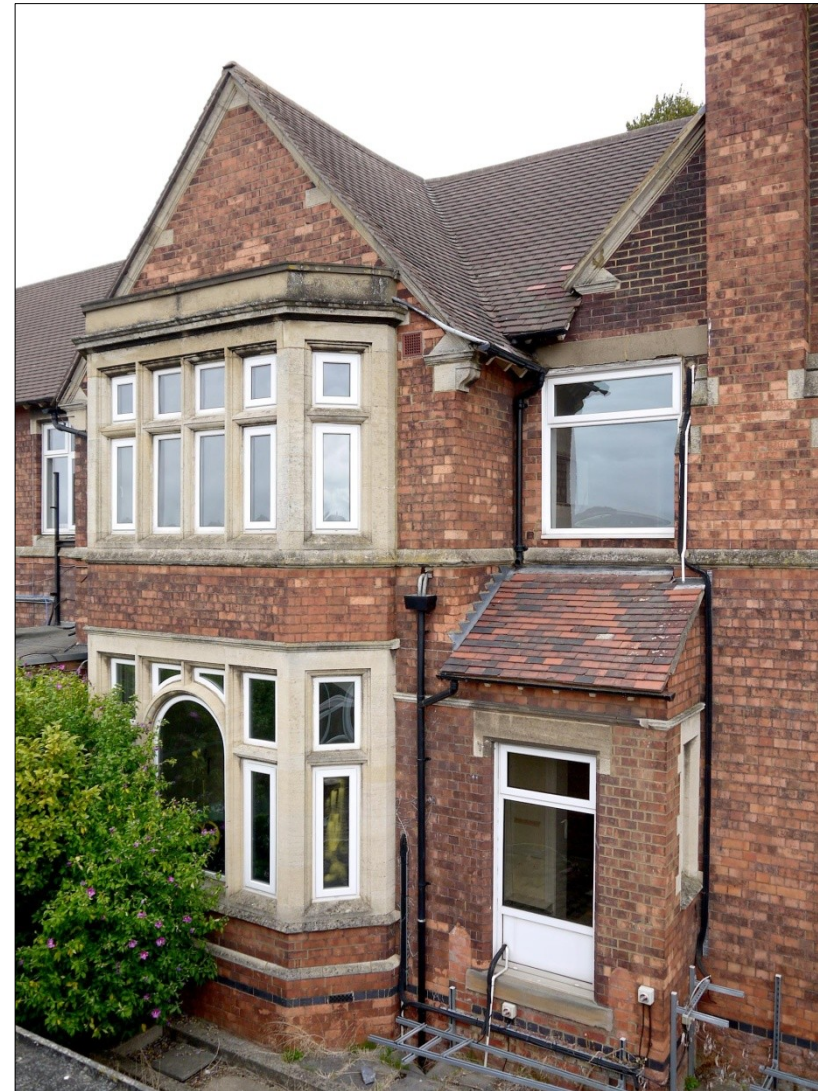
30. N-S wing. Gable with two storey bay window of the late 19 th century building. Facing NE
