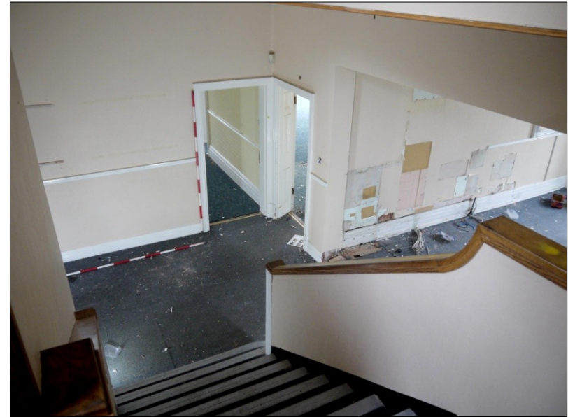
95. N-S Wing. Stairway. View towards vestibule (Room 5 to right) Facing SW
