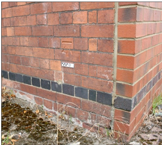
49. East elevation. Carved O.S benchmark near NE corner
