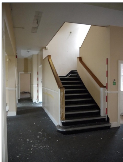
86. N-S Wing. Central corridor and stairway. Facing N
