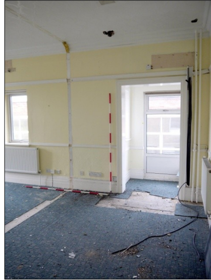
73. Room 4. Facing SW Former rear entrance (to right).
