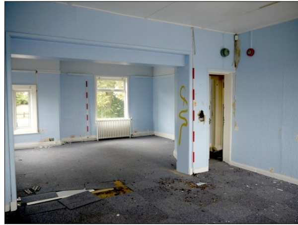
138. N-S Wing. Room 17W (bedroom) View towards Room 17E. Entrance from corridor to right. Facing SE
