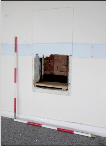
90. N-S Wing. Room 6. Former window opening in north wall.
