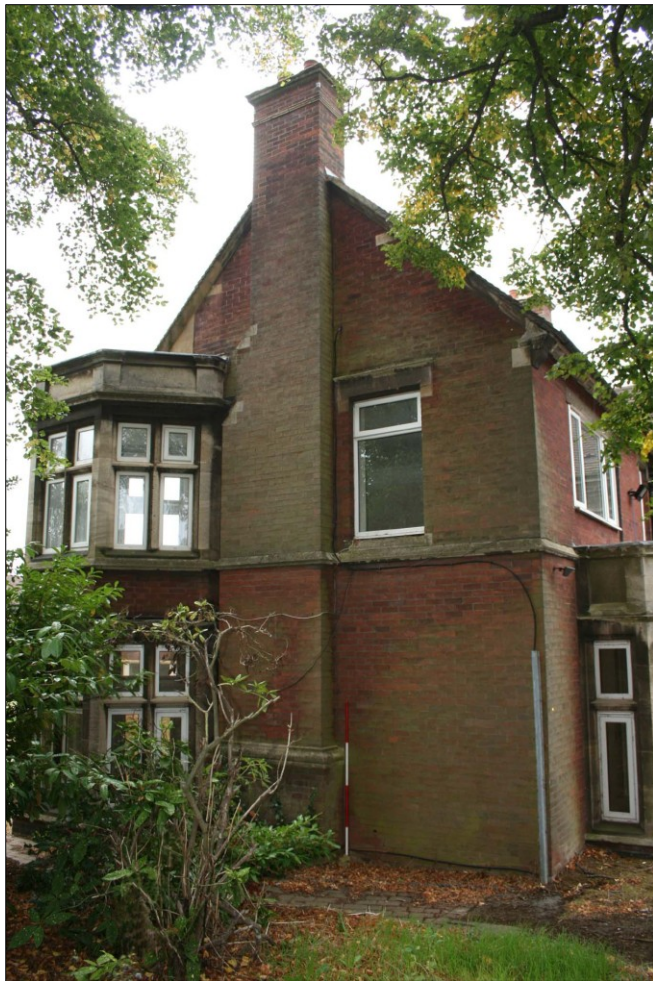
9. E-W wing, eastern elevation. Facing SW
