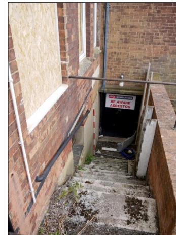
39. Basement access. Facing S
