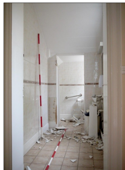
88. E-W Wing. Room 10. W.C. beneath stairway. Facing N
