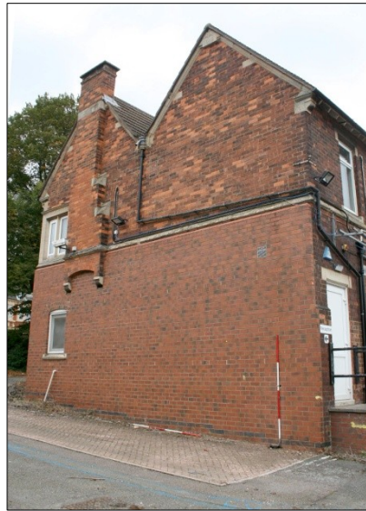
43. North elevation. Facing SE
