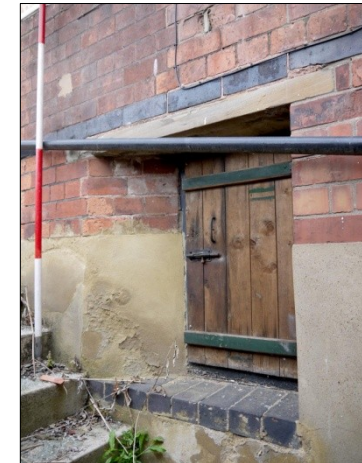
40. Side hatch /light to basement. Facing NE
