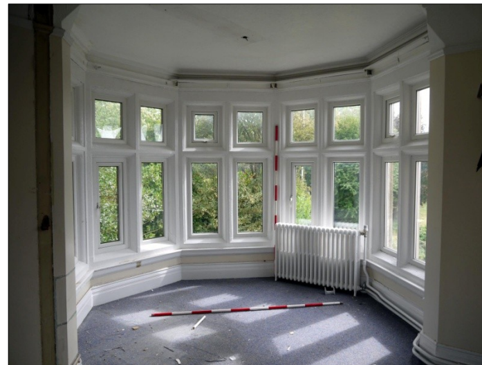
103. E-W Wing. Room 12. 5-sided bay window (SE turret) overlooking rear garden. Facing SE
