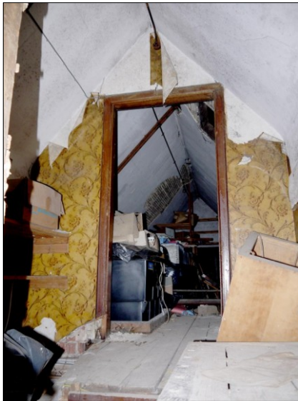
140. N-S Wing. Wall-papered attic room (east side of roof). Facing S
