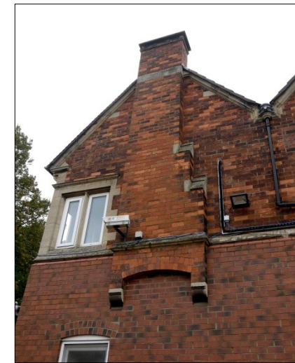
46. North elevation. Corner window and external chimney breast
