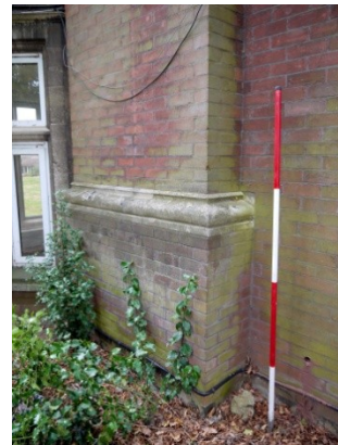
11. E-W wing, Chimney buttress. Facing SW
