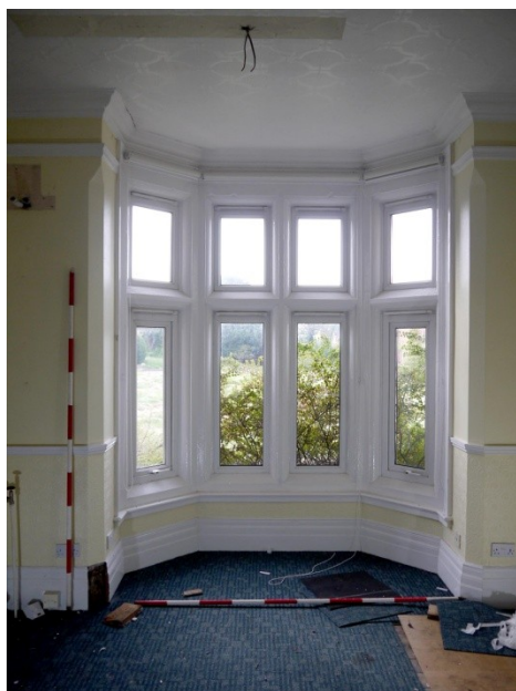
69. E-W Wing. Room 3. Living room. 3-sided bay window overlooking rear garden. Facing S
