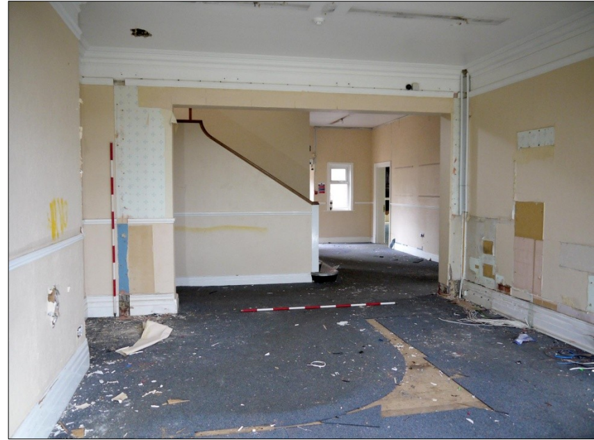
82. N-S Wing. Room 5. View towards vestibule. Facing SE
