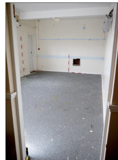
89. N-S Wing. Room 6. Overview, Facing N
