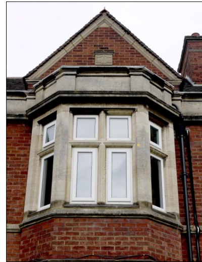
19. Upper bay window & parapet (W half of wing)
