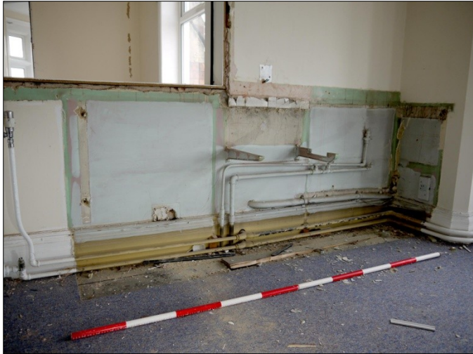
121. N-S Wing. Room 15. Residual décor: site of wash-basin and fitted cupboards in south wall. Facing SW
