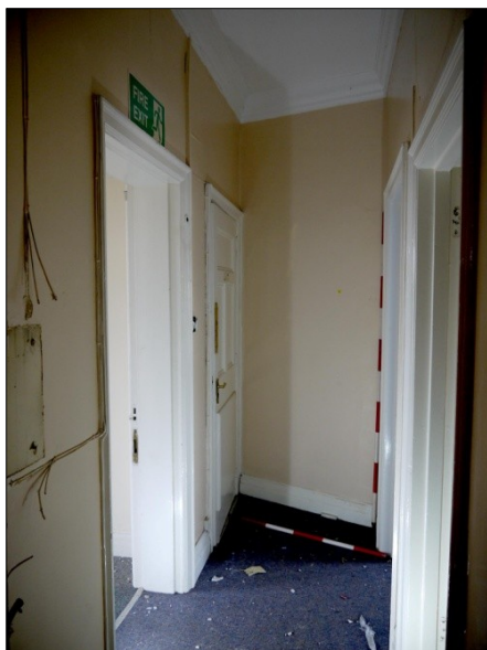
131. N-S Wing. Angled terminus of central corridor Facing N
