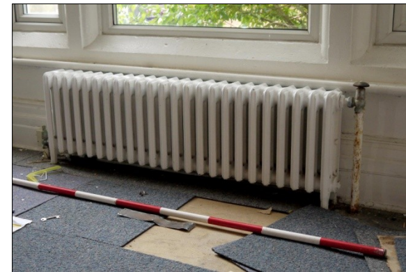
83. Cast-iron radiator in window bay. Facing SW
