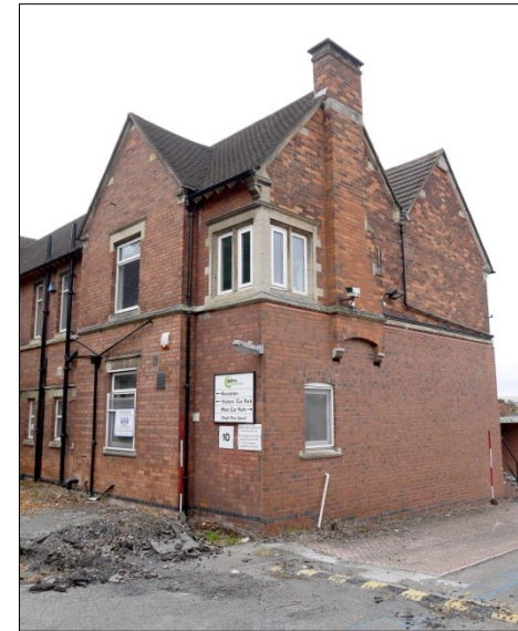
44. North elevation. Facing SW
