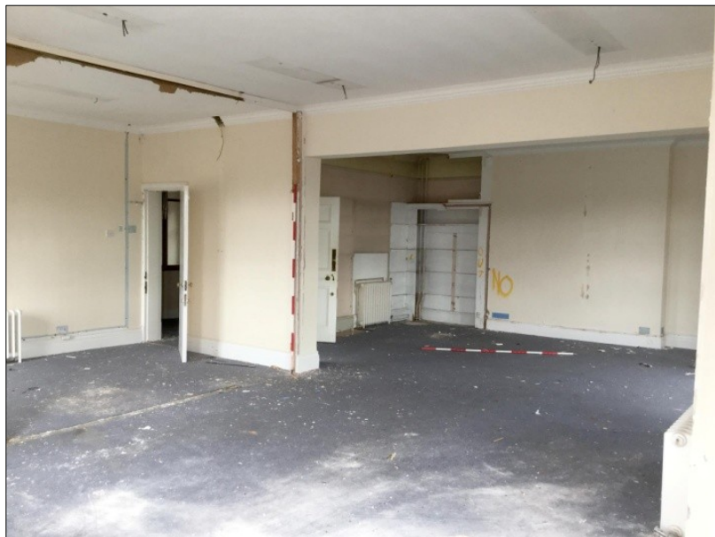
116. E-W Wing. Room 14. Facing NE
