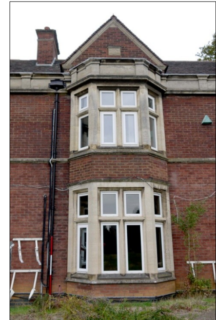
21. Two-storey bay window (E half of wing)
