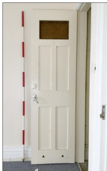
108. E-W Wing. Room 13. Vented door of airing cupboard
