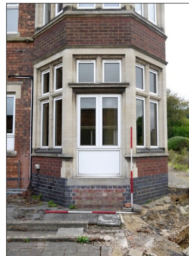
26. Former rear access from SW turret. Facing E
