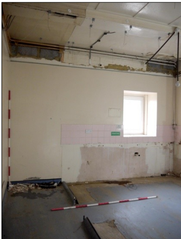
93. N-S Wing. Room 7. Kitchen. Facing E
