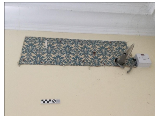
65. E-W Wing. Room 2. Residual C20 patterned wall paper
