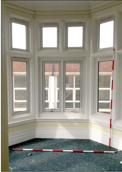
72. E-W Wing. Bay window in SE turret. Central panel denotes site of former rear door to garden. Facing SW
