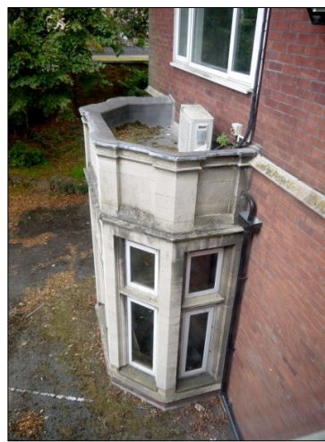
6. Front bay window parapet. Viewed from first floor, N-S wing
