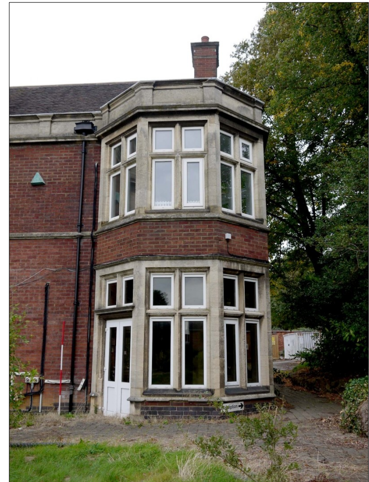
12. E-W wing, southern elevation. SE turret. Facing N
