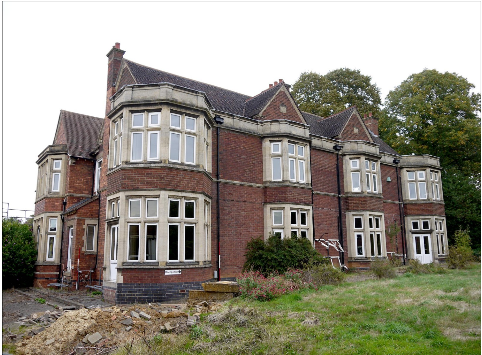
23. Overview of the rear of the building (E-W wing). Facing NE
