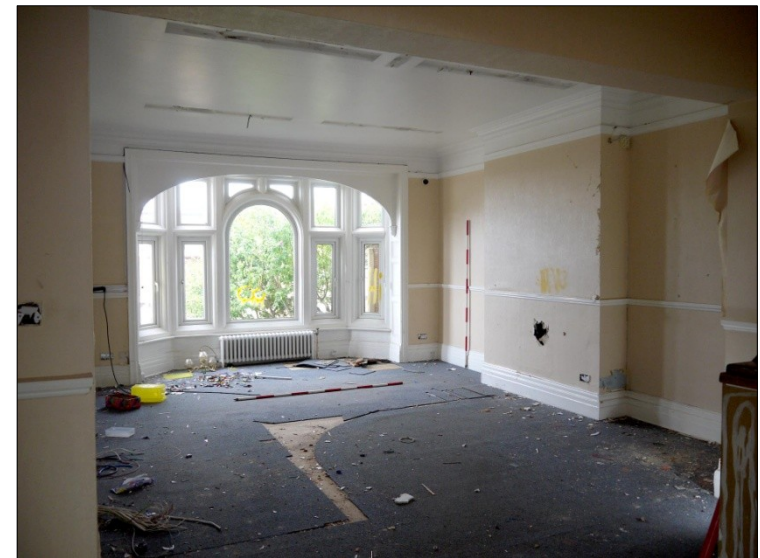
78. N-S Wing. Room 5; view from vestibule. Facing NW
