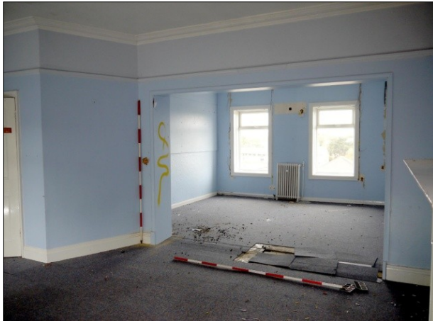
137. N-S Wing. Room 17E (bedroom). View towards Room 17W. Facing SW
