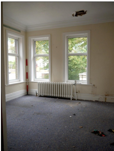
98. Room 11. Connecting room above lobby. Facing NE
