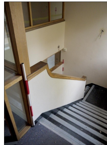
96. Stairway, upper flight. Facing NW
