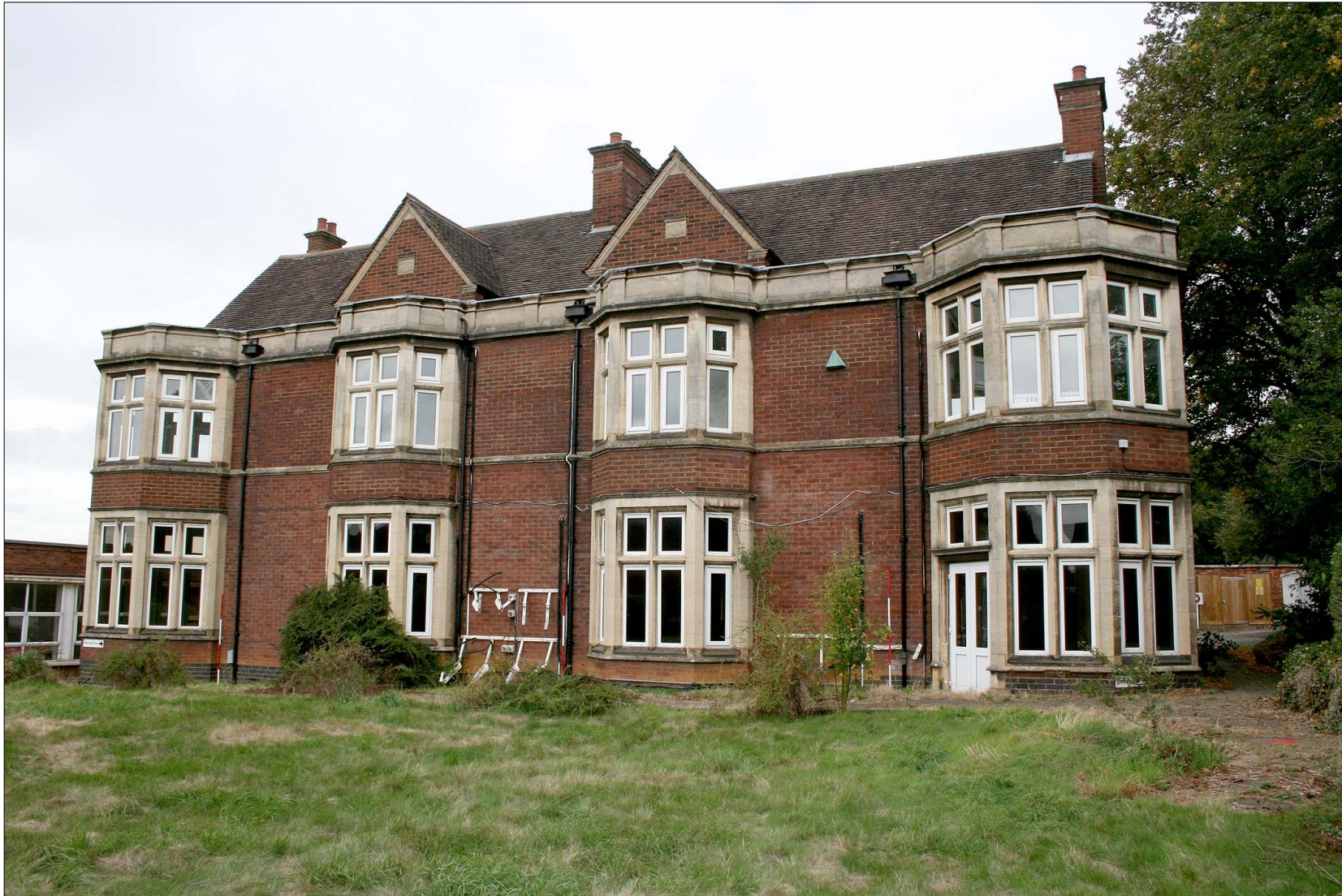
13. E-W wing. Overview of the rear (S) elevation. Facing NW
