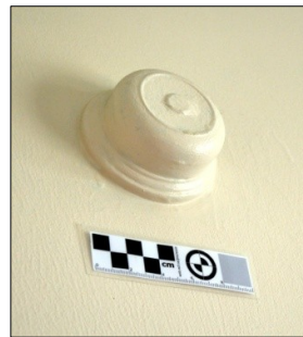
127. Room 16. Bakelite light fitting on chimney breast
