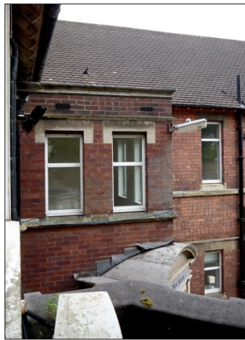
7. First floor landing. Viewed from E-W wing. Facing W
