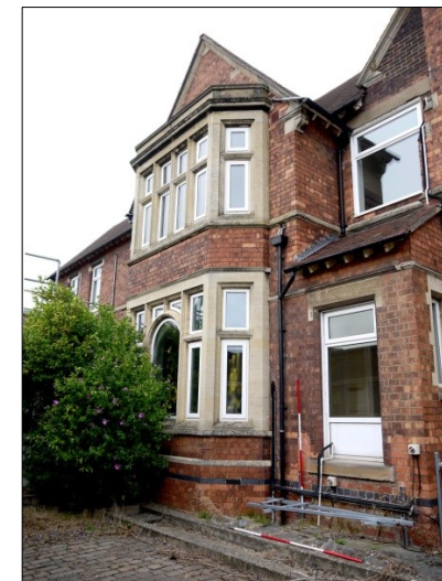
28. W elevation. Facing NE
