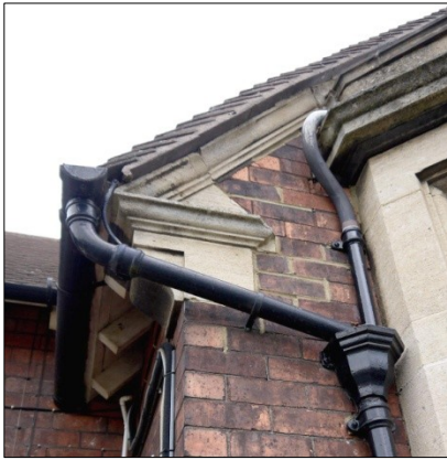
31. N-S wing. Eave return (late 19 th century building)
