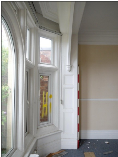
80. Left . lower part of moulded pelmet. Facing N
