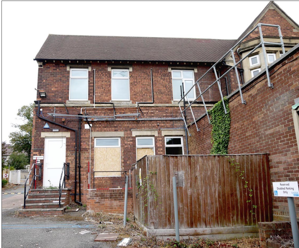
37. Rear aspect of the west elevation (northern end). Facing E
