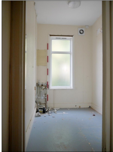
122. N-S Wing. Room 19. Probable former bathroom). Facing E
