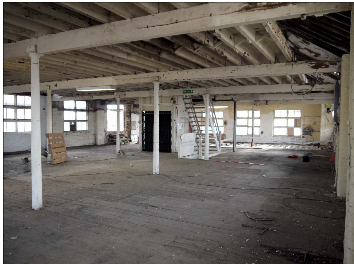
48. Second Floor. Overview. Facing SSE
