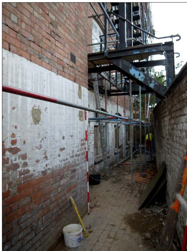
12. NW End, overview. (Fire escape attached to boundary wall). Facing SW
