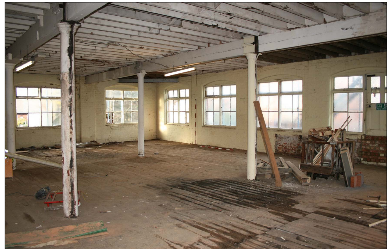
36. First Floor. Overview of NW end. Facing NW
