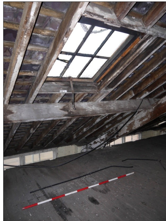
66. Third Floor. Typical casement roof light. Facing NW
