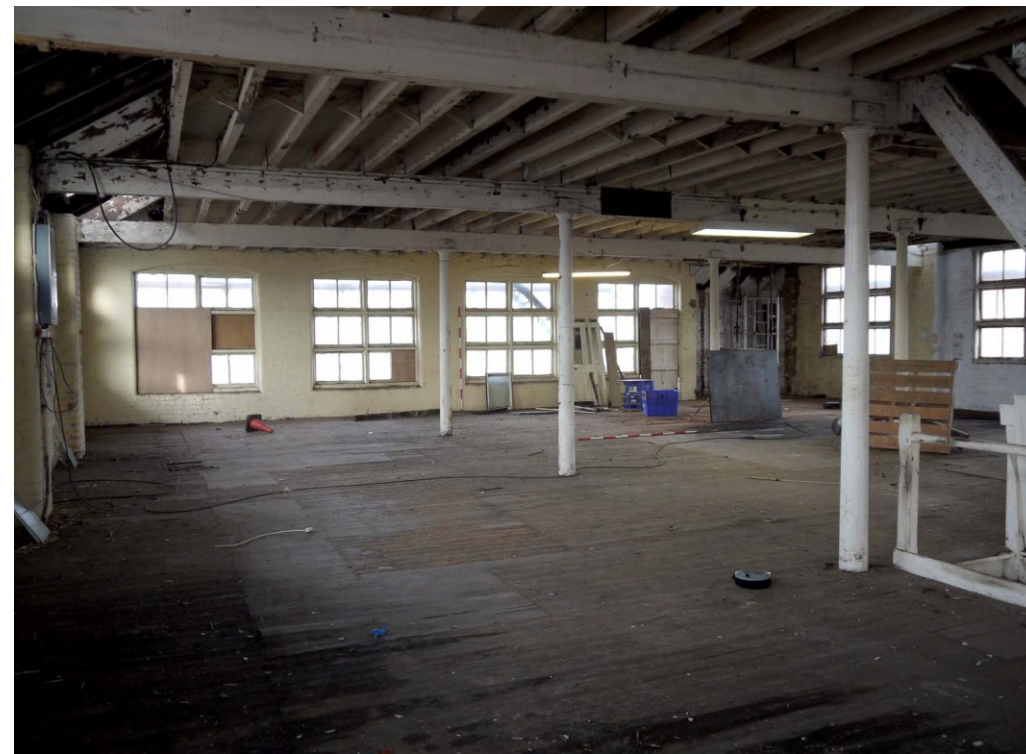
46. Second Floor. Overview of NW end. Stair to R. Facing NNE
