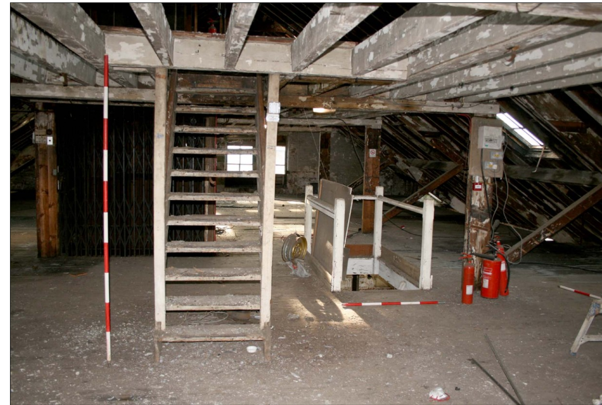
57. Third Floor. Landing area. Facing SE
