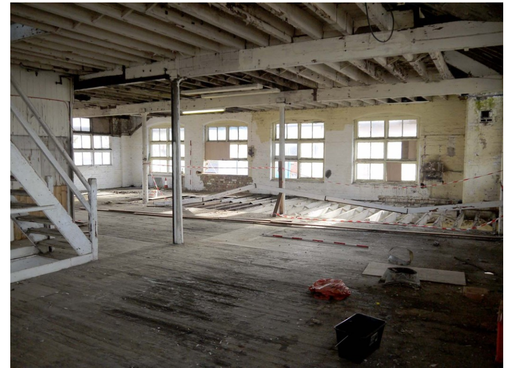
47. Second Floor. Overview of SE end. Stair to L. Facing SE
