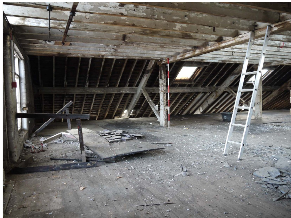
58. Third Floor. Overview of NW end. Roof truss. Facing SE
