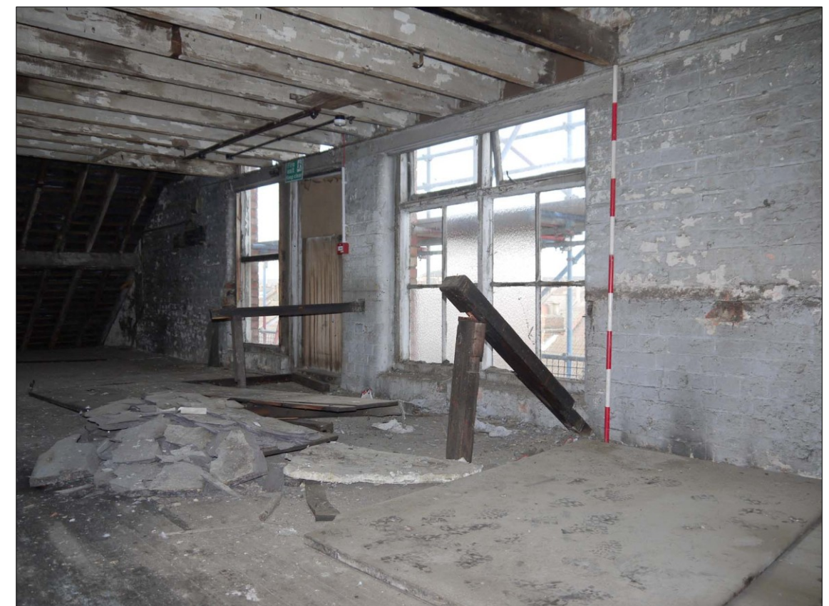
63. Third Floor. Overview of NW end. Fire exit. Facing NW
