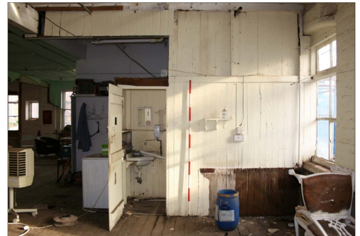
30. First Floor. W.C. Facing ENE
