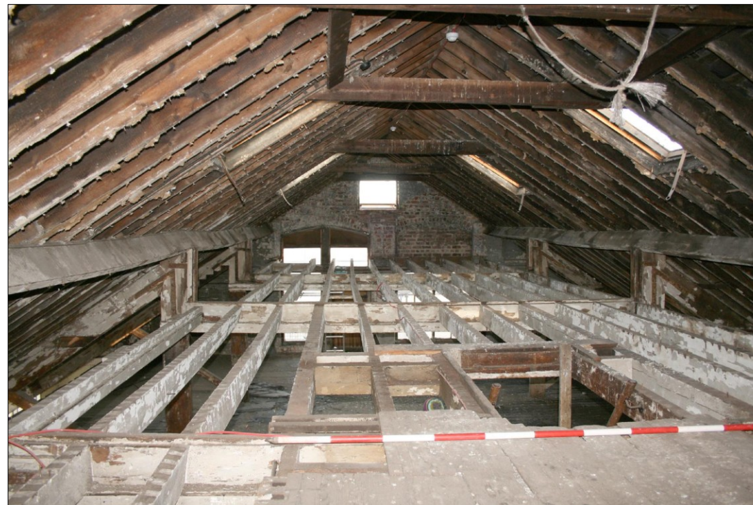
67. Fourth Floor and roof frame (floor boards removed). Facing NNW
