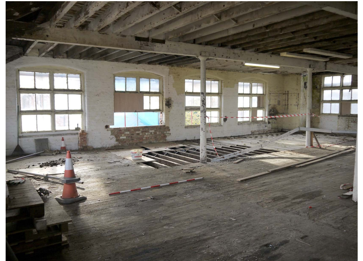
51. Second Floor. Overview of SE end. Facing SW
