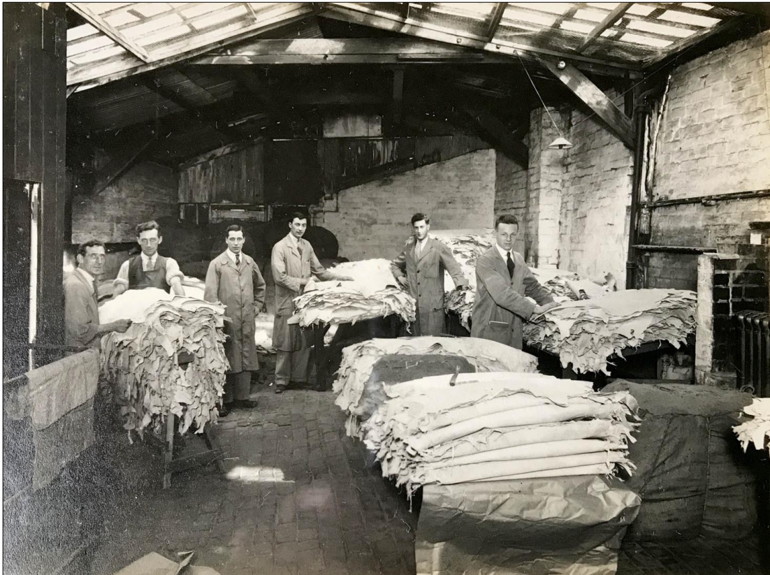
Figure 15. Dickens Brothers Leather Works, 1929: baling finished sides for despatch (? front annexe)
