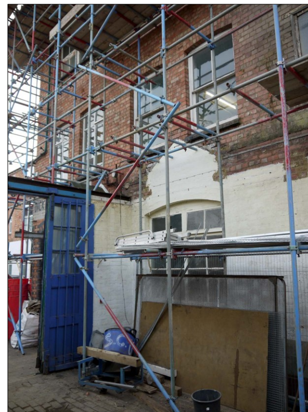
6. Front elevation. Facing SW
