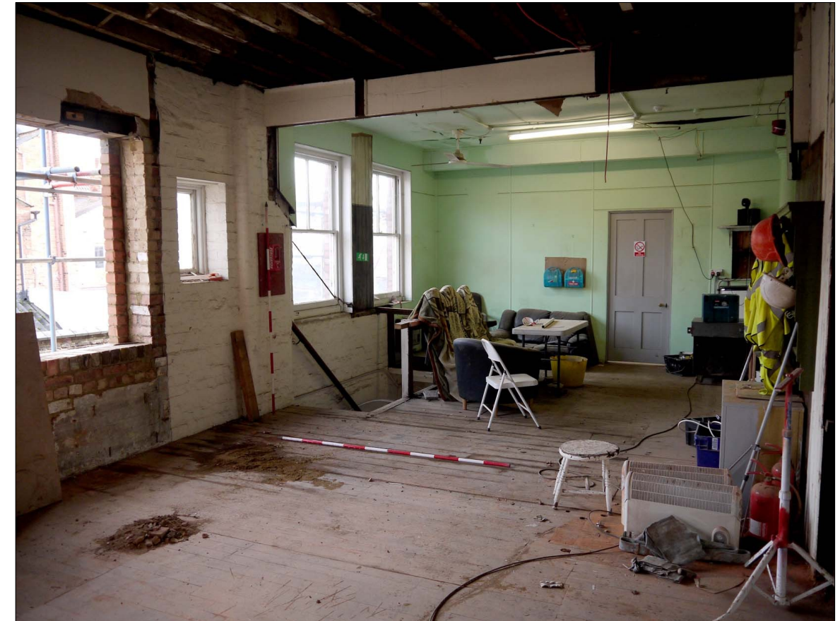
40. First Floor. View towards former office area and stair. Facing SE
