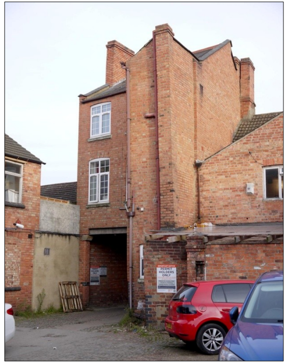
70. The rear of the entrance to Kettering Place from Kettering Road. Facing NE
