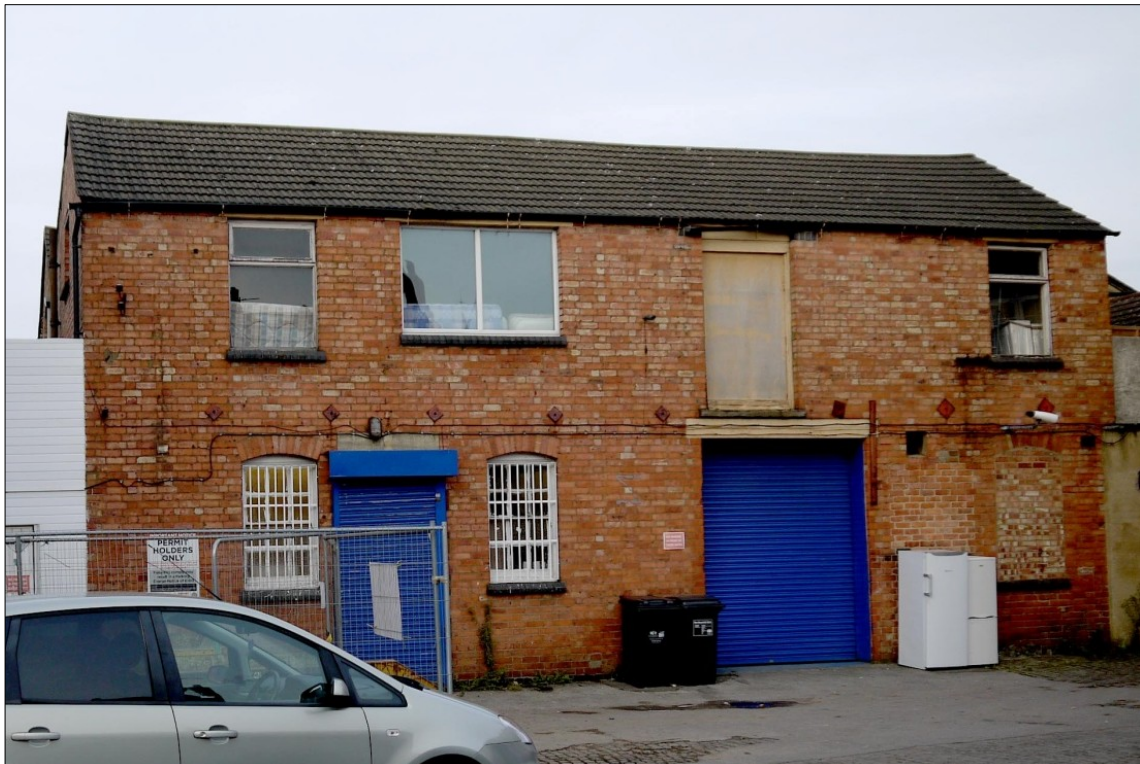
71. Former warehouse/ later works canteen. Facing N
