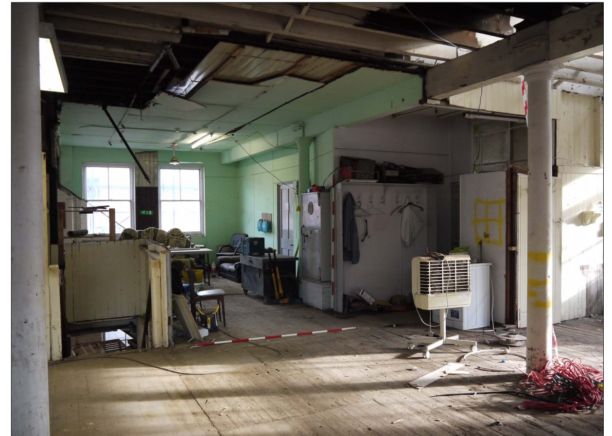
29. First Floor. View towards office area. Stairs to L. Facing E
