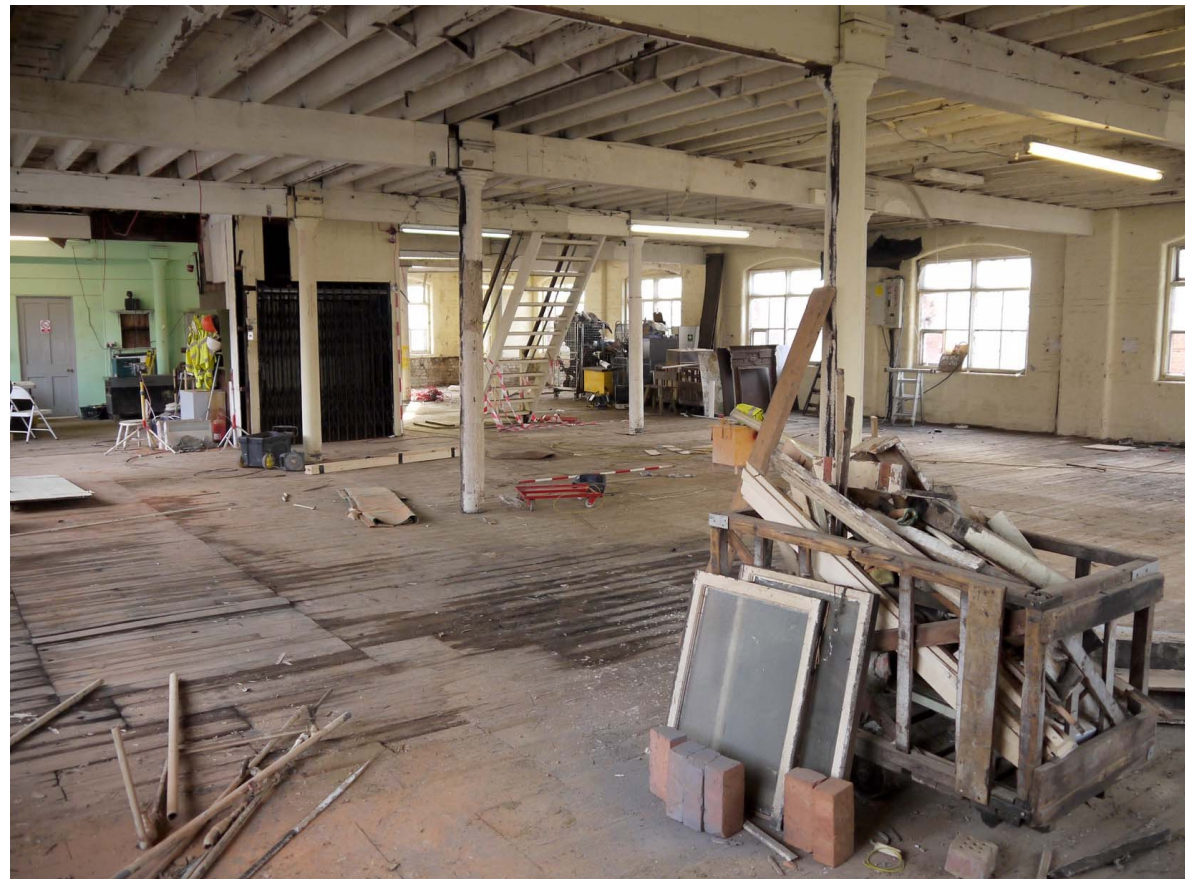
37. First Floor. Overview. Facing SW
