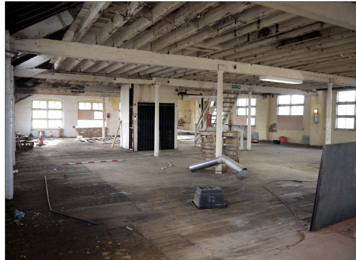
49. Second Floor. Overview. Facing SSW
