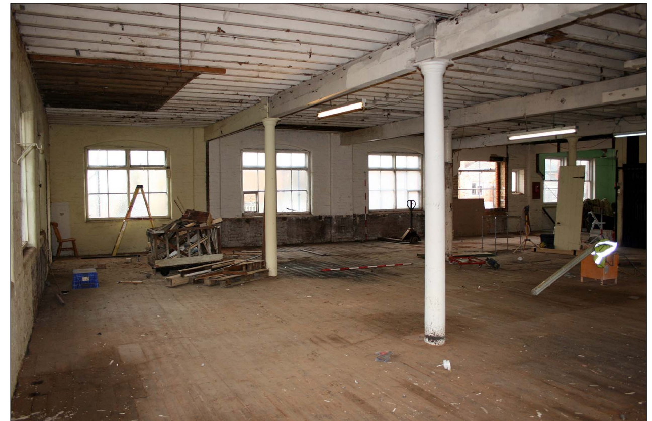
35. First Floor. Overview of NW end. Facing NE
