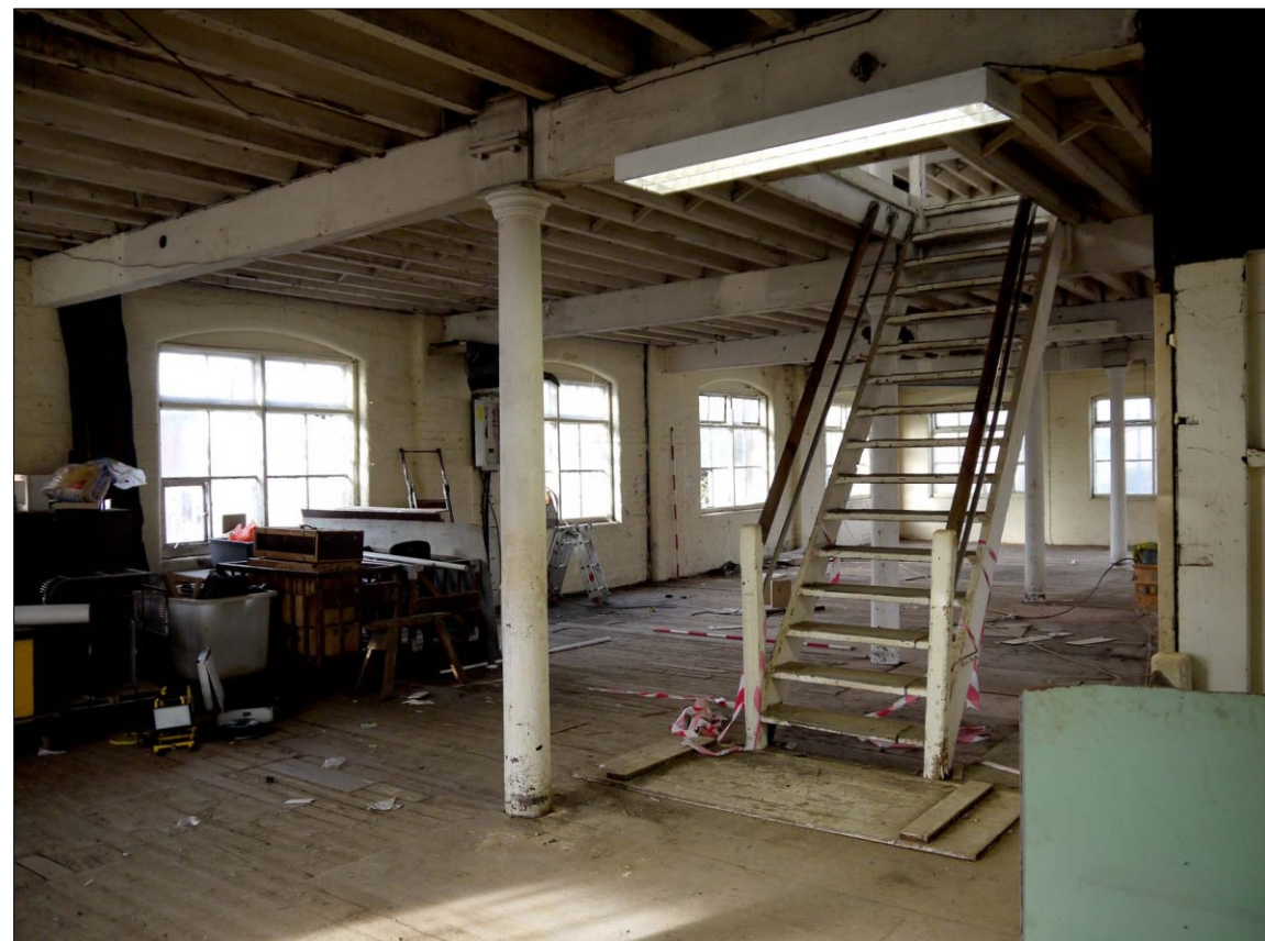
34. First Floor. Stair to Second Floor. Facing NW
