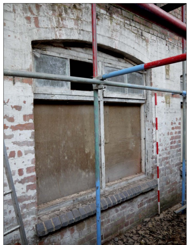
13. NW End. Typical ground floor window. Facing WSW
