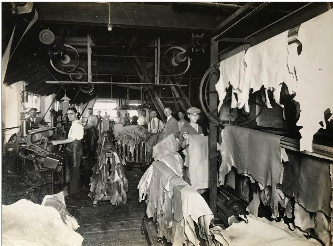
Figure 12. Dickens Brothers Leather Works, 1929: boarding processes (2 nd or 3 rd floor)
