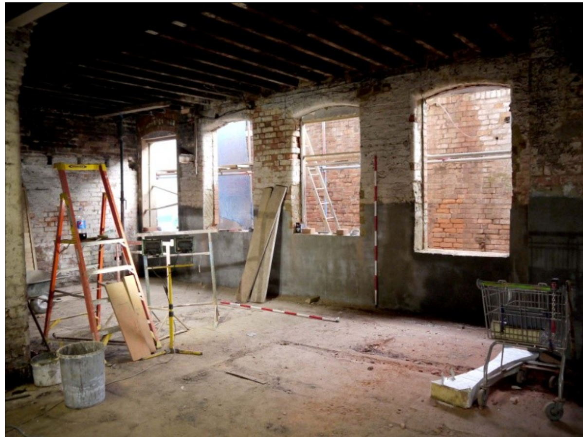
27. Ground Floor. SE End, workshop windows. Facing SE
