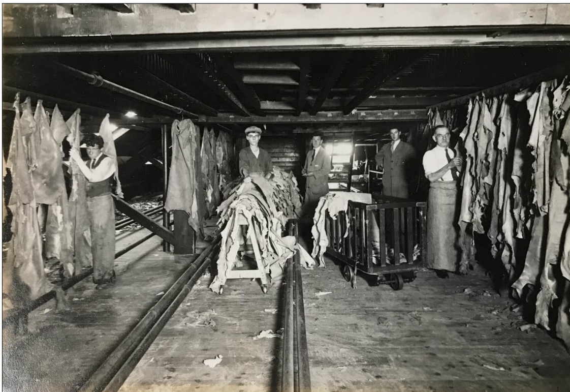
Figure 10. Dickens Brothers Leather Works, 1929: hanging sides to dry (3 rd floor)
