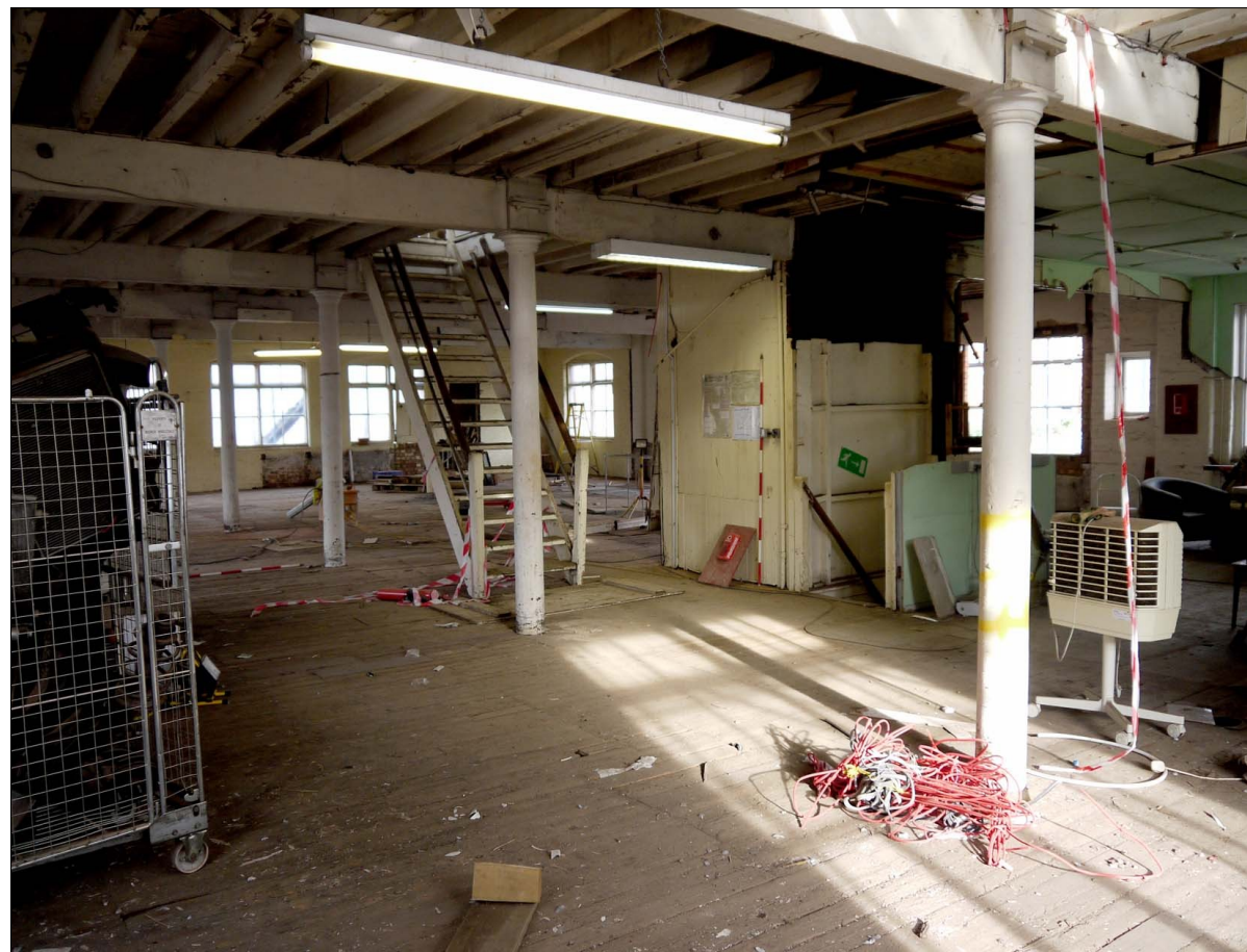
28. First Floor overview. Facing NNE
