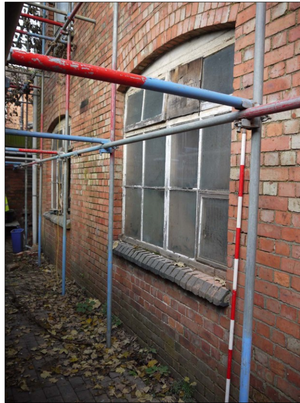
16. Rear elevation. Typical ground floor window. Facing N
