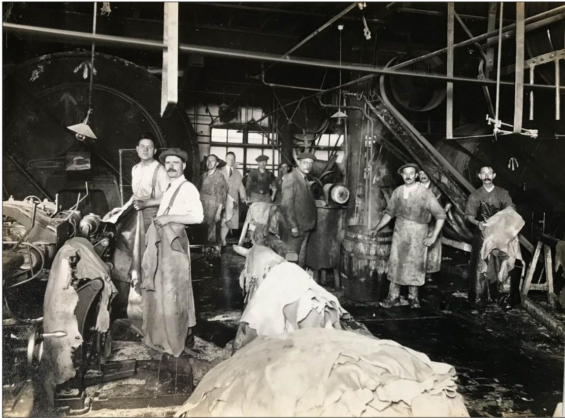
Figure 9. Dickens Brothers Leather Works, 1929: shaving and tumbling sides (ground floor)
