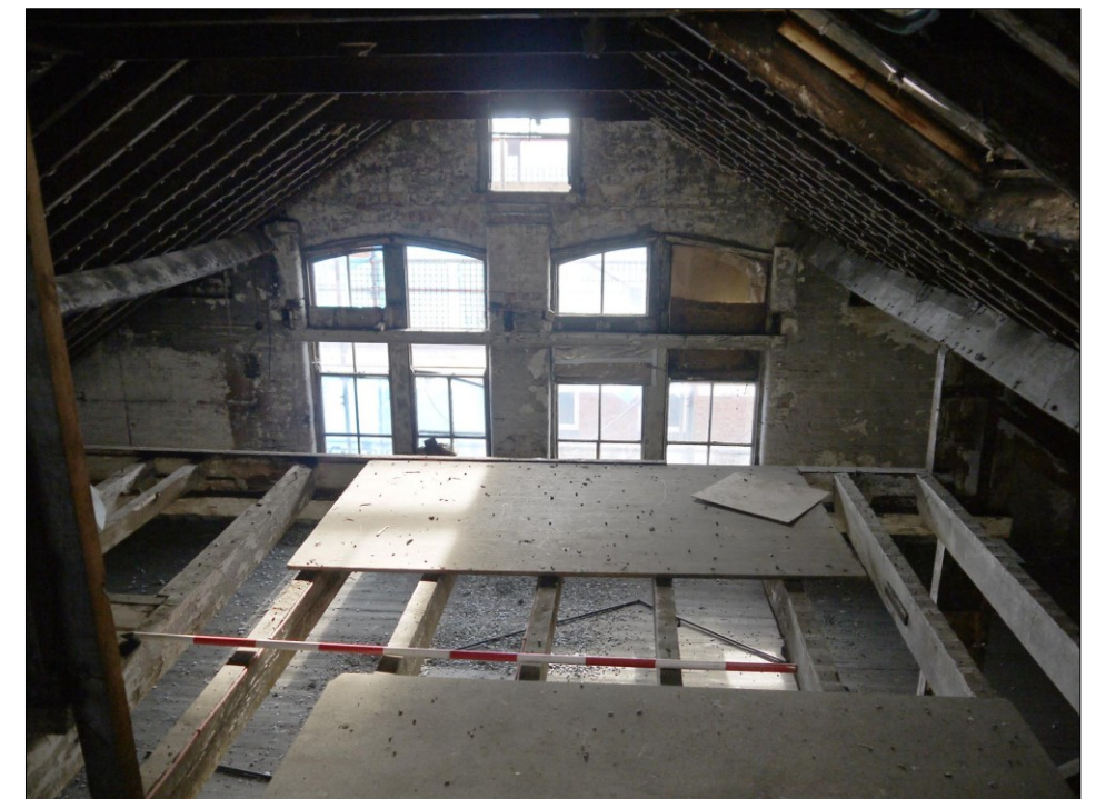
68. Fourth Floor and roof frame (floor boards removed). Facing SSE
