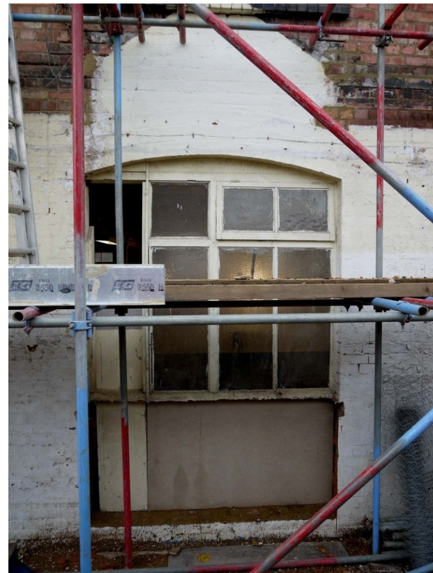
9. Front elevation. Typical ground floor window. Facing WSW
