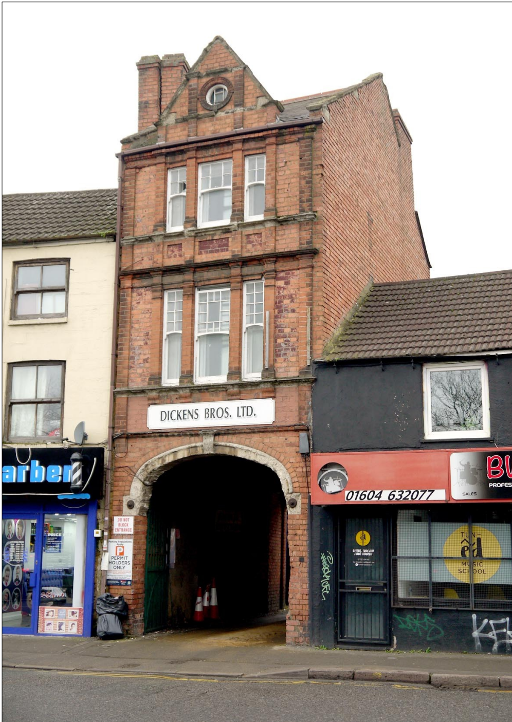
72. Entrance to Kettering Place from Kettering Road. Facing SW
