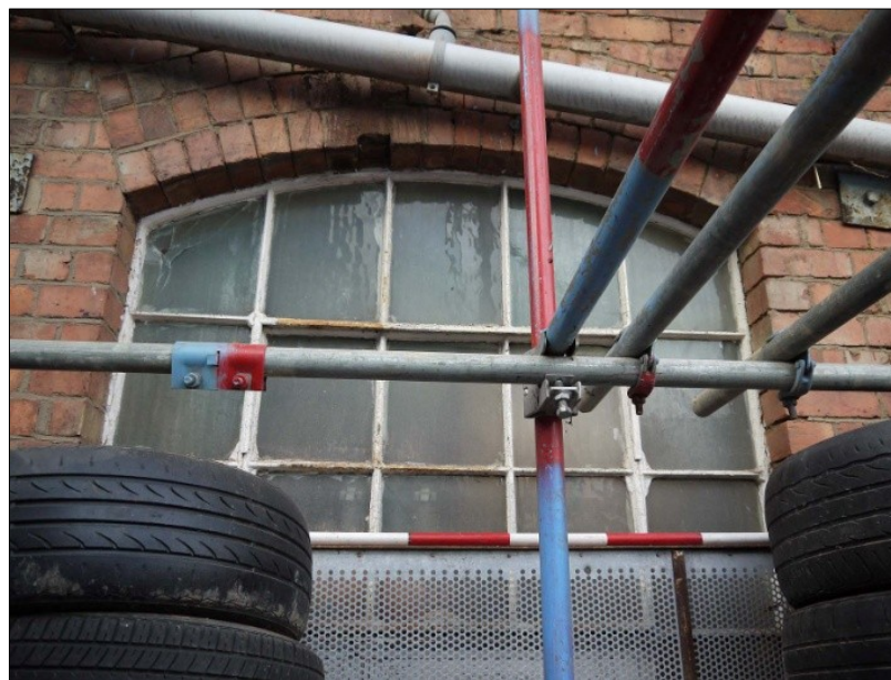
20. SE End. Metal-framed window. Facing NNW
