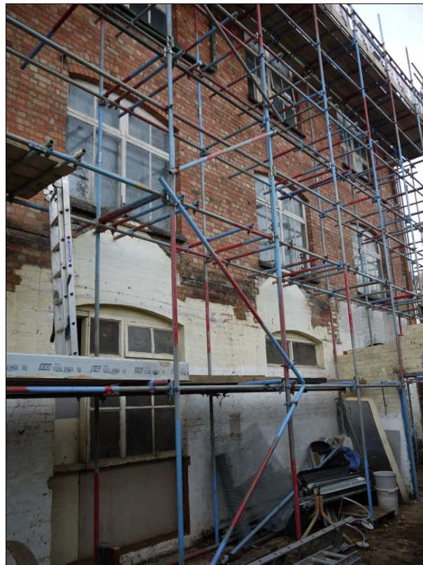
8. Front elevation. Facing NW
