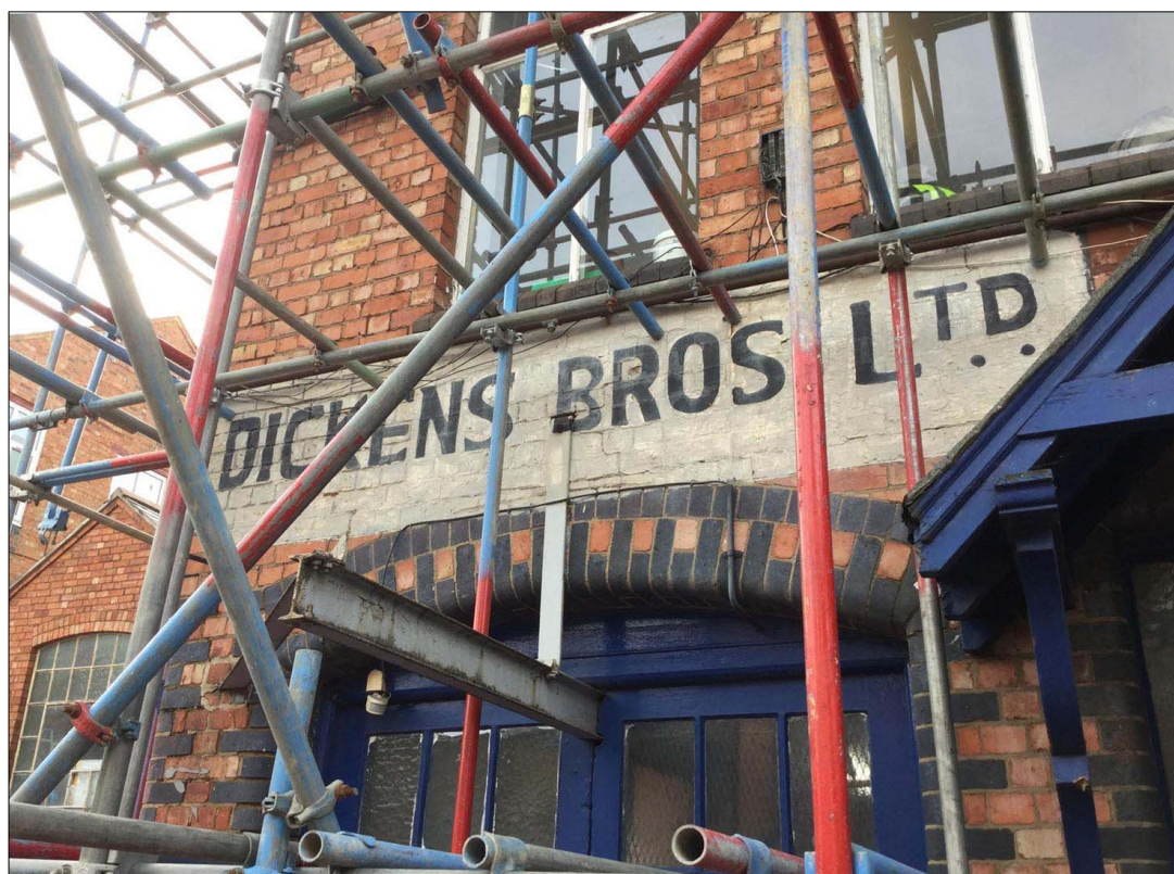
2. Hand-painted signage above the factory and main/finished goods door. Facing SW
