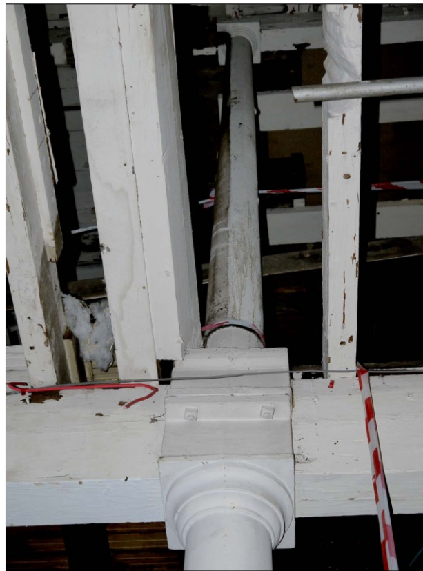
45. First Floor. Column junction between First Floor & Second Floor, Facing NNW
