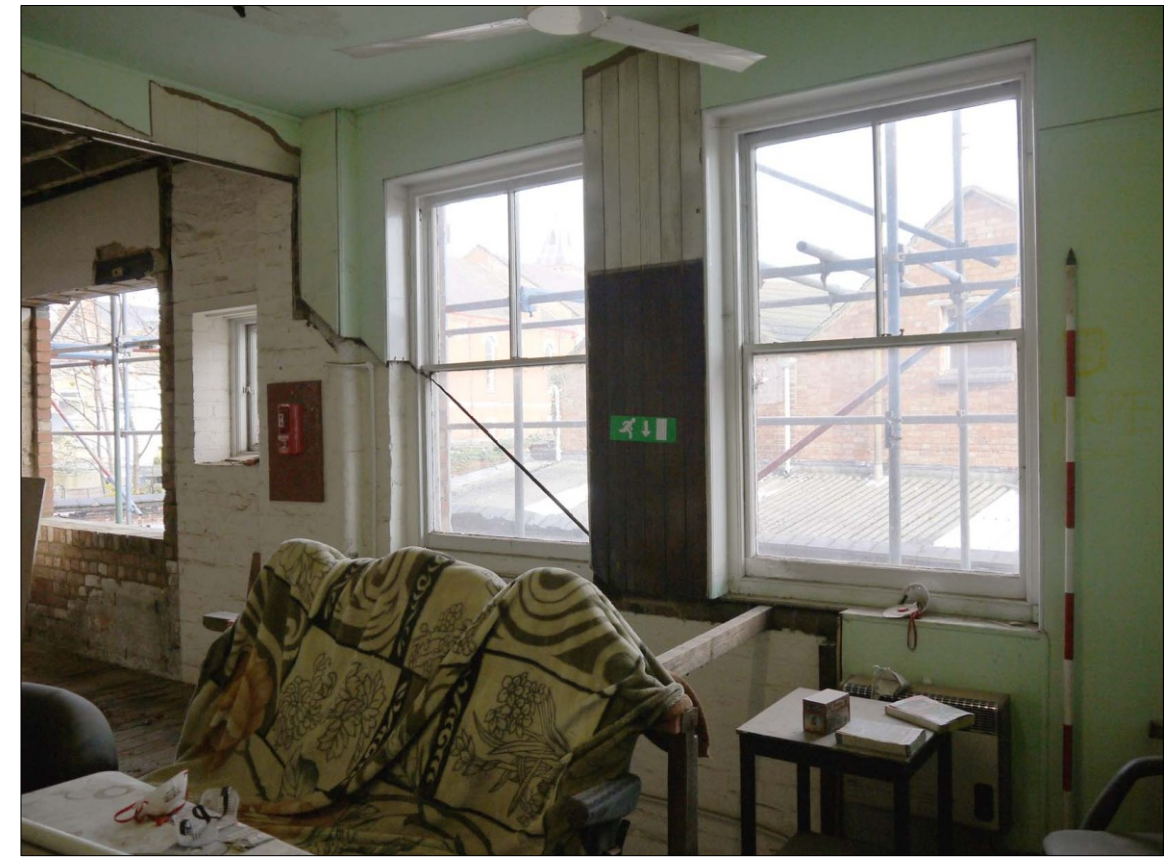
42. First Floor. Former office area. Facing NE
