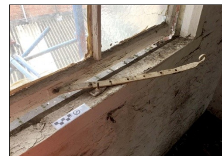
55. Second Floor. Typical wrought iron window stay (late C19). Facing SSE
