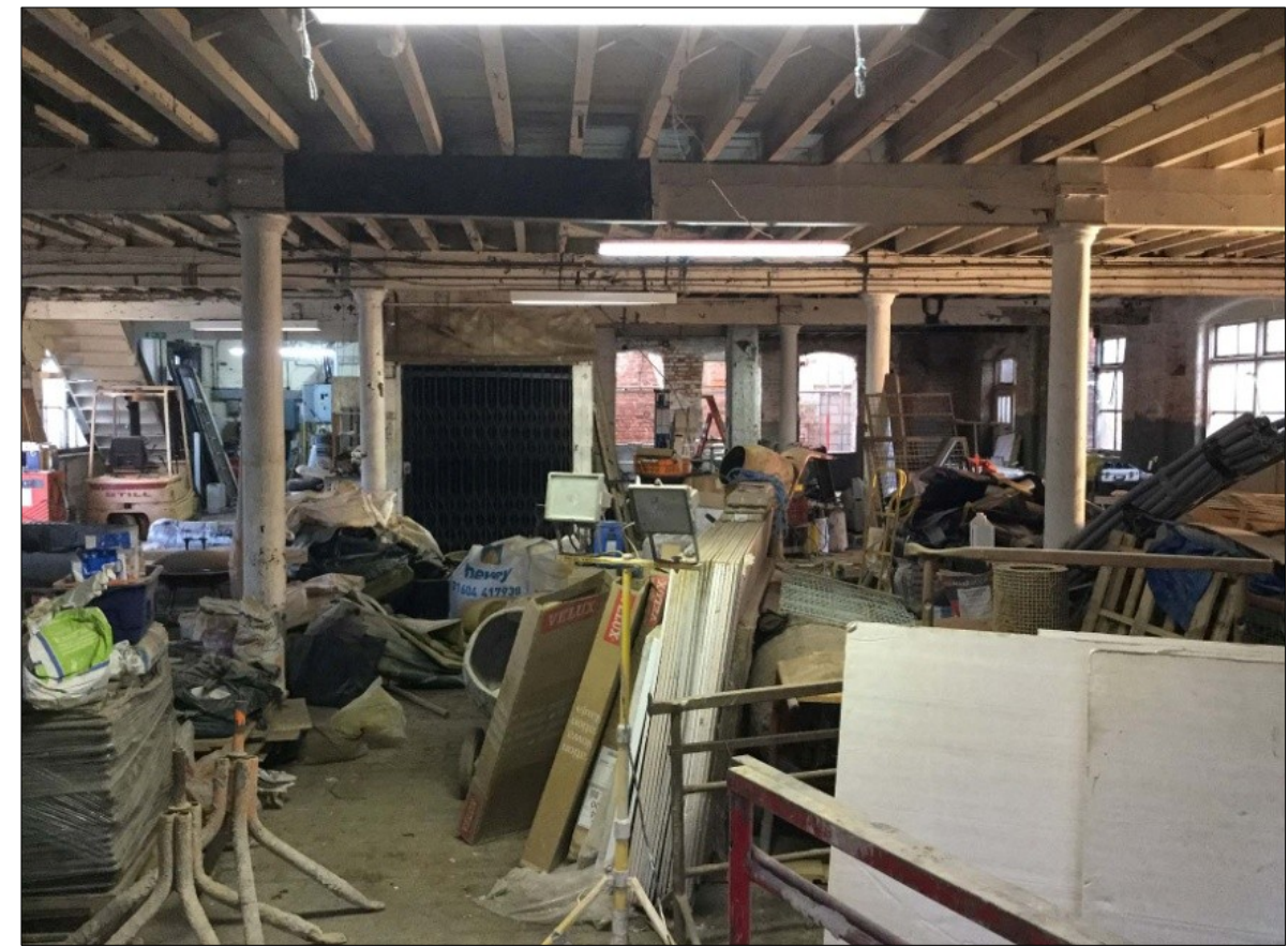
24. Ground Floor, overview. Facing SSE
