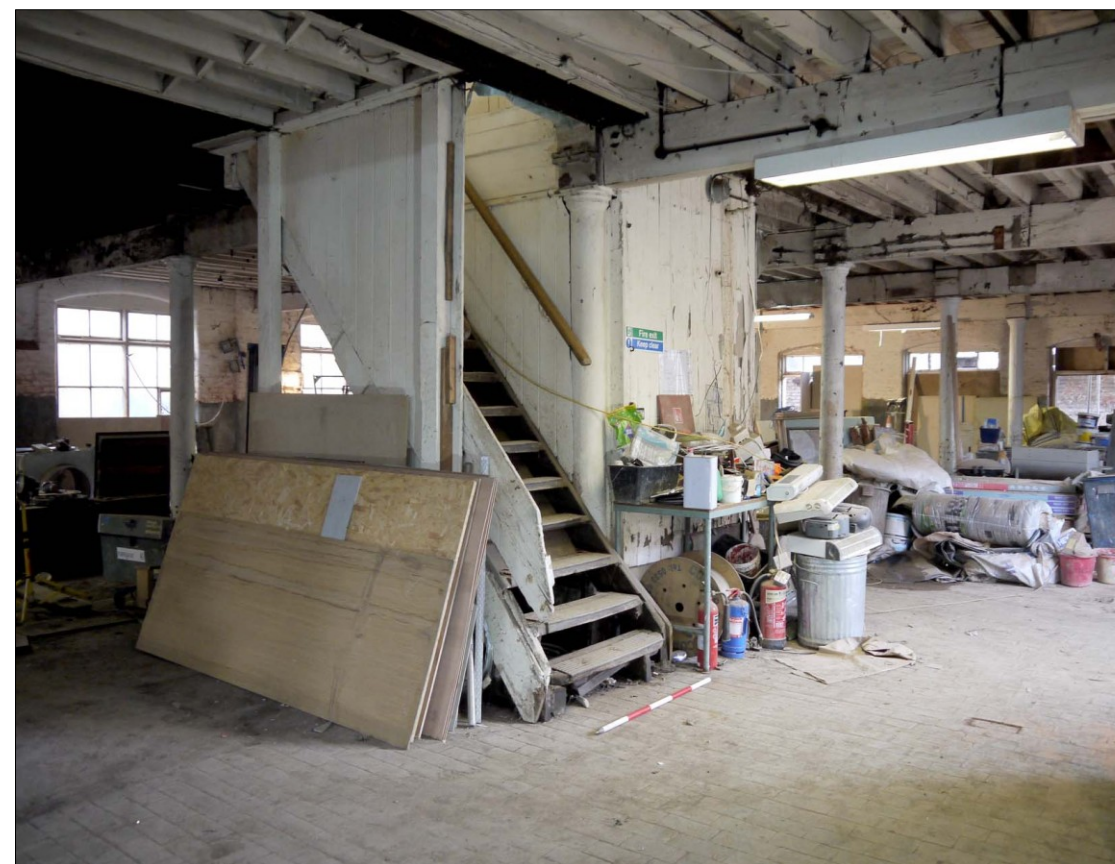
21. Ground Floor. Main access to floors. Lift shaft behind. Facing NW
