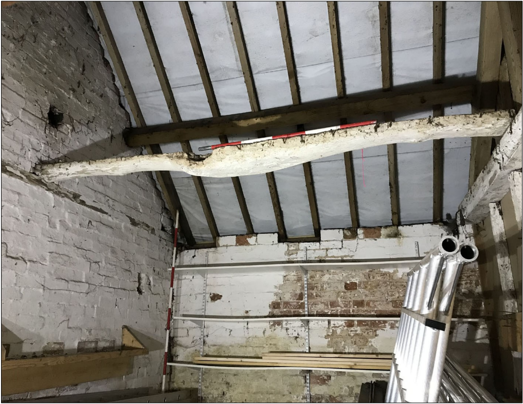
59. Loosebox at the SE end of Building 5, showing a re-claimed cambered oak tie beam used as a longitudinal /spine beam. Facing SW
