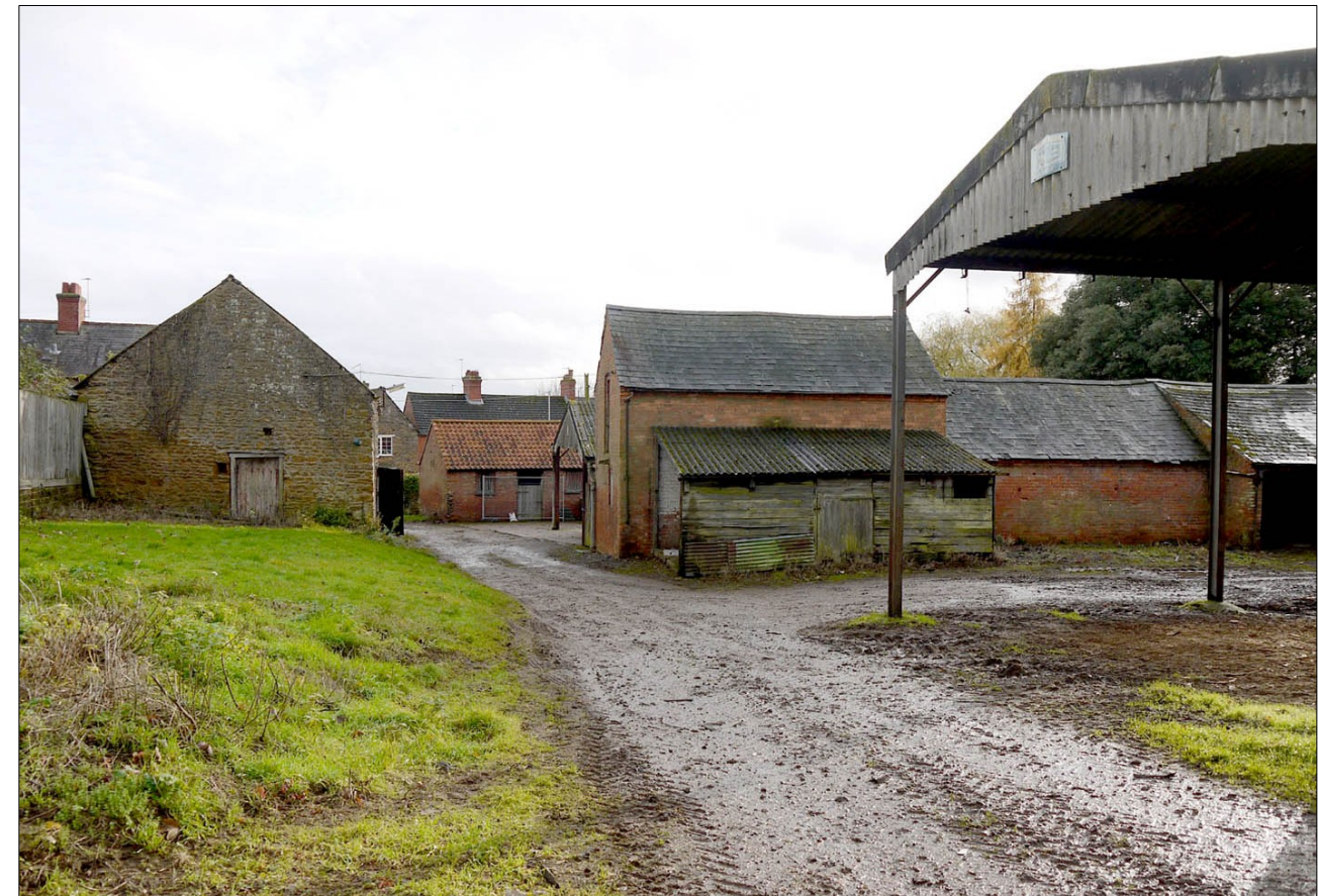
11 . Overview of the farm buildings from the NW
