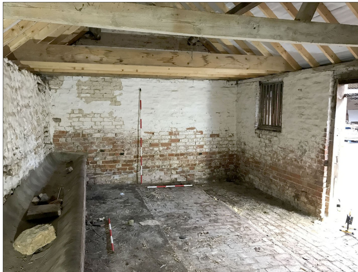
63. Interior of Building 6 (cow house). Manger to L Facing SW
