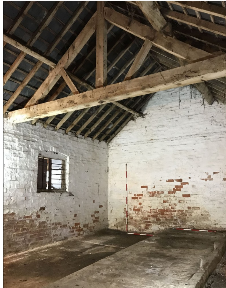
46. Interior of the Building 3, cow house/milking parlour. Facing SW
