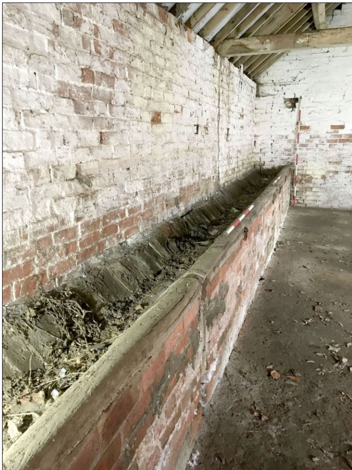
57. Brick-built manger in Building 5 (open-fronted cow shelter), facing NW
