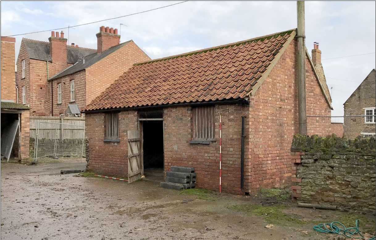
31. Building 6, cow house. Facing SE
