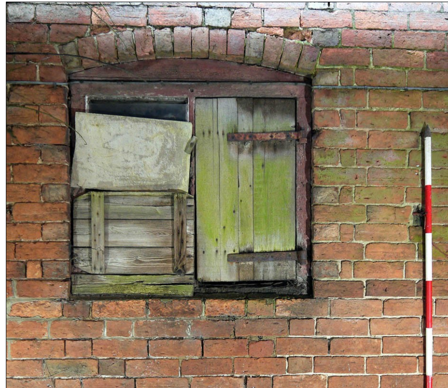
24. Building 2 (cow house/milking parlour), shuttered window. Facing NW
