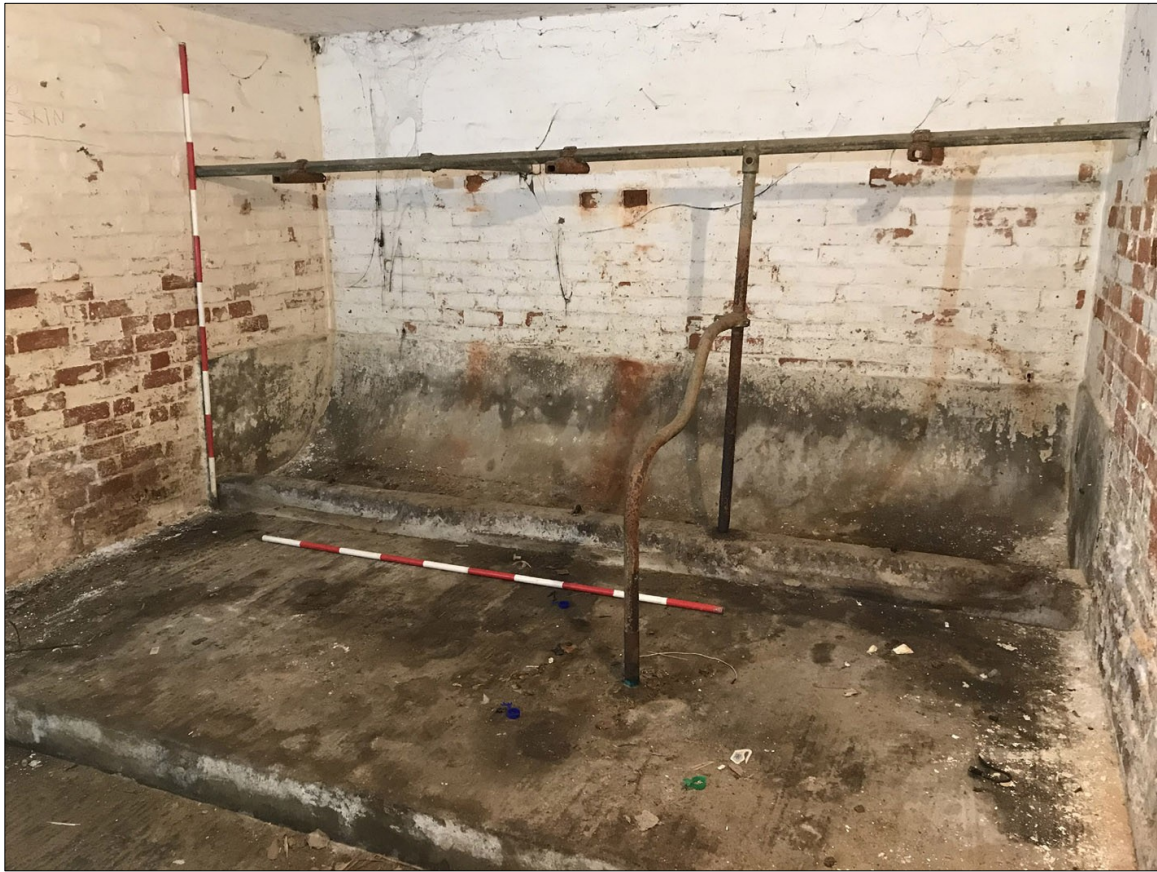
44. Building 2, SW box (milking parlour), cow stalls and trough manger. Facing NW
