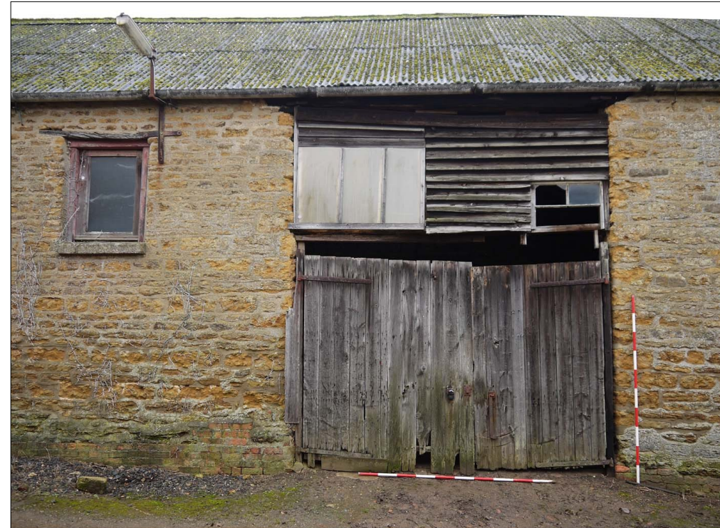
8. Building 1 (the stone barn), wagon entrance. Facing NE
