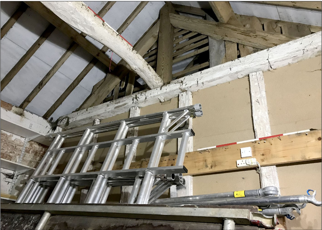
60. Loosebox at the SE end of Building 5, showing the partition wall constructed of re-claimed oak timbers. Facing NW
