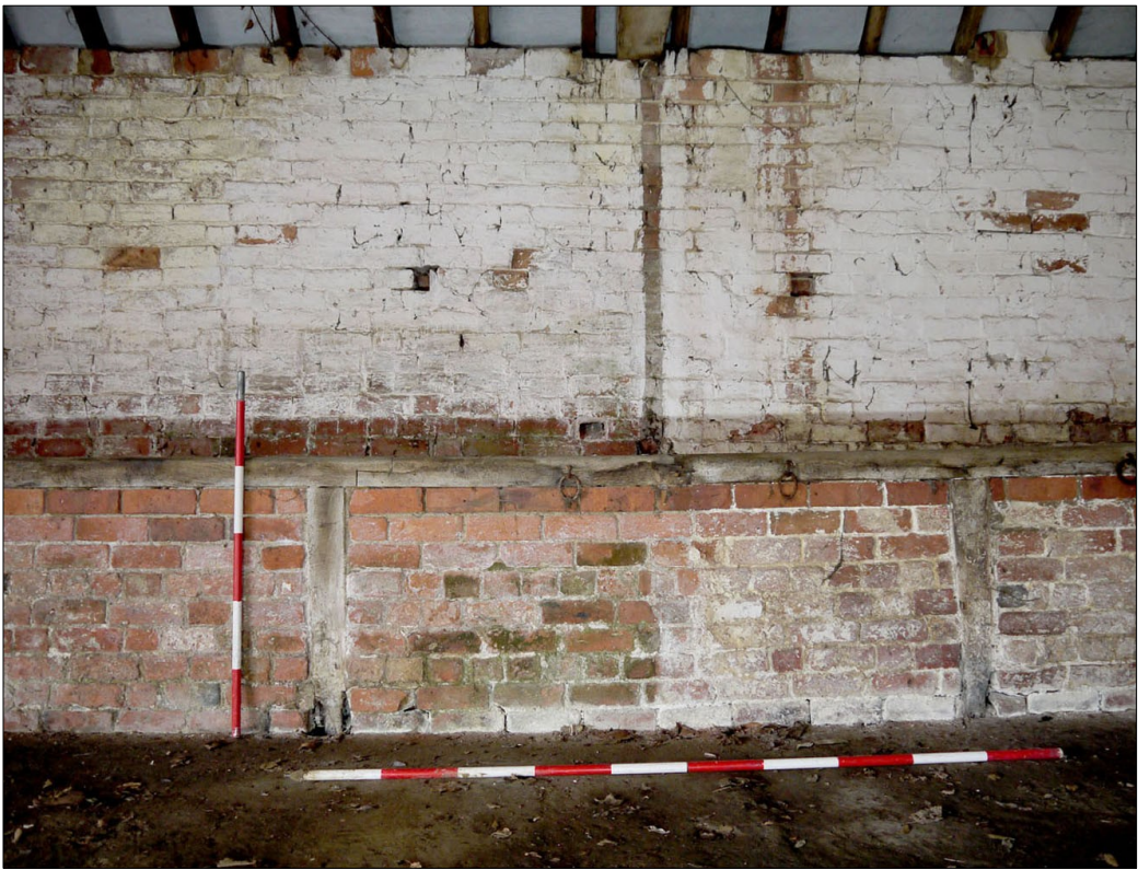
58. Brick-built manger in Building 5 (open-fronted cow shelter), facing SW
