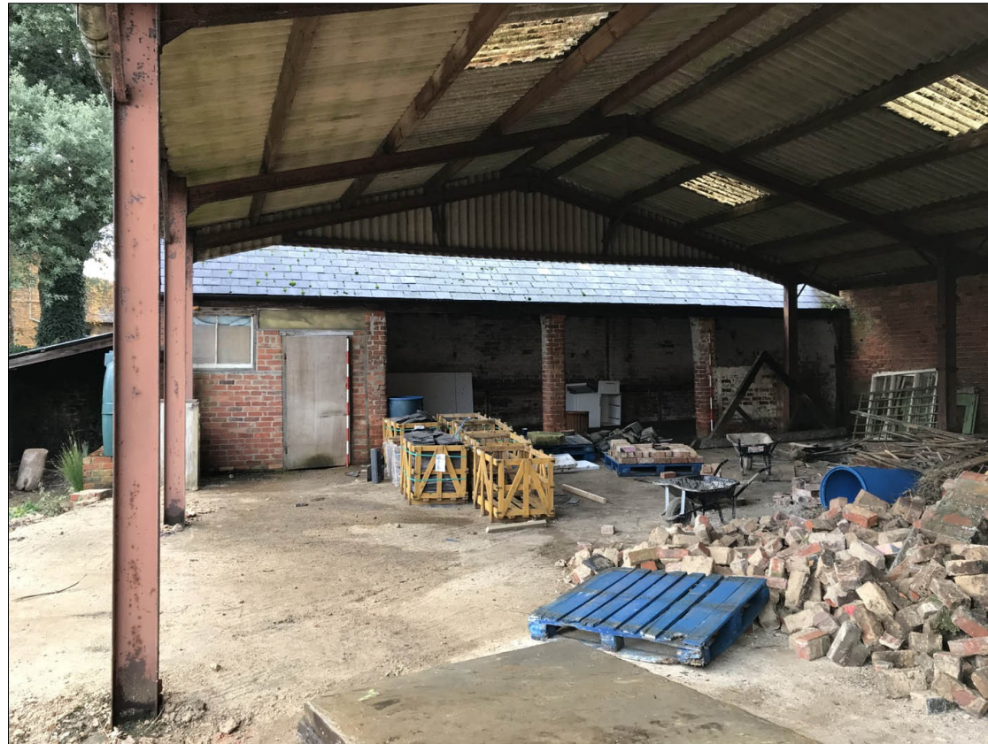
26. Building 5 (open-fronted cow house), view from the yard. Facing SW
