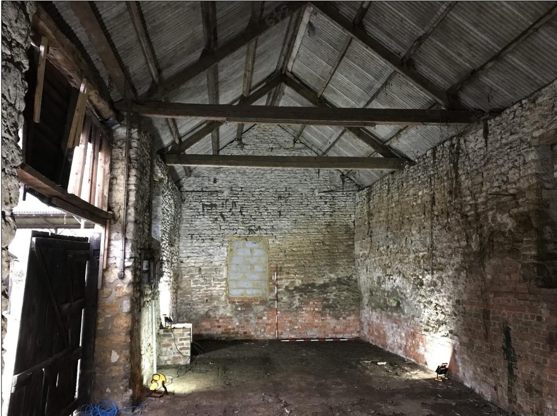
32. Interior of the Building 1, the Stone Barn. Facing NNW
