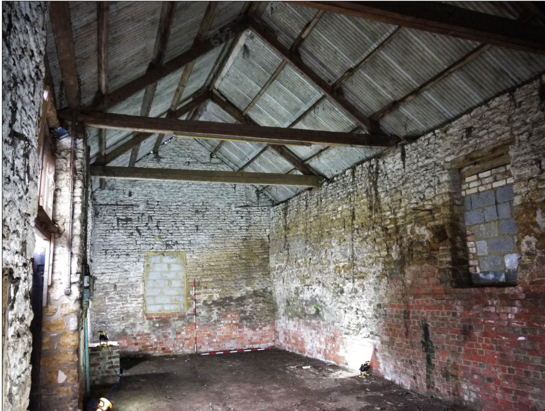
33. Interior of the Building 1, the stone barn. Facing NNW
