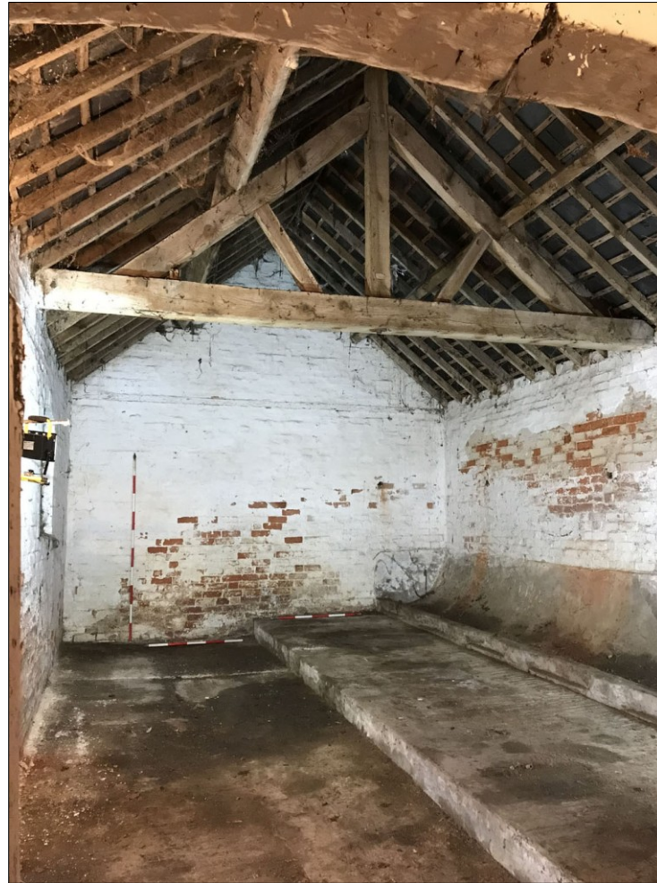
45. Interior of the Building 3, cow house/milking parlour. Trough
