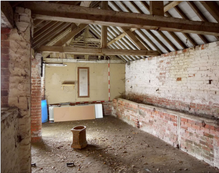
56. Interior of Building 5 (open-fronted cow shelter), facing S. Manger to R
