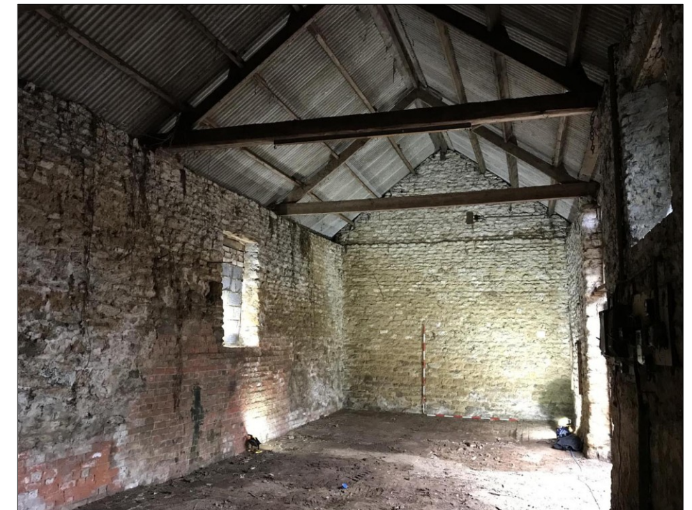
37. Interior of the Building 1, the stone barn. Facing SE
