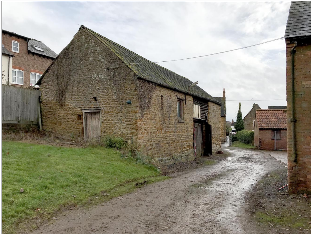
7. Building 1 (the stone barn). Facing SE
