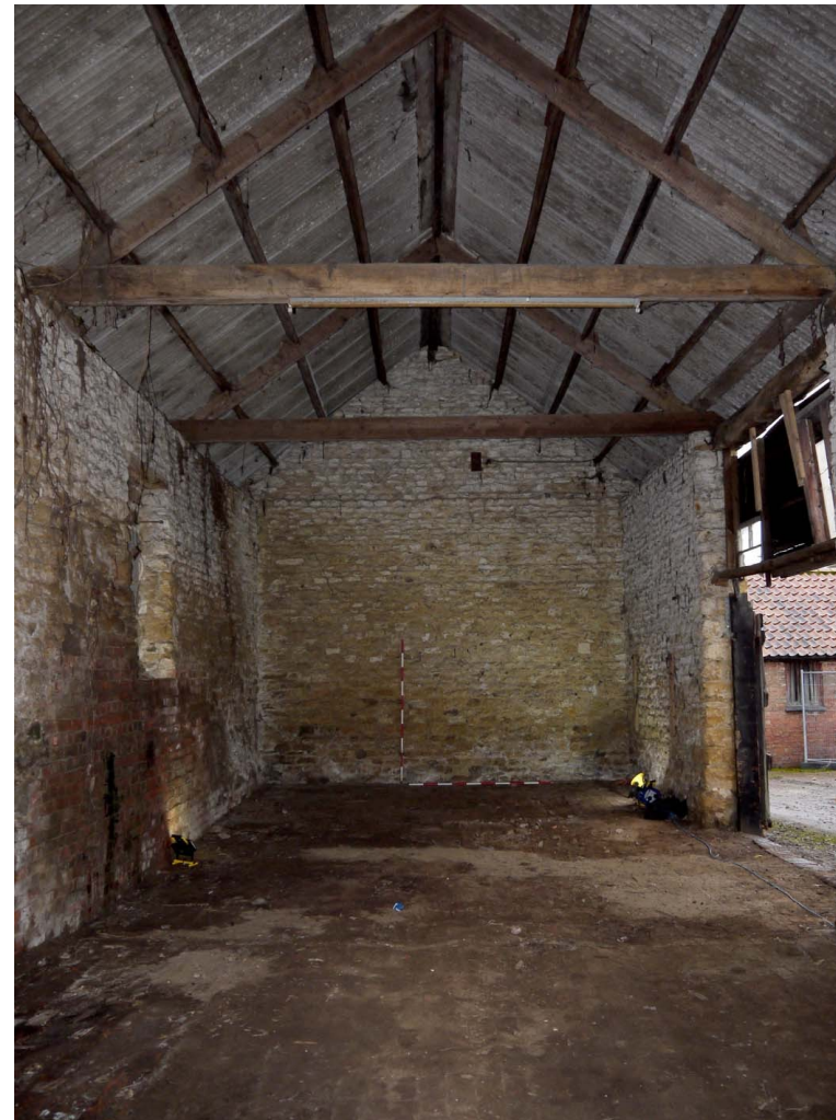
36. Interior of the Building 1, the stone barn. Facing SE
