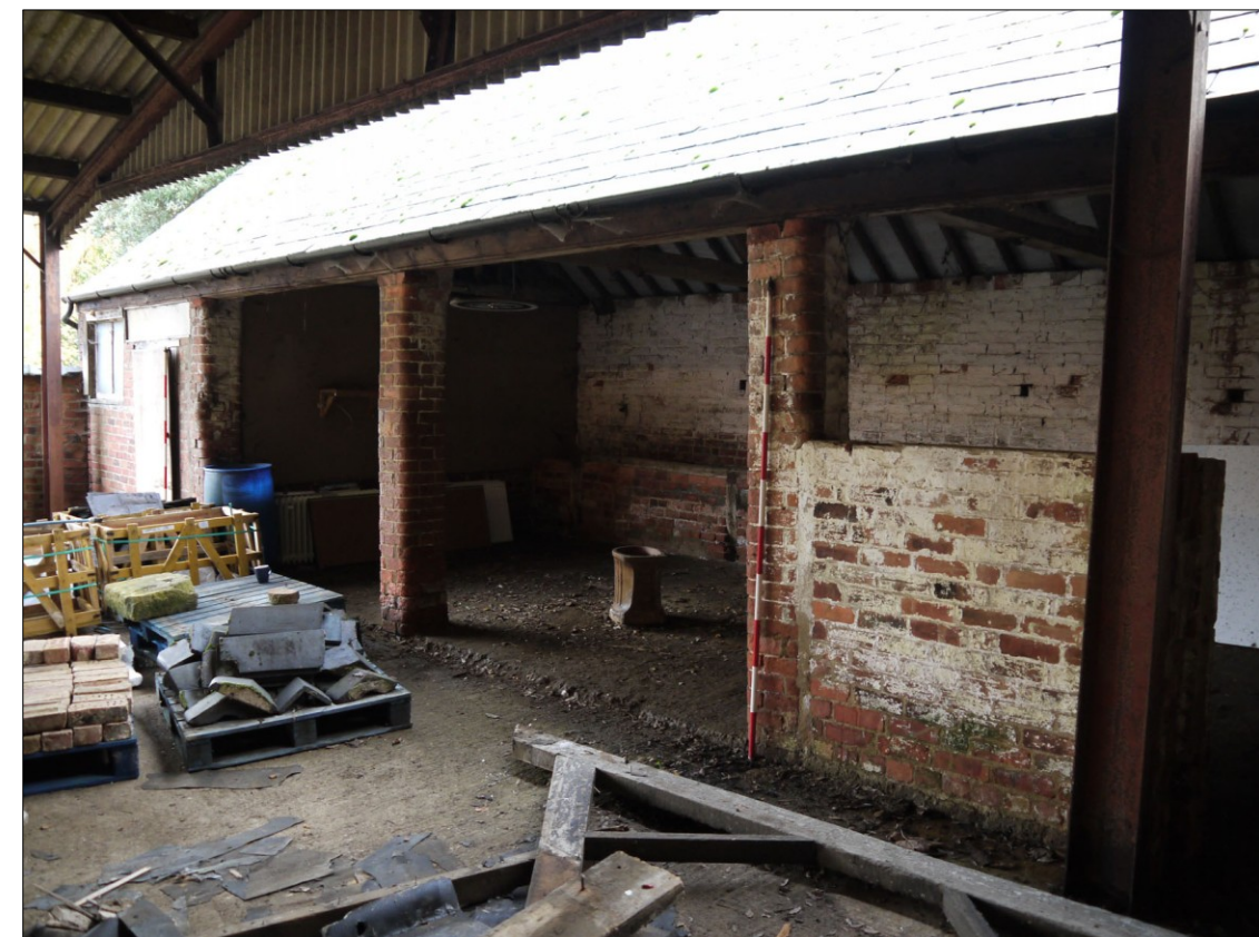
29. Building 5 (open-fronted cow house). Facing SSW
