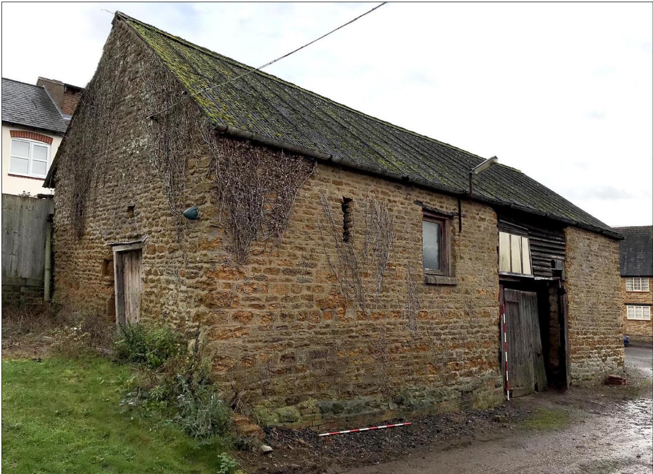
6. Building 1 (the stone barn). Facing SE
