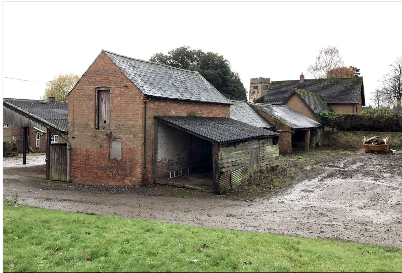
12. View of the Buildings 2 to 4, facing SW. Looking beyond to The Vicarage and Earls Barton Church. Mercer's Farm farmhouse to extreme L
