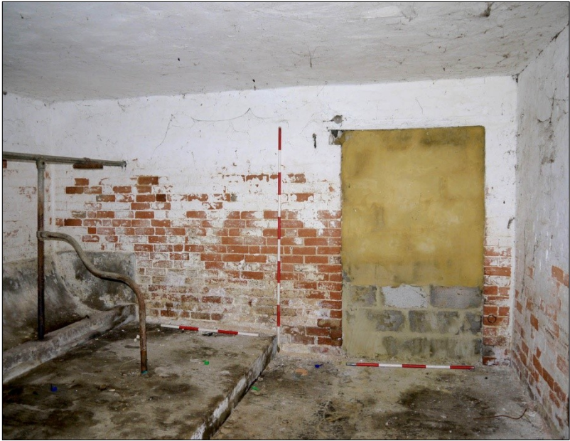
41 Interior of the SW box (milking parlour) of Building 2. Manger (L) and blocked doorway (R) to the the NE box. Facing NE
