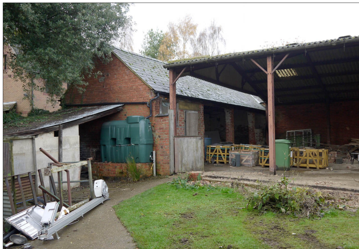
28. Building 5 (open-fronted cow house). Facing NW
