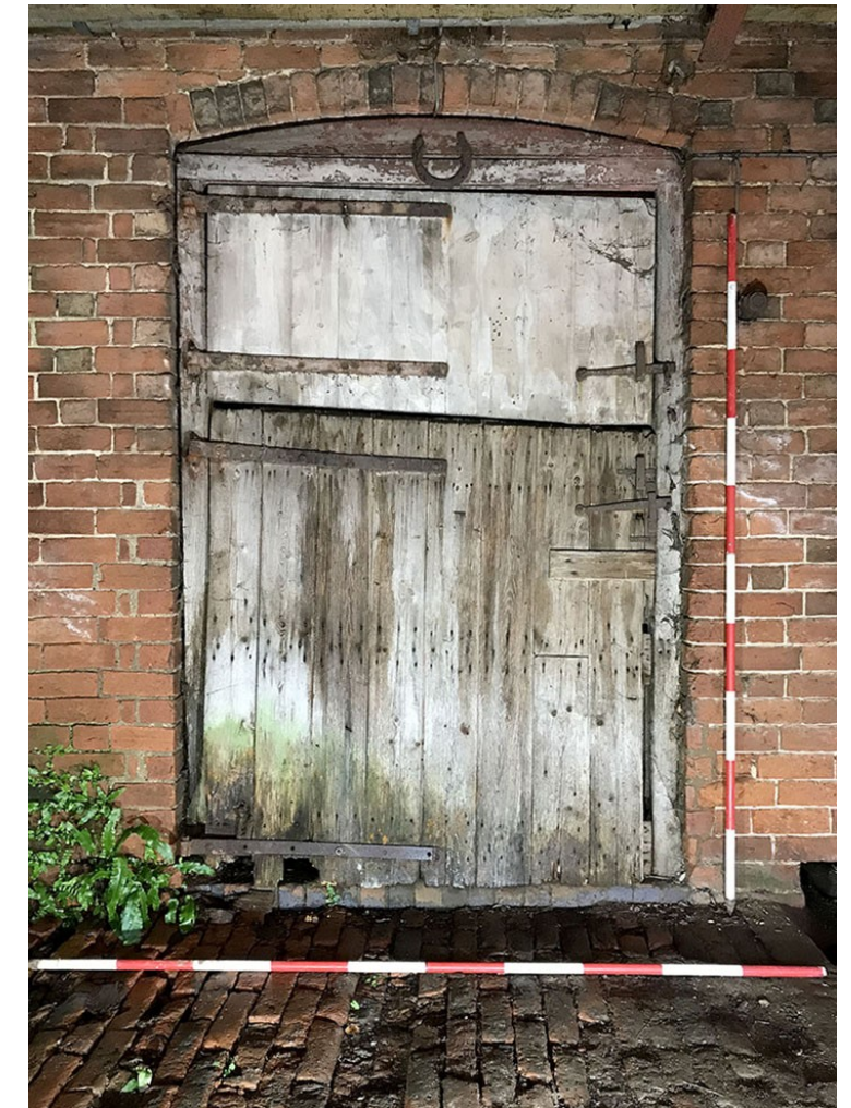
25. Building 3 (loosebox), entrance with stable-type door. Facing NW
