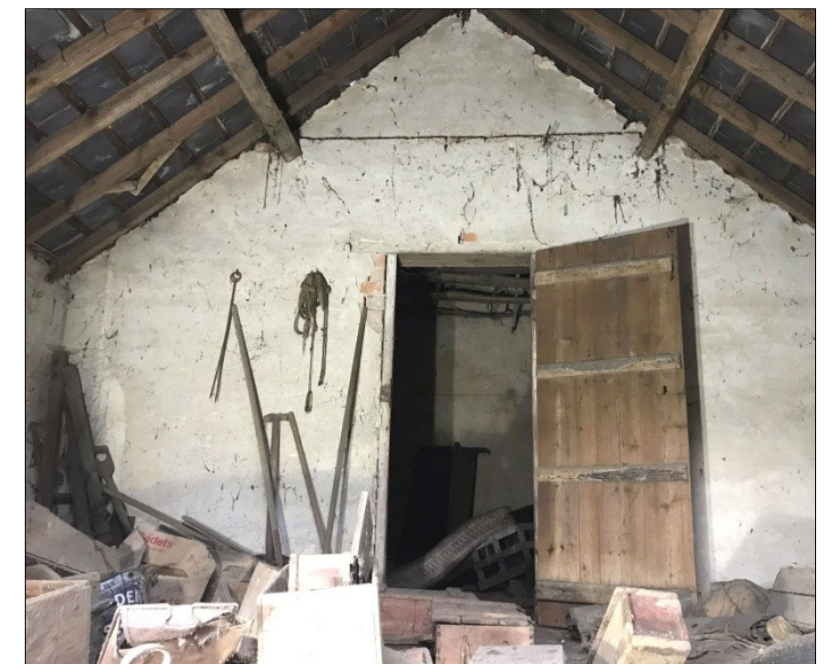
50. Interior of the hayloft above Building 2. Facing SW
