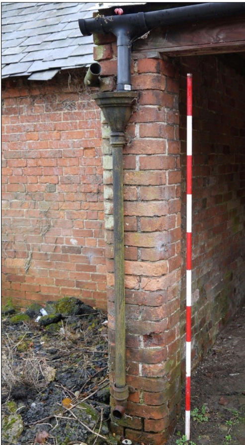
17. Cast-iron down-pipe and hopper (Building 4)
