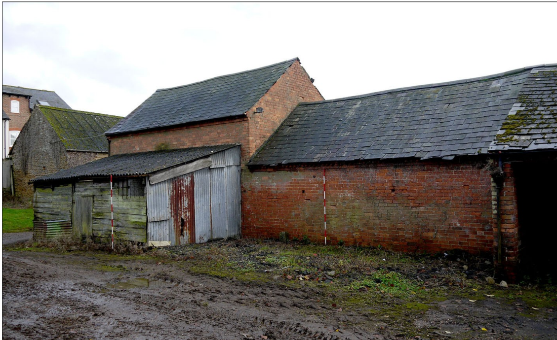
16. The rear of brick-built cow-houses, Buildings 2 and 3. Facing ESE
