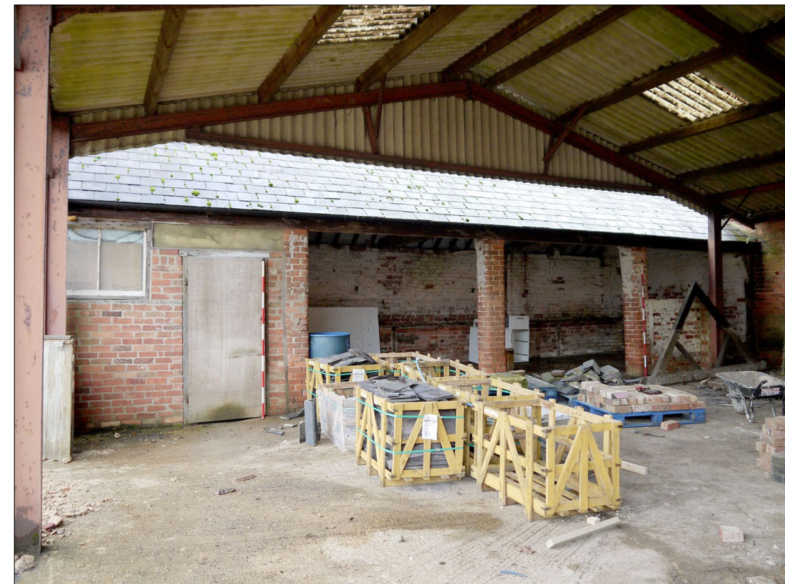
27. Building 5 (open-fronted cow house). Facing W
