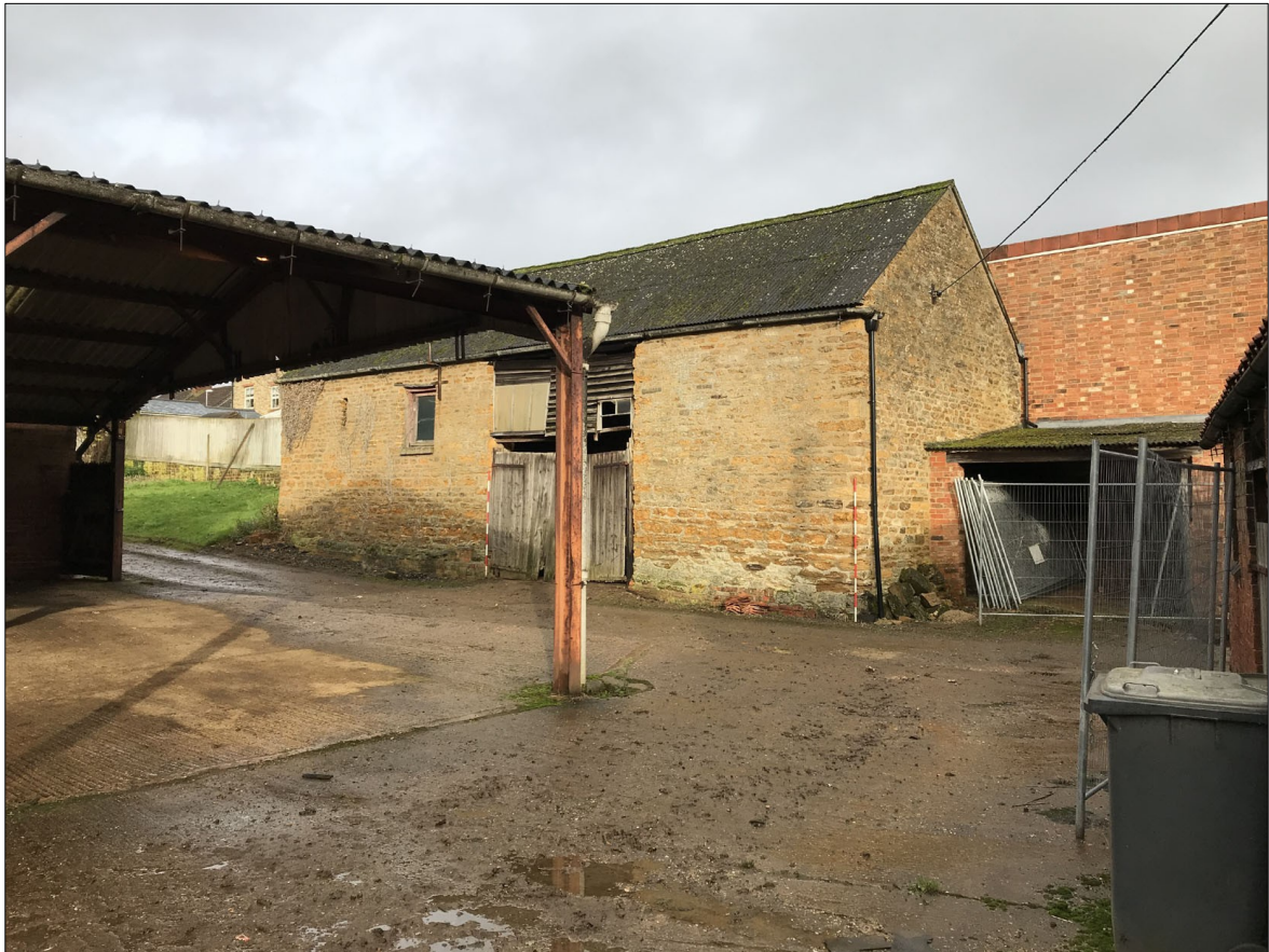
19. (Below) General view of Building 1 from farmyard and farmhouse. Facing NE
