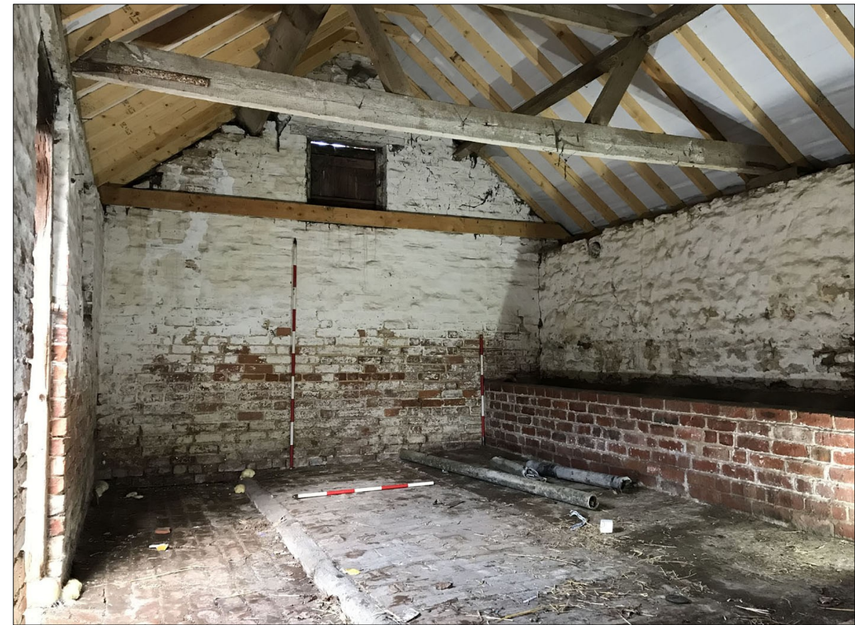
62. Interior of Building 6 (cow house). Manger to R. Facing NE
