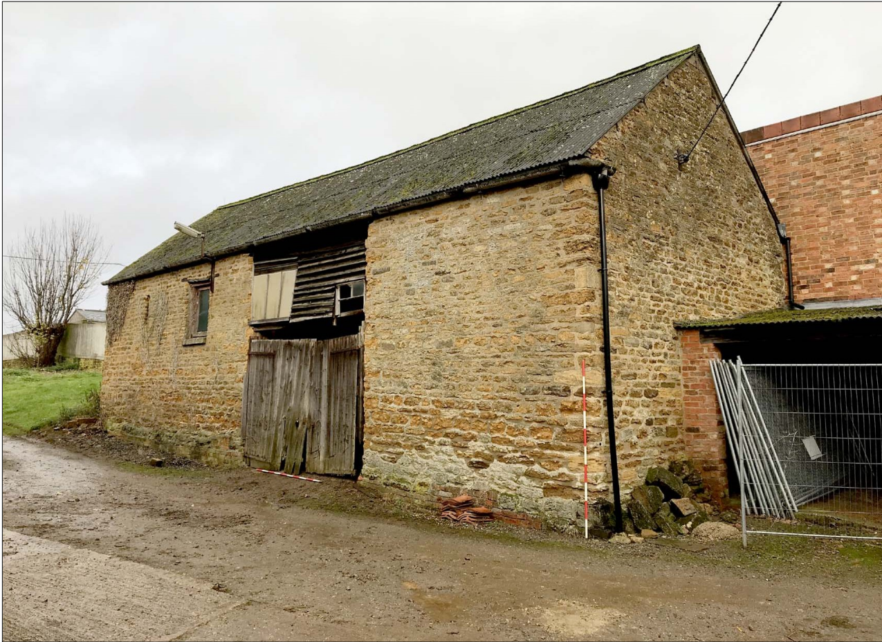
5. Building 1 (the stone barn). Facing NNE
