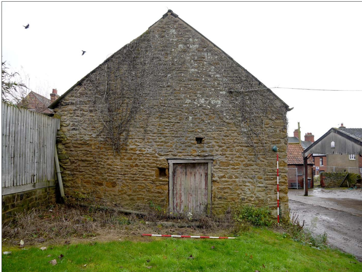
9. Building 1 (the stone barn). NW gable end. Facing SE
