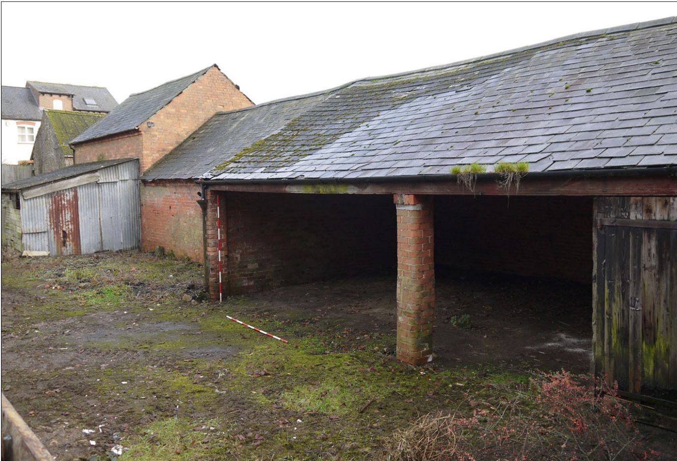
18. Building 4 (open shelter). Facing E
