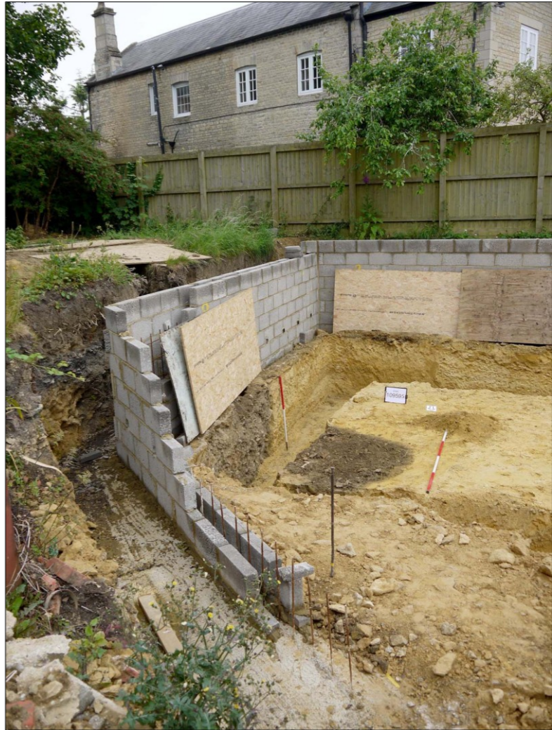
Above: 12.06. 2020. Overview, facing SE
