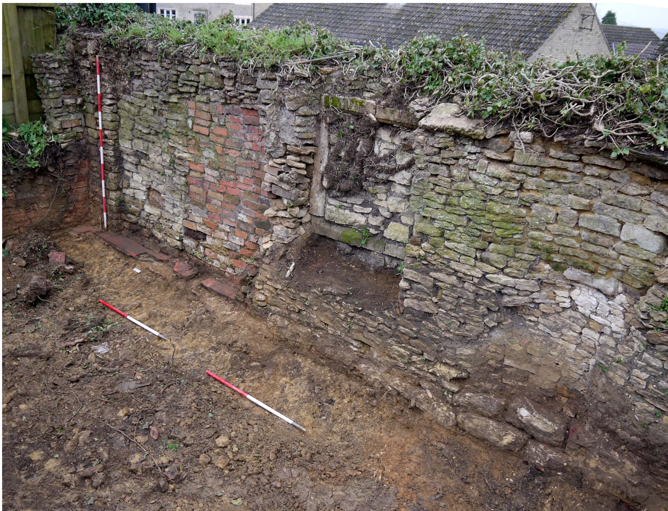
Figure 16. Former front interior wall of the cottages, facing SW (15.03.2020)
