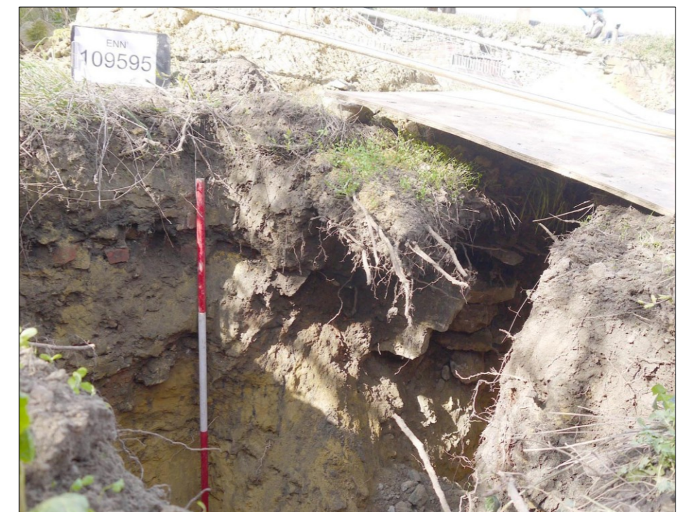
Above: 23.03.2020. Cottage walls exposed in trench for new soak-away. Facing W
