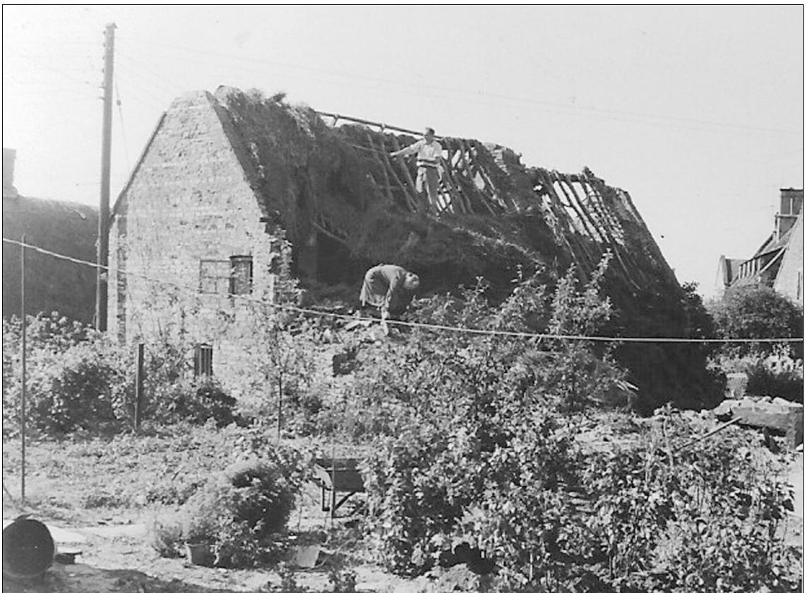
Figure 26. Demolition of Japonica Cottage, 1959
