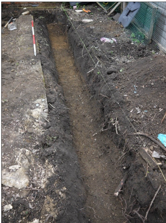
Photo 2. Overview of northern foundation trench. Facing WNW
