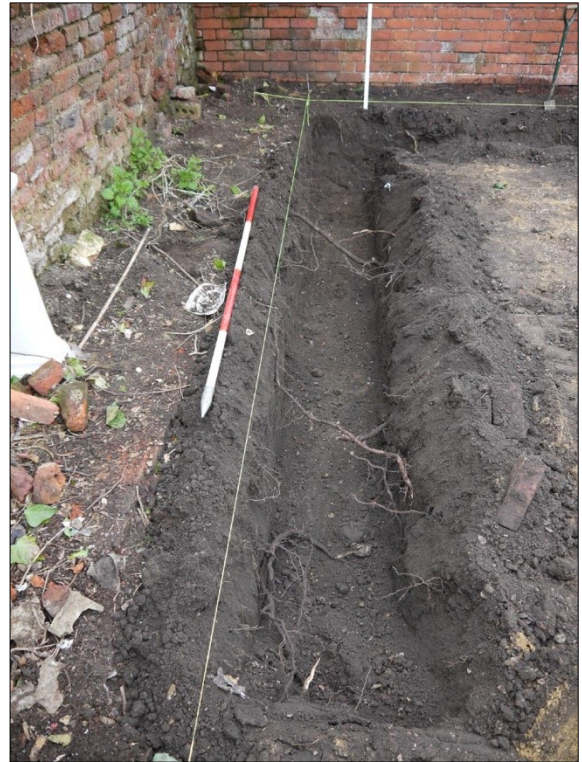
Photo 6. Overview of southern foundation trench. Facing W
