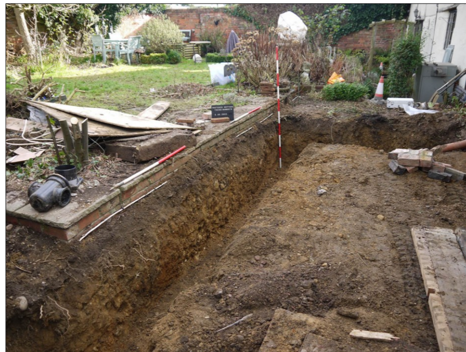
P5. Foundation trench (Section 1), facing SE
