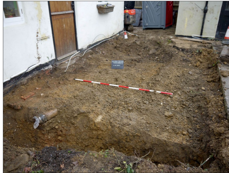
P2. Initial ground reduction throughout the new conservatory footprint. Facing NW
