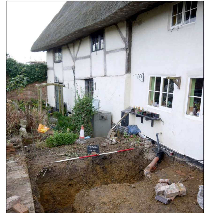
P3. Overview of foundation trench, facing SE
