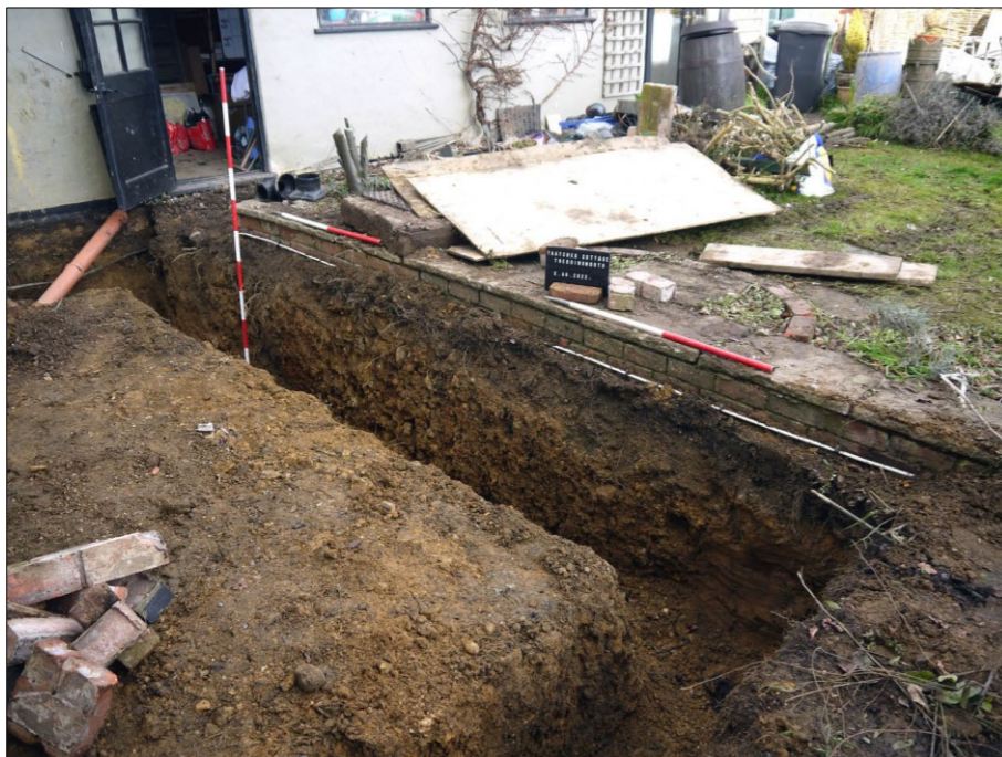
P4. Over view of foundation trench (Section 1), facing SE
