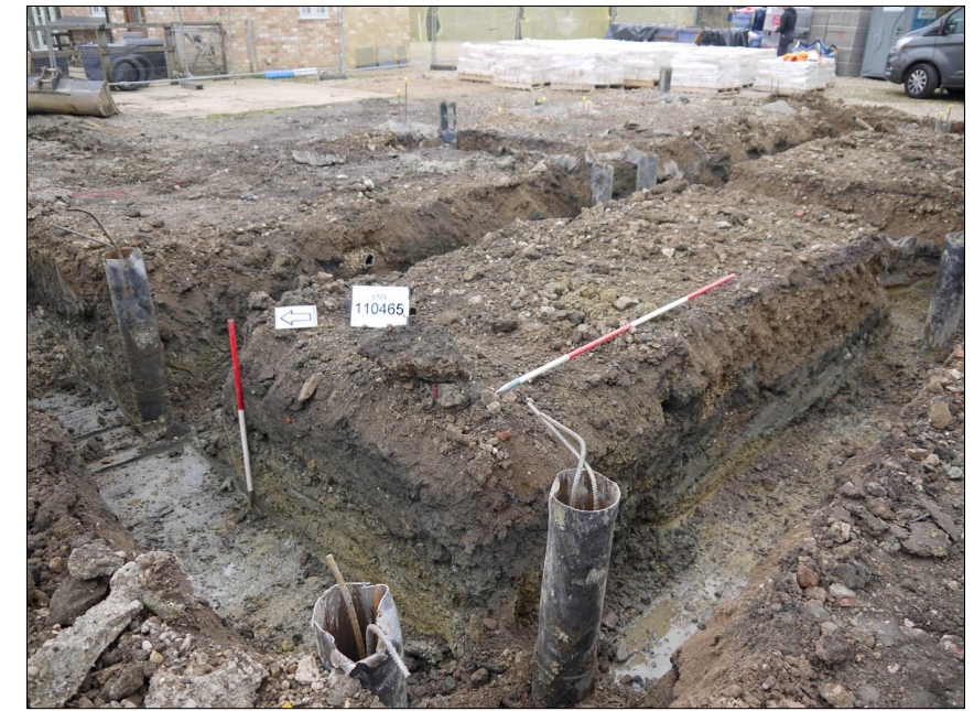
P9. House foundation trench. Facing SE
