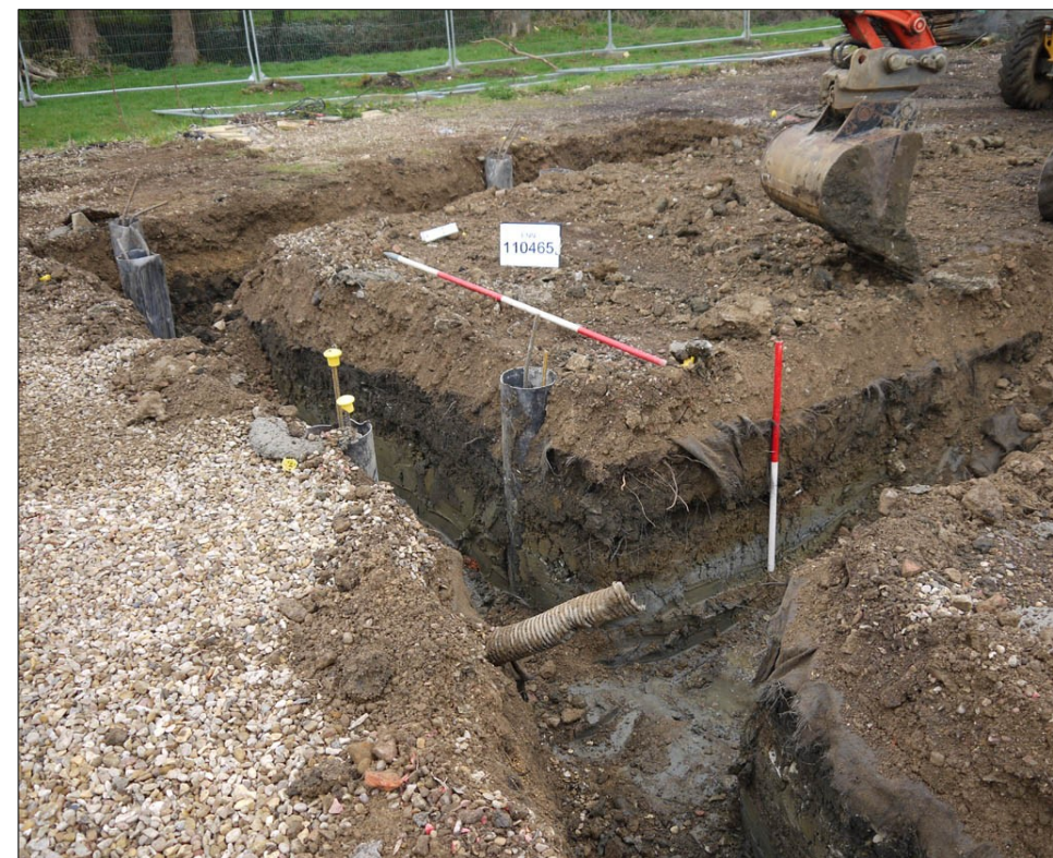
P5. House foundation trench. Facing NW
