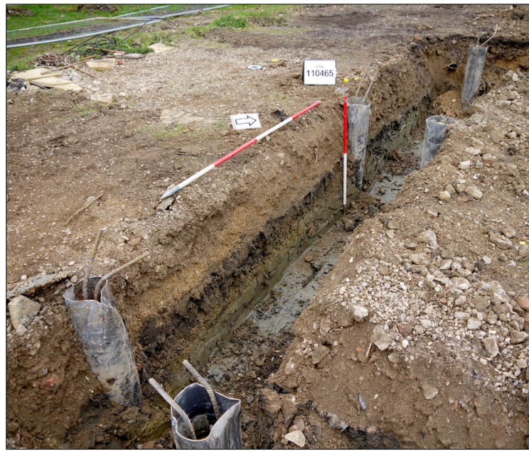
P7. House foundation trench. Facing NW
