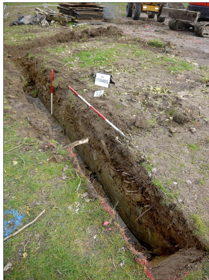
P4. Garage foundation trench. Facing N
