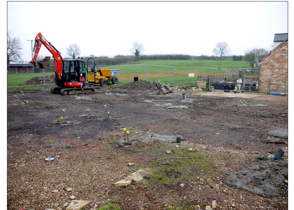
P3. Pre-commencement overview. Facing NE
