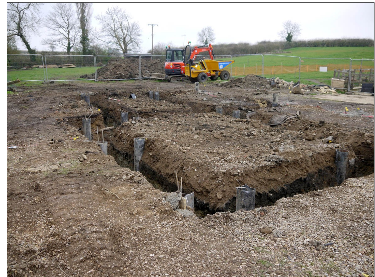
P11. Overview of house foundation trenches. Facing NNE
