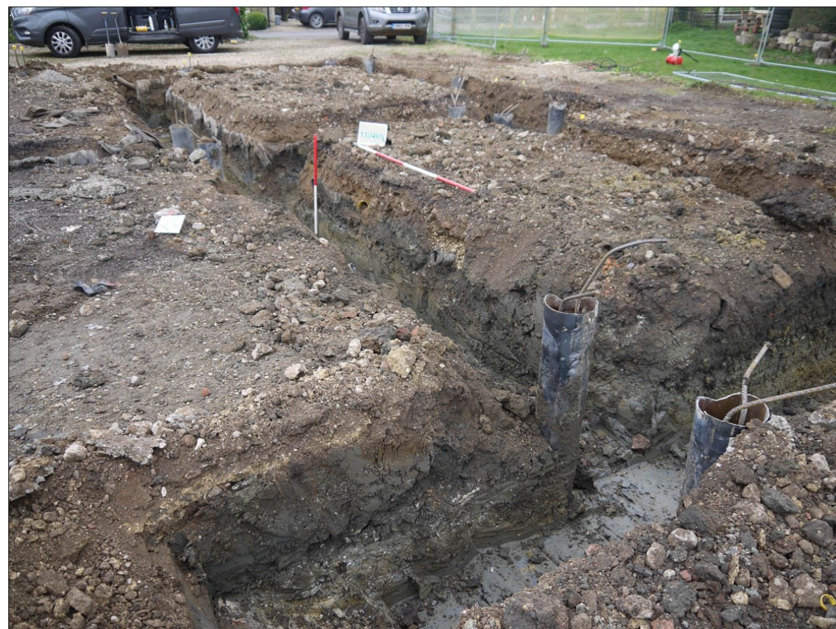
P10. House foundation trench. Facing SW
