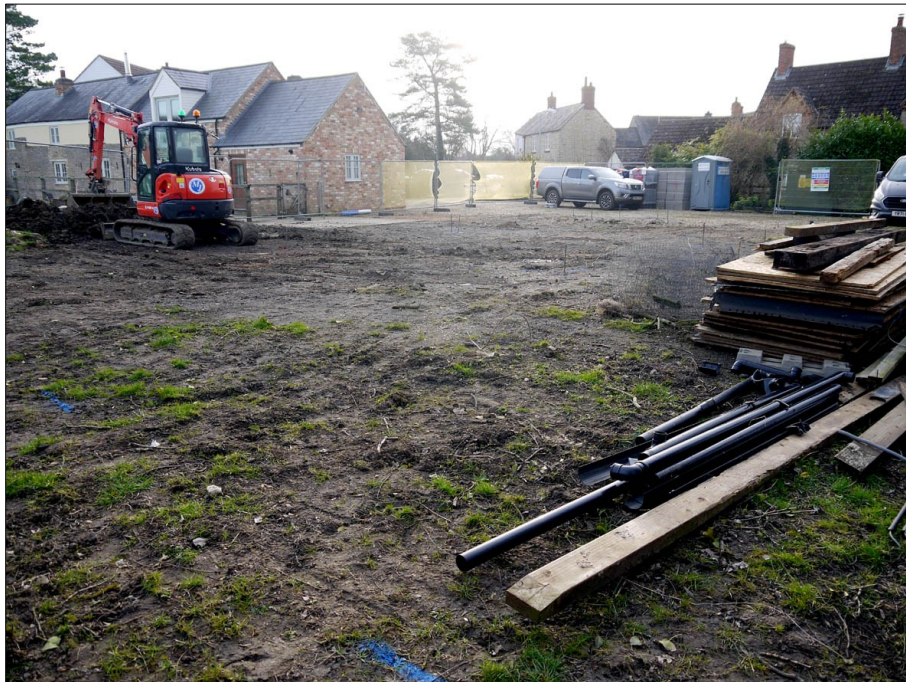
P1. Pre-commencement overview Facing SE
