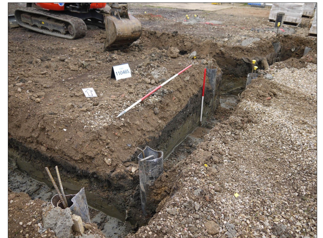
P6. House foundation trench. Facing NE
