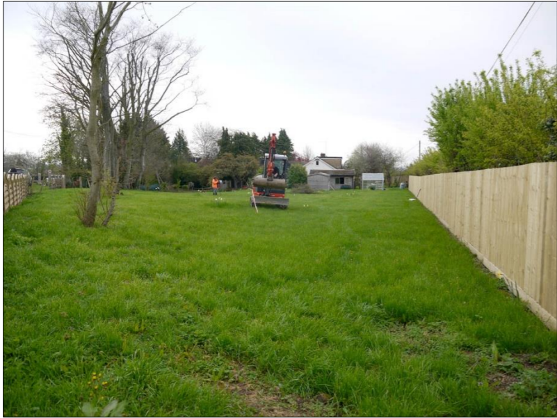
P1. Pre-commencement site overview, facing SE
