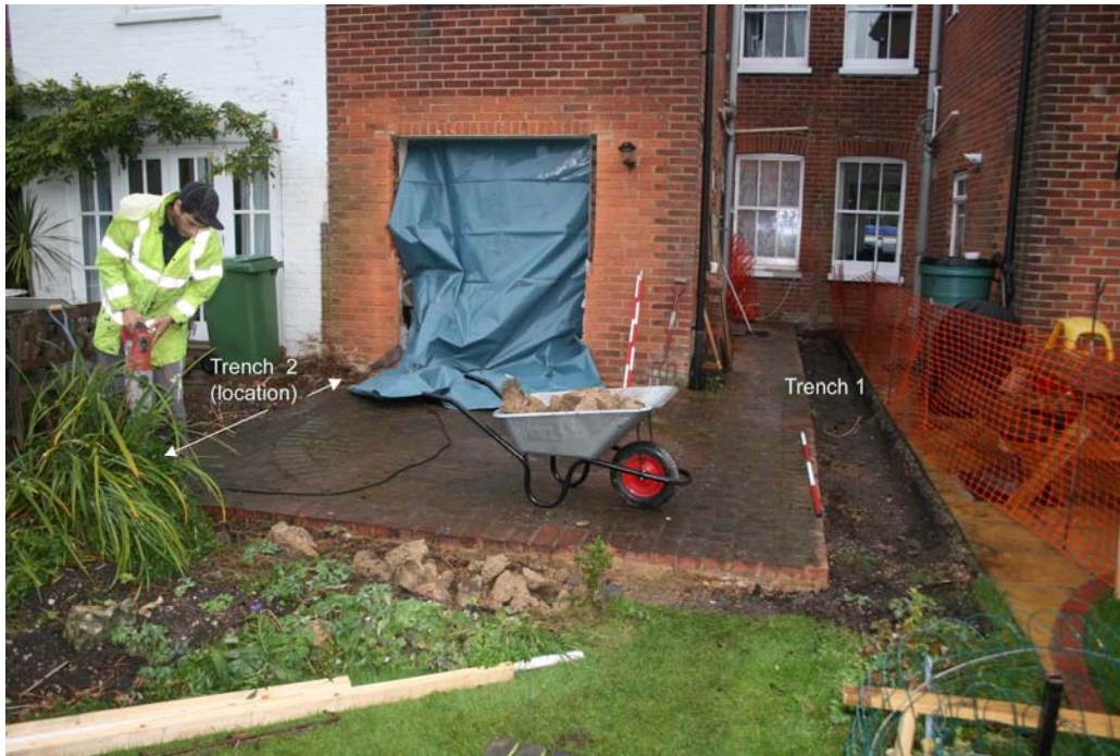
Plate 1. Overview of site, facing north
