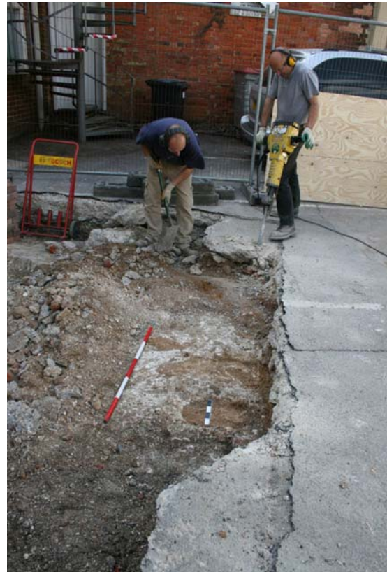
Plate 4: Depth of modern overburden; Features 1, 3, 5 & 8, facing north-west
