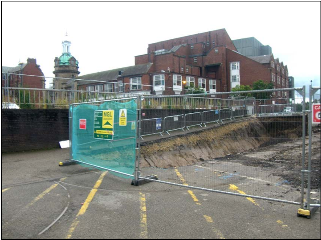
Plate 1: Trench 1, looking south-west towards the rear of the Sunderland Empire Theatre.
