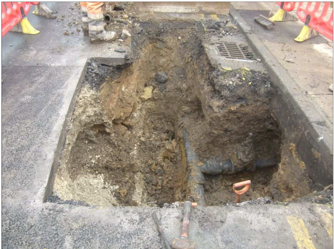
Plate 1: pit on Horsefair showing backfill of existing services
