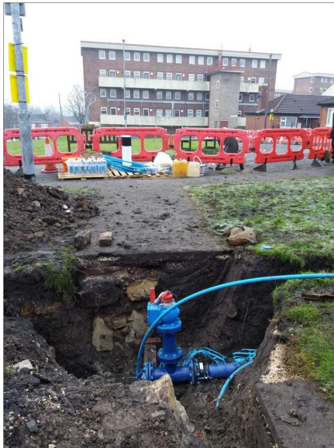
Plate 3: Wall 1, behind valve gear, facing south-east
