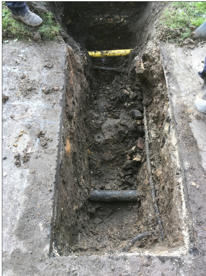
Plate 1. Trial Pit 1, 10 Micklegate Square
