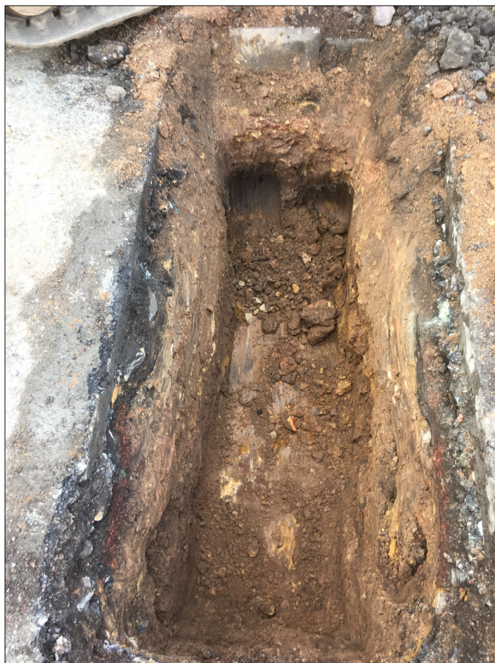
Plate 2. Trial Pit 2, 32 Bede House Villas
