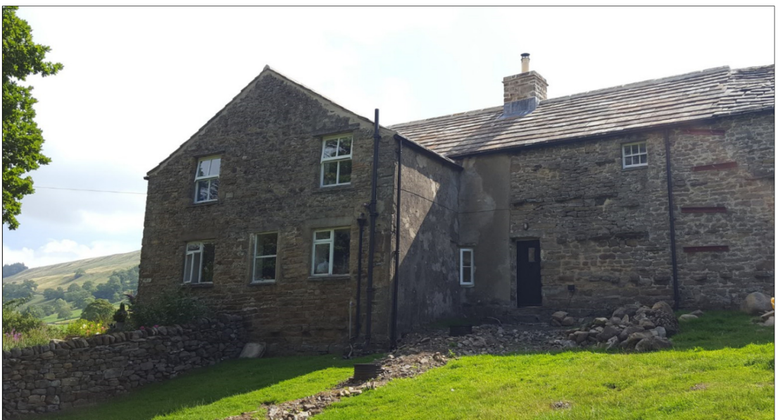
Plate 3: view of west facing (rear) of farmhouse showing two-storey extension.
