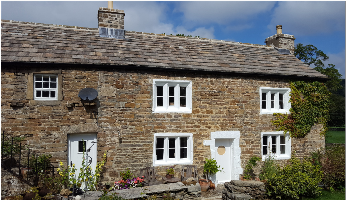
Plate 2: view of east facing (main) façade of farmhouse.
