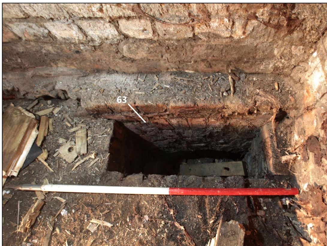
Plate 6: opening 62 in sub-basement floor showing brick arch 63 in the east wall.
