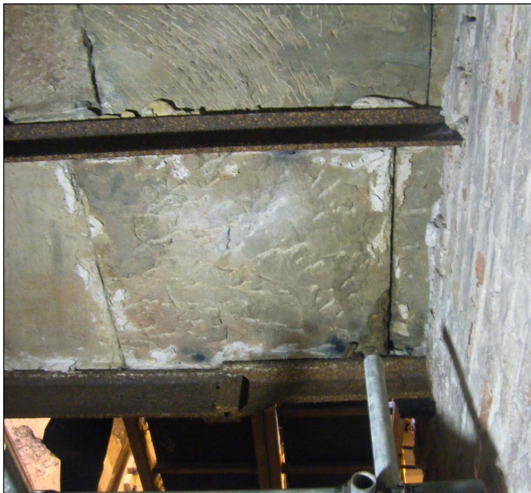
Plate 3: underside of the original sandstone floor surface (110) of the west engine house.
