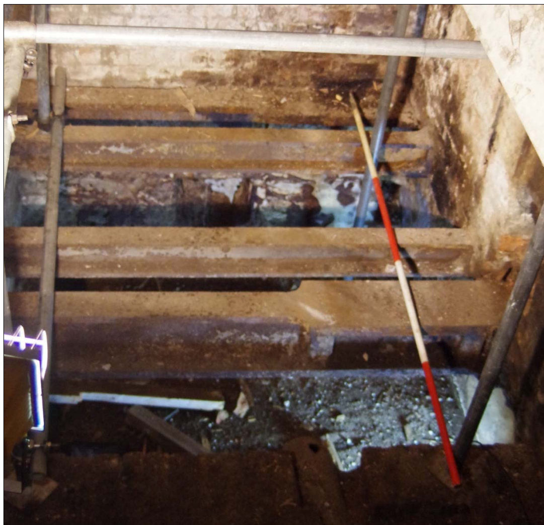
Plate 5: iron girders 53 over sub-basement level 60.
