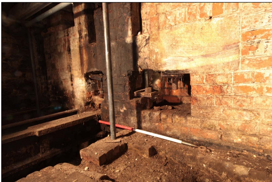
Plate 9: anchoring mechanism 31 within west wall (30) of the pumping chamber, facing south-west.
