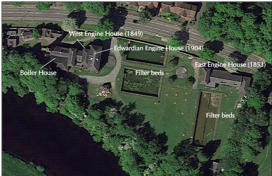
Figure 2: Google Earth aerial image showing the pumping station complex with key elements annotated.
