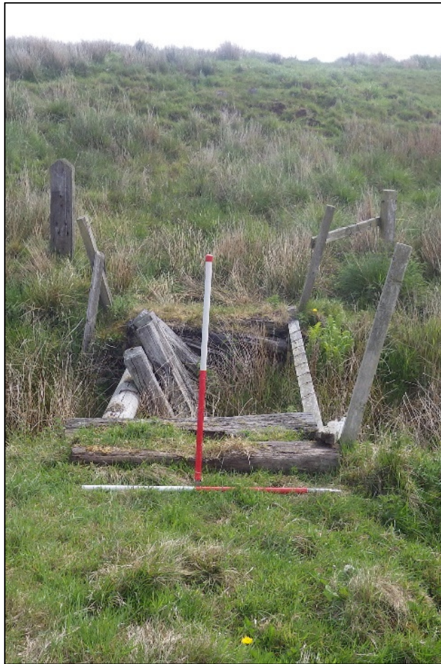
Plate 38: the adjacent bridge looking east.
