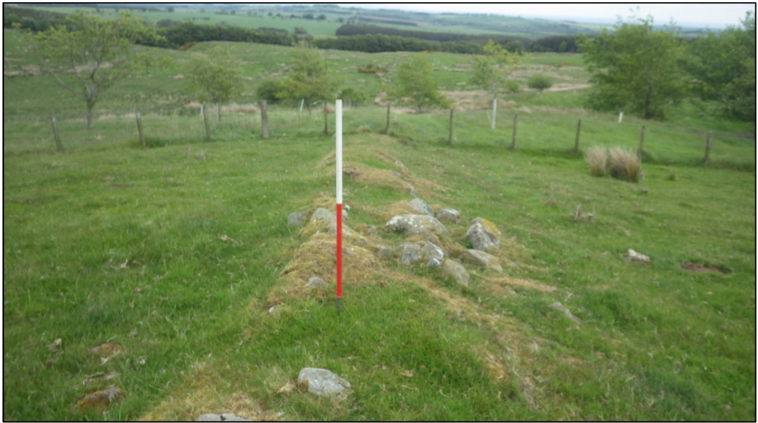
Plate 19: boundary wall 110 looking east.
