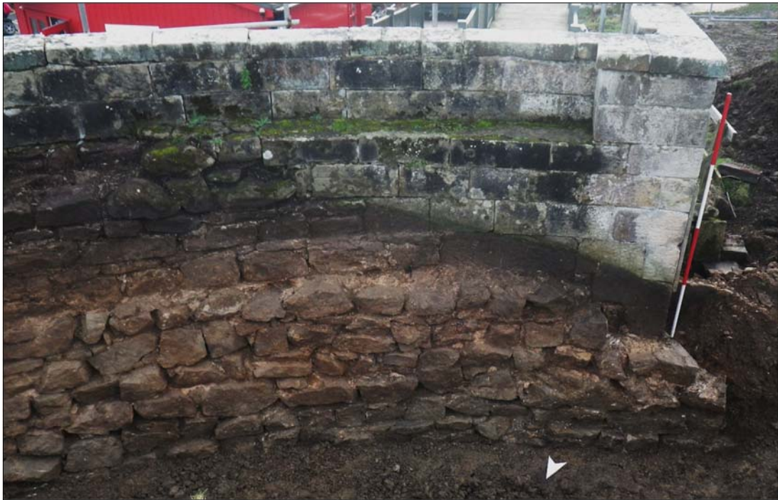
Plate 3: stepped construction courses within the entrance to the bastion, with ashlar courses at and above the turfline.
