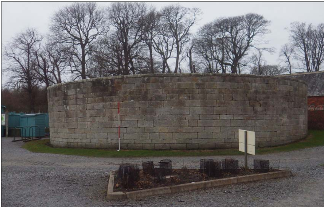
Plate 2: external face of north-west bastion, facing south-east.
