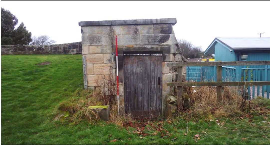
Plate 6: gateway 23 prior to excavation showing the slope of the bastion bank.
