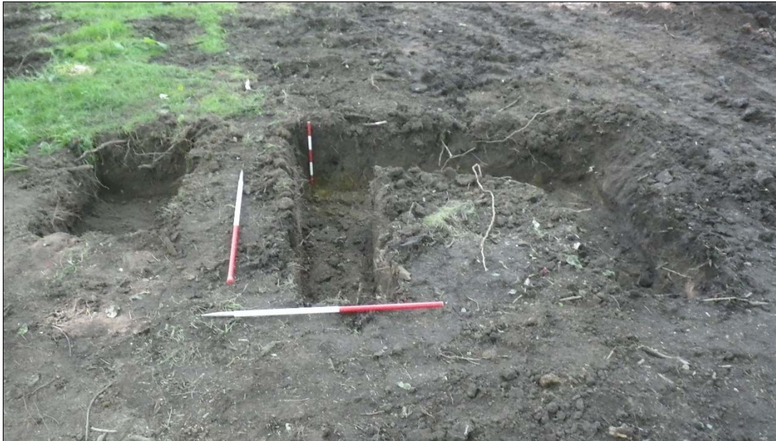
Plate 25: foundation trenches for the playground equipment in the north-west woods.
