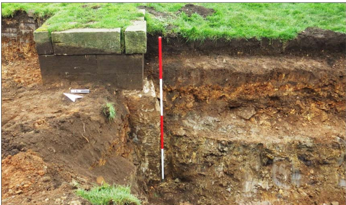
Plate 5: excavation through the infill of the bastion with exposed statue plinth 24 (facing east).
