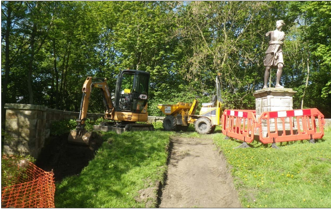
Plate 9: initial machine excavation and removal of soil within the north-west bastion.
