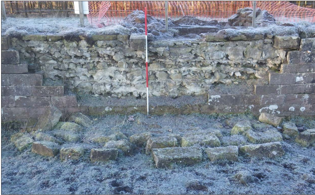
Plate 13: southeast-facing section of wall 34 with collapsed ashlar facing and heavily mortared rough-coursed inner face exposed. Investigation test pit just visible to the rear.
