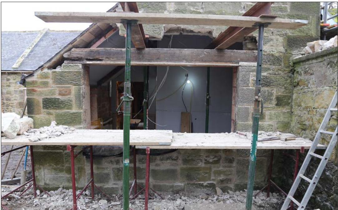
Plate 20: cartshed; west-facing gable-end window lintel during removal.
