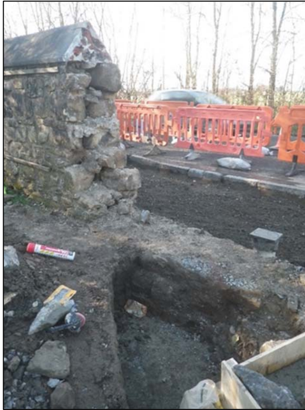
Plate 34: northern boundary wall 147 during the enlargement of the exit.
