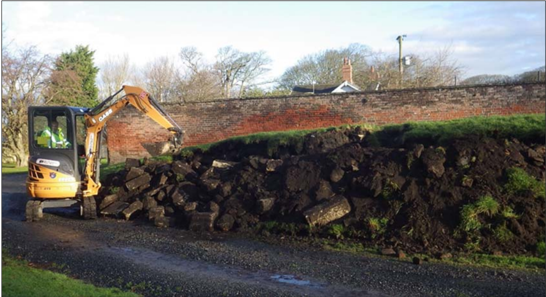
Plate 35: removal of the turfed mound at the commencement of site works.
