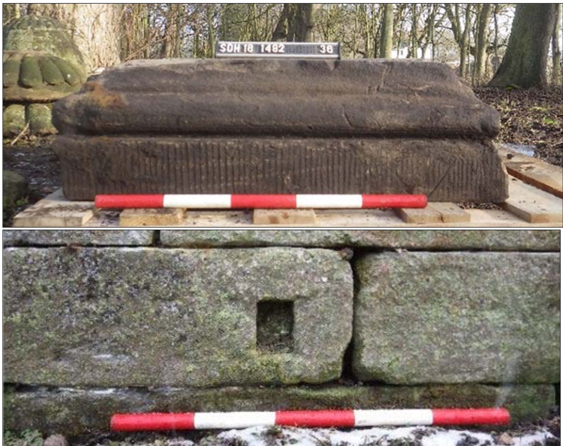
Plates 43,44: (top) stone plinth 36 and (bottom) carved recess 79 in bastion wall for gate.
