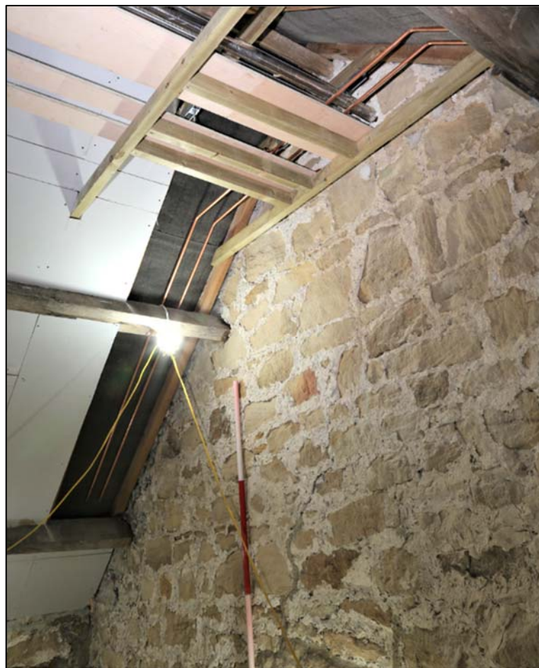
Plate 25: south-facing side of the partition wall apex, showing differential wear of the stonework extending down the wall.
