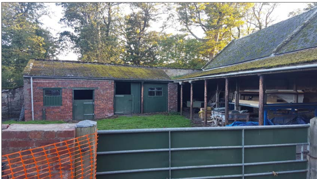
Plate 12: late 19th-century lean-to implement shed (right) and brick-built stable block (left) both demolished as part of the development.
