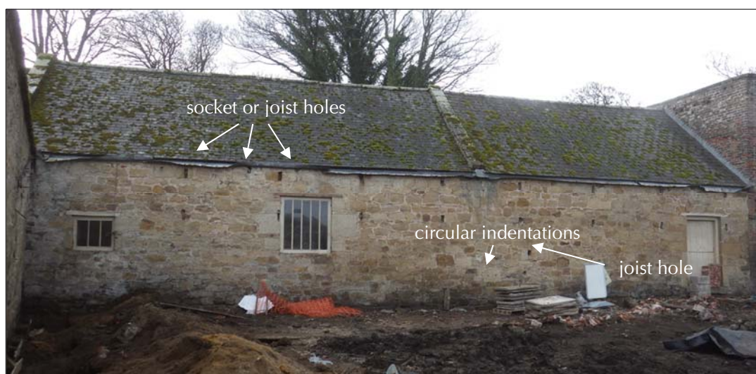
Plate 13: east-facing elevation of brewhouse following the removal of the lean-to structure.
