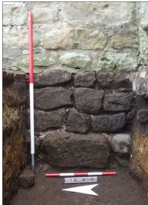
Plate 11: brewhouse foundations (53) at the south-east corner of the cartshed.
