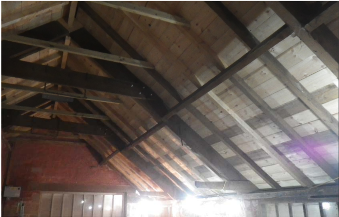
Plate 4: roof structure prior to removal.
