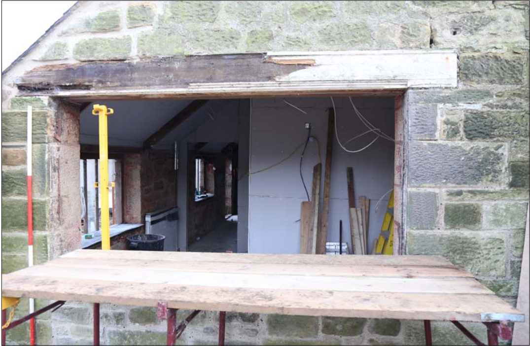
Plate 19: cartshed; west gable-end window lintel prior to removal.
