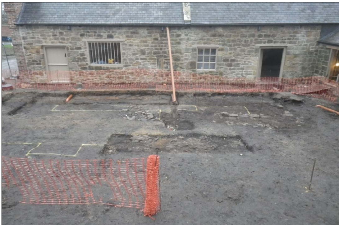
Plate 31: hand clearance and excavation within the brewhouse terrace.
