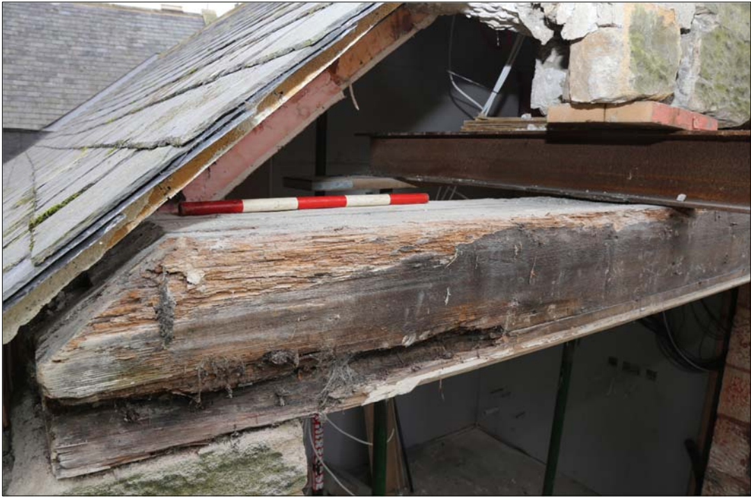
Plate 21: detail of northern end of lintel, cut to accommodate later roof line.
