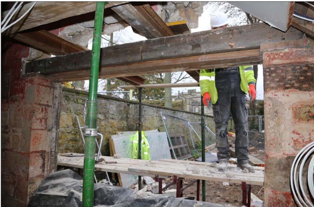
Plate 22: cartshed; east-facing view of gable-end window lintel during removal.
