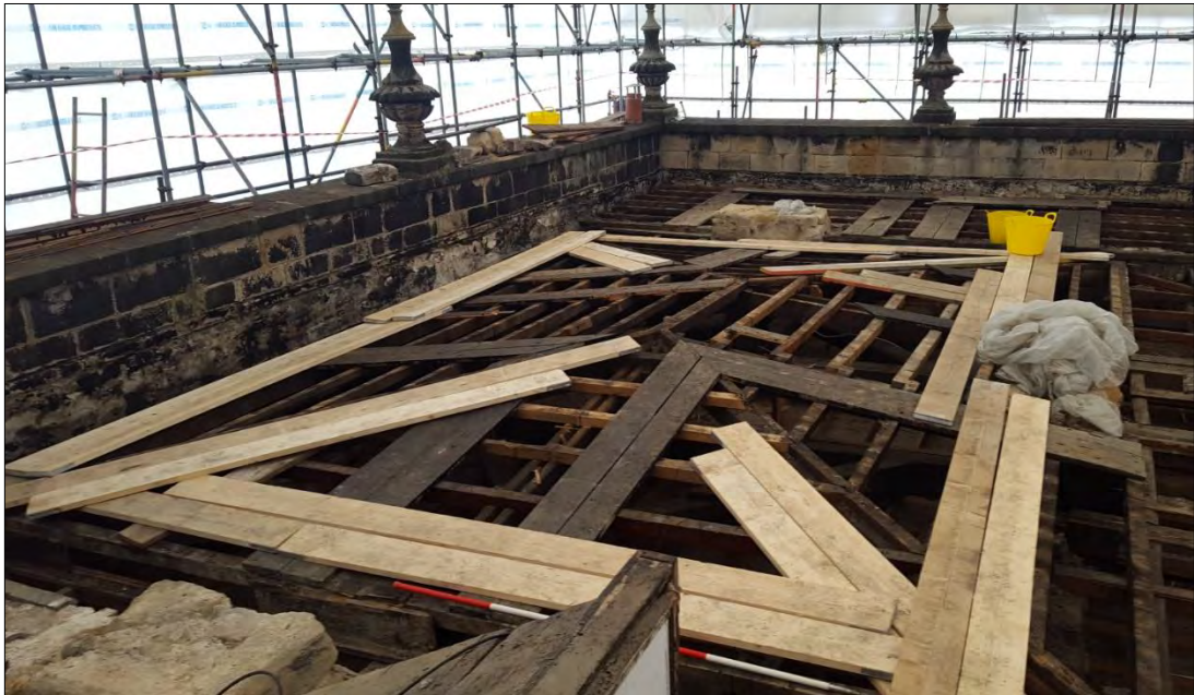
Plate 10: north range looking east across northern hipped roof (111).
