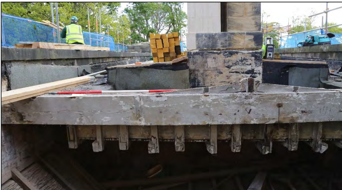
Plate 116: truss 700; looking east with the purlins visibly supported from the truss above.
