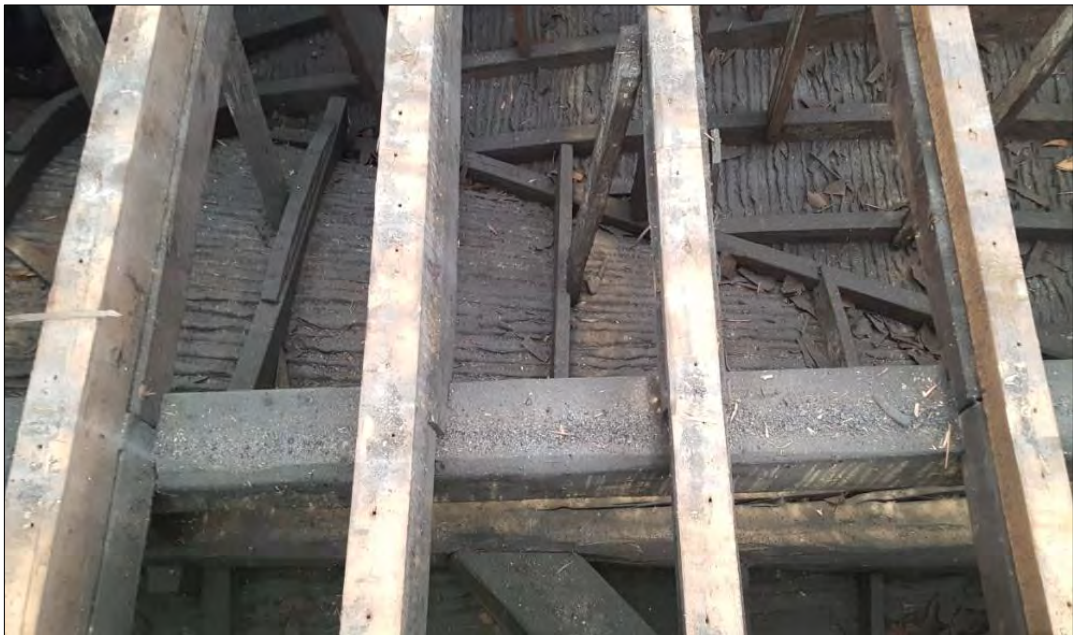
Plate 27: detail of vaulted and groined ceiling structure beneath central range.
