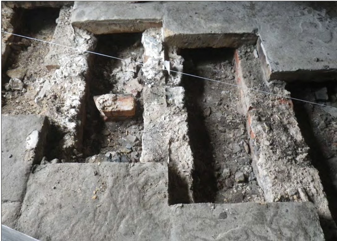
Plate 124: brick support structure 170 after lifting of flagstone floor 169.
