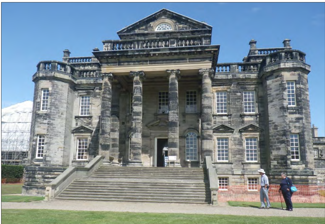
Plate 102: south portico steps prior to repair.
