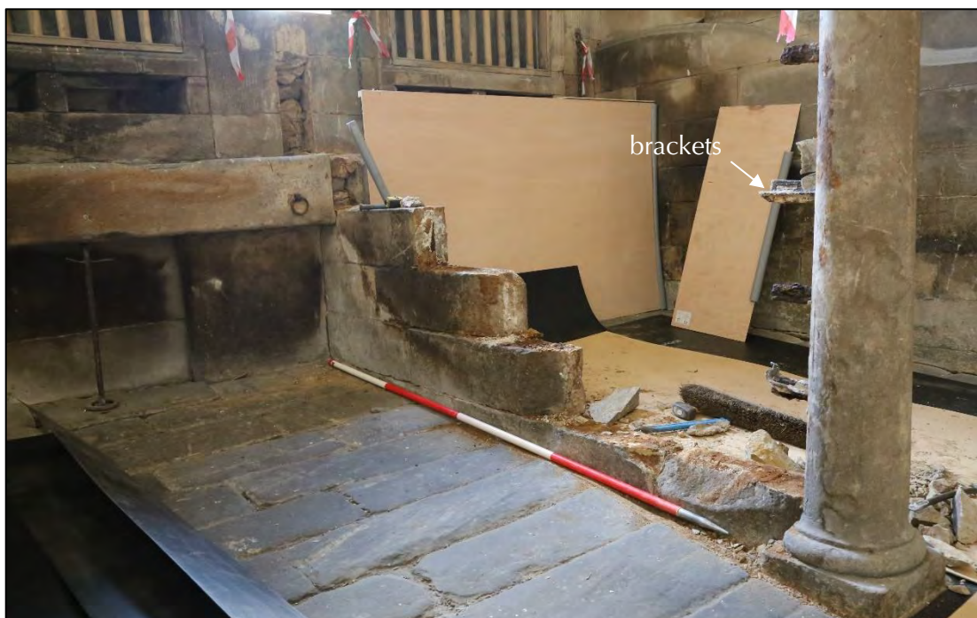
Plate 136: dismantled divider S09; view is south-east toward the trough, with iron brackets visible along the post. The remainder of the divider could not be removed because it supported the trough.
