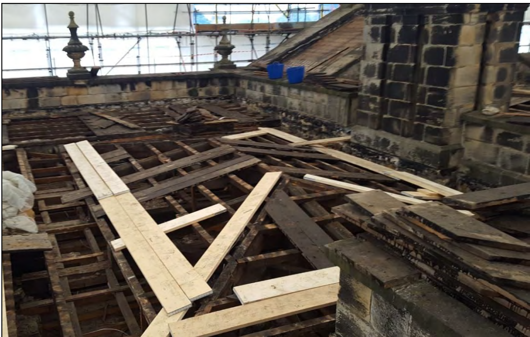
Plate 11: the south hipped roof (112), looking north-east towards the pediment chamber.
