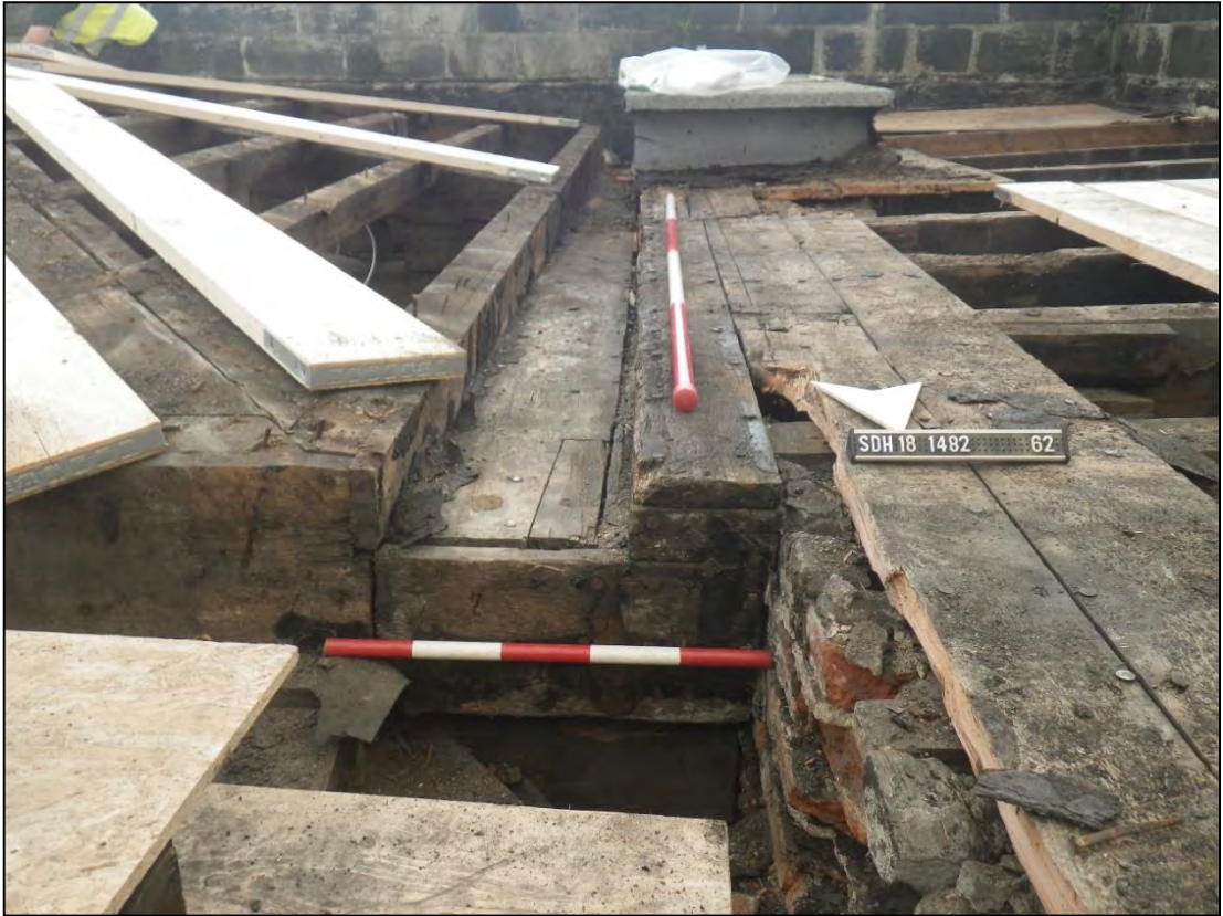
Plate 39: gutter 146 looking south. Chimney 109 can be seen at the end of the ranging rod.
