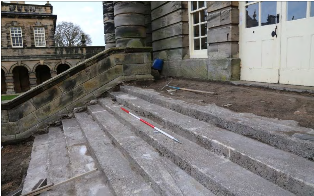
Plate 107: concrete risers of the upper landing.
