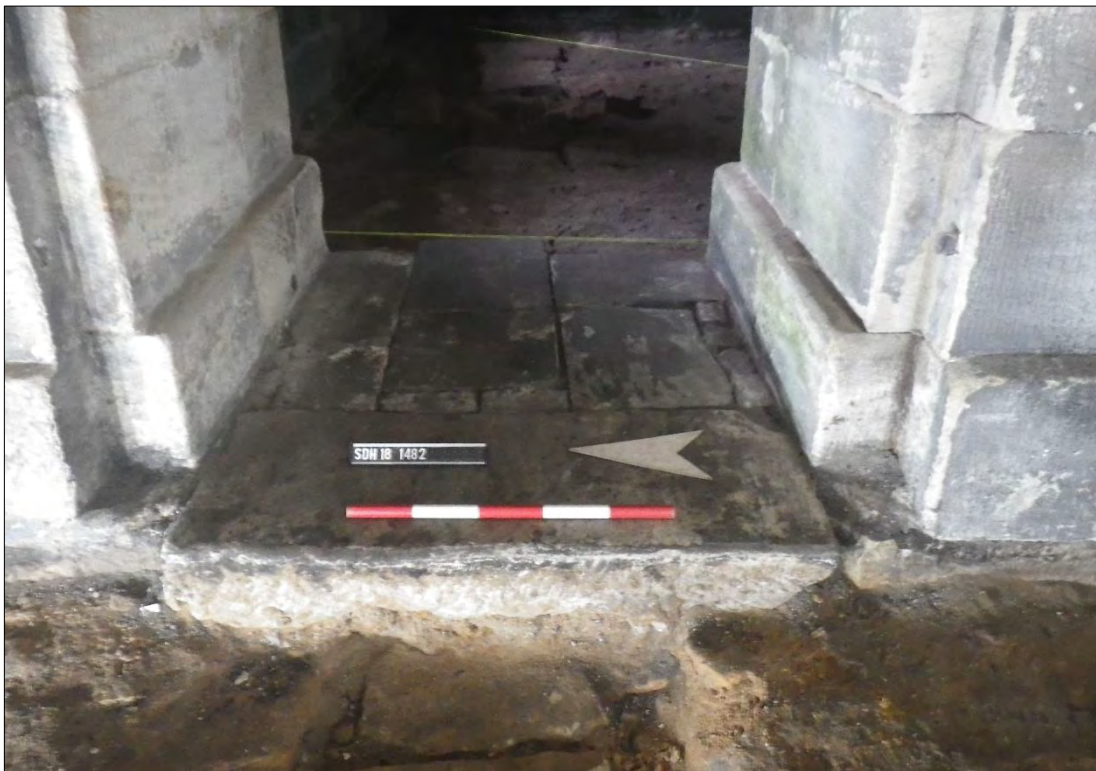
Plate 77: remains of flagged floor 132 in the doorway between the pantry and Housekeeper's Room.
