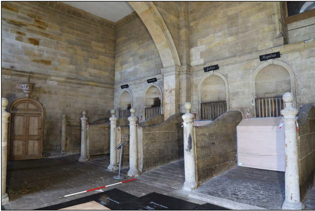
Plate 133: stall dividers S08 , S07 , S06 , S05 and S04 along the west wall of the stable. The bars of the hay racks in the arched recesses can just be seen.
