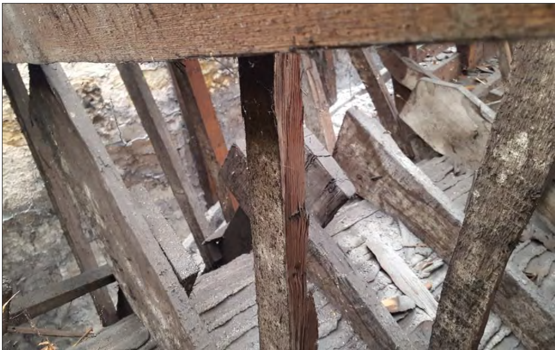
Plate 23: crossing braces carrying the vaulted ceiling structure beneath.
