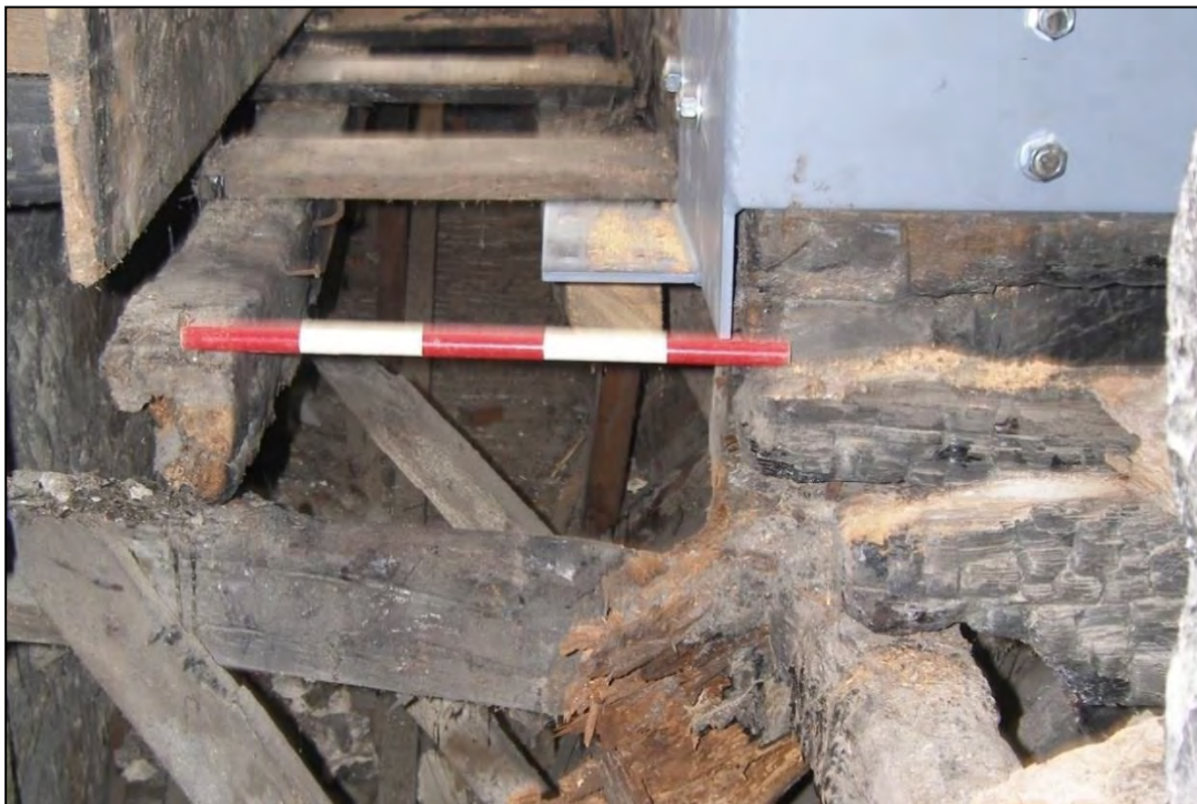
Plate 33: evidence of charring is visible on the timbers adjacent to gutter 121.
