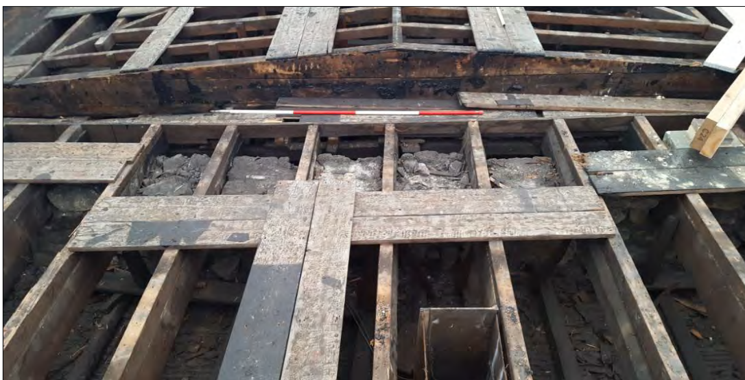
Plate 19: detail of the inserted gable and flat roof (123).
