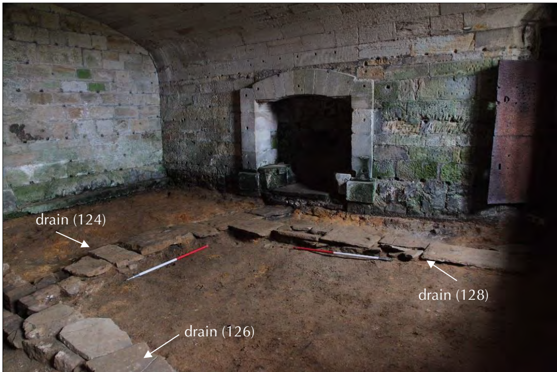
Plate 91: B08 with drain network 123/124/126 and fireplace 212, facing north-east.
