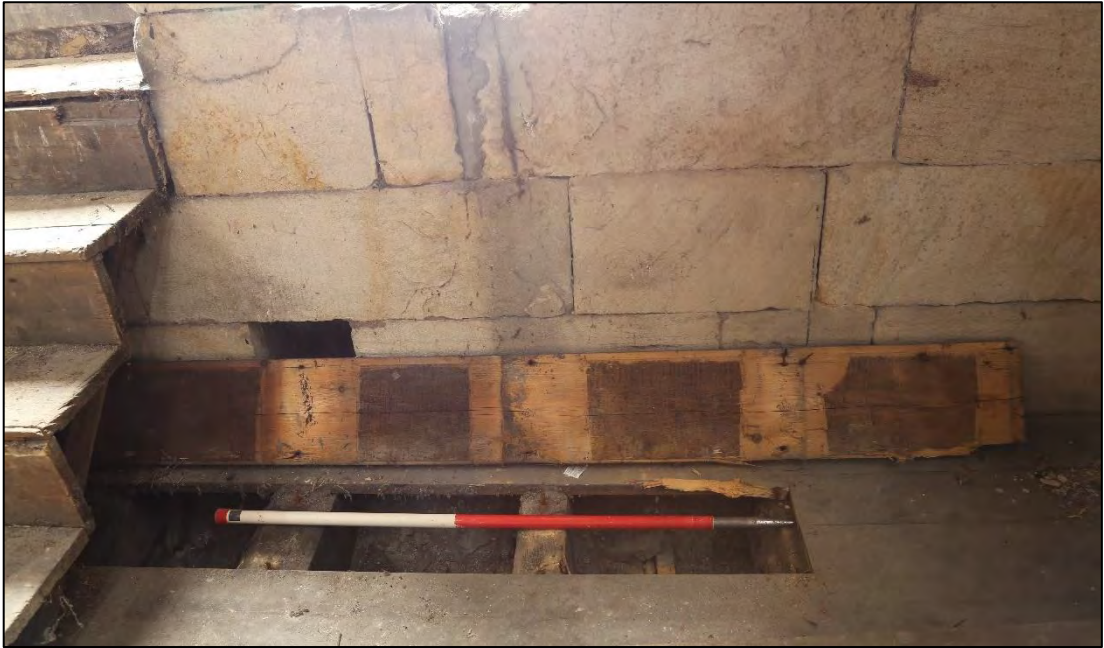
Plate 52: removed floorboard of the clocktower. The access steps are visible to the left (south).
