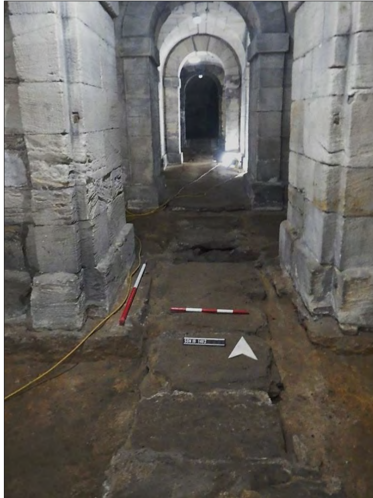
Plate 78: drain 118 running north through the centre of the basement.
