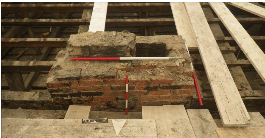
Plate 6: chimney 107 during dismantling, looking south.
