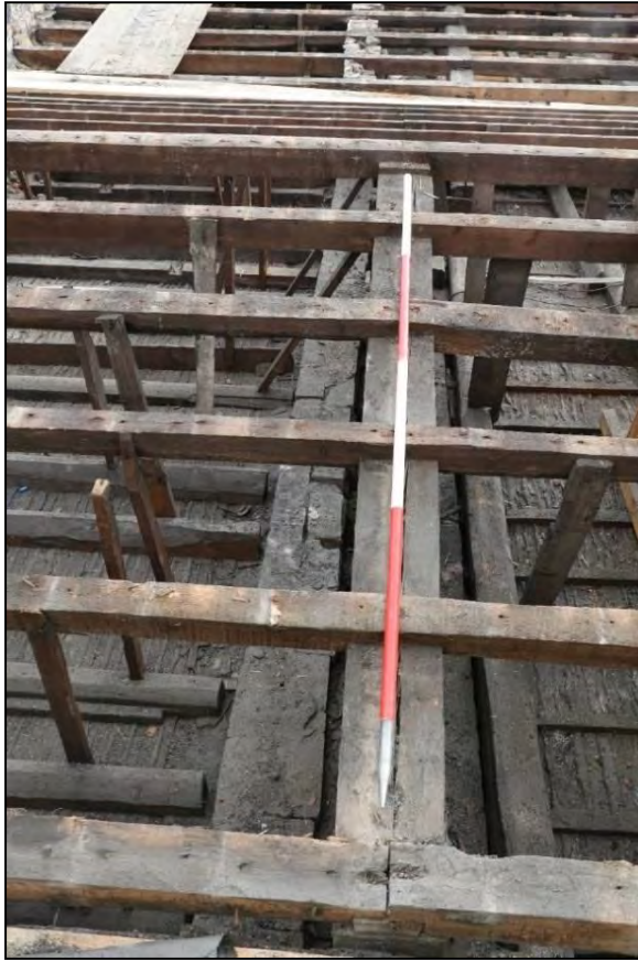
Plate 422: truss 208 on roof 143, looking south.
