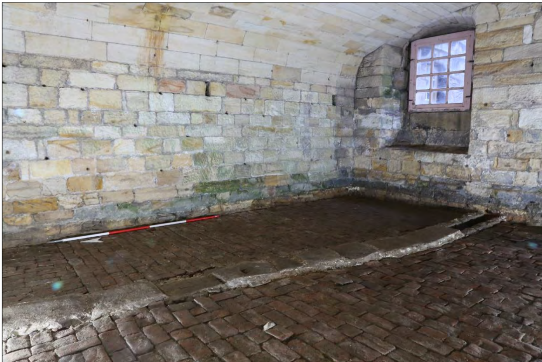
Plate 96: drain 134 and brick surface 133 in B10, the Footmen's Room, facing south-east.
