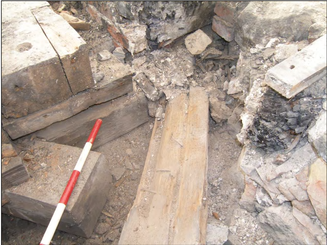
Plate 38: charring of the trusses of roof 145 visible at the junction of truss 203 and 204.
