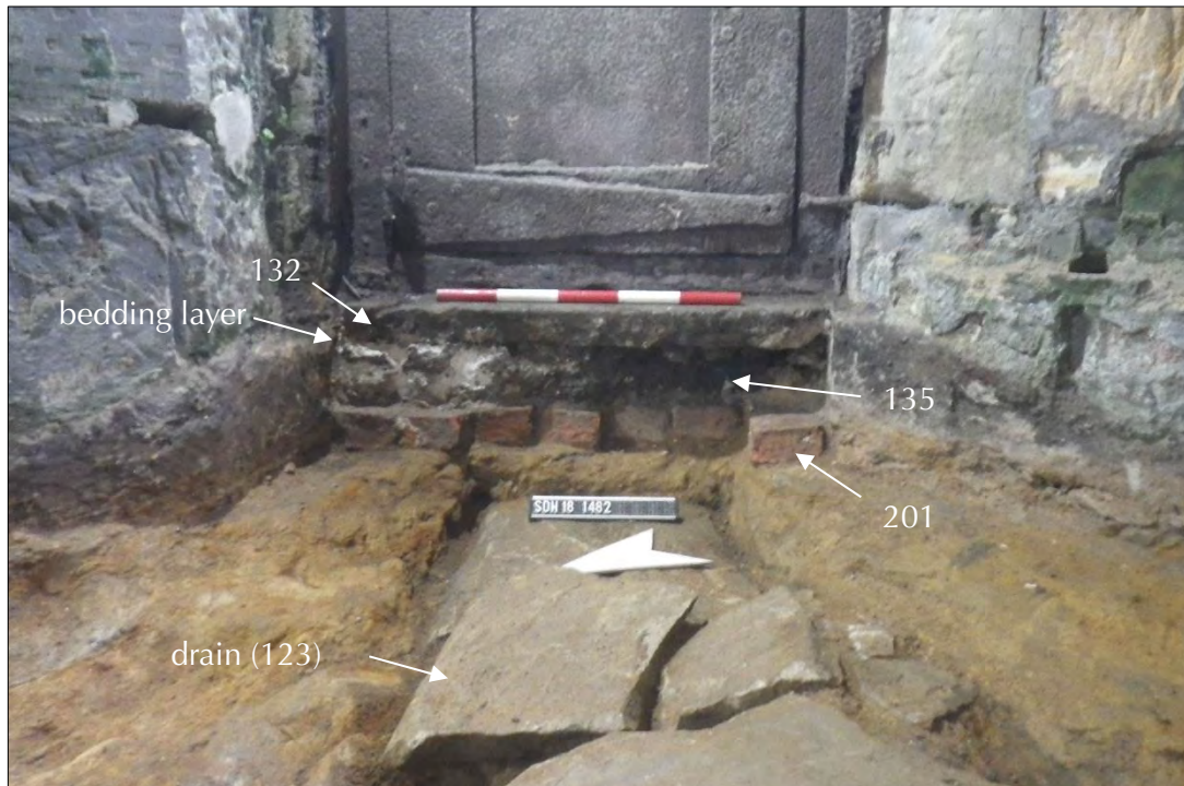
Plate 95: section showing sequence of basement deposits as preserved beneath the door to the silver safe. Drain 123 in the foreground.
