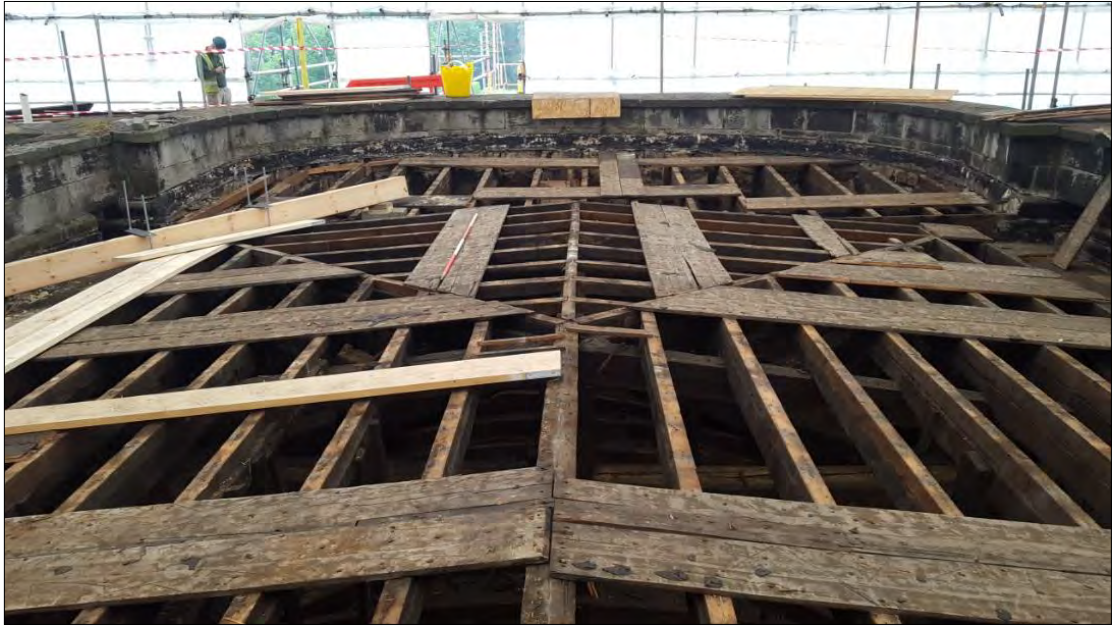
Plate 20: looking east across the west end of the central range towards the apsidal bay, showing the modifications to the earlier hipped section (124).
