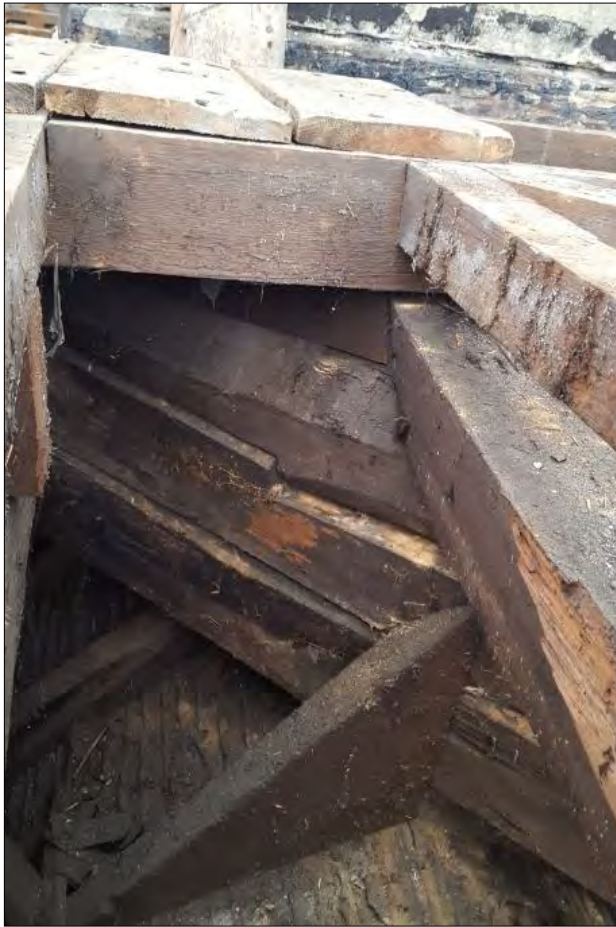
Plate 22: north-west hip truss. This is carried over the ceiling vaulting, visible beneath. It has subsequently been built up to support the gable roof and the insertion of a later tie beam.
