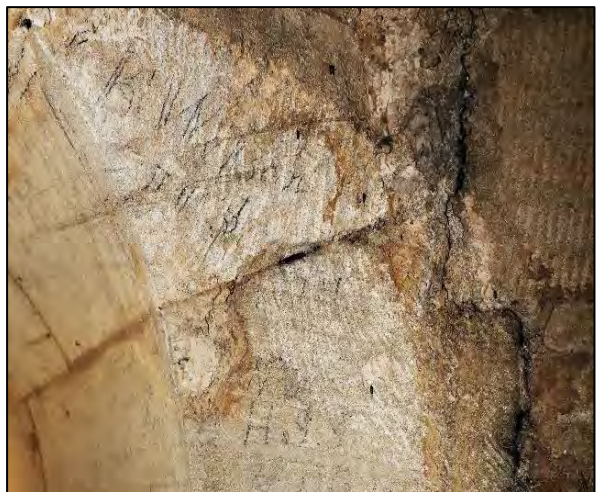
Plate 72: graffiti beside door to s400, looking north-west.
