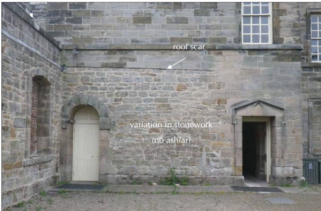
Plate 130: east-facing wall profile with traces of the former south range.
