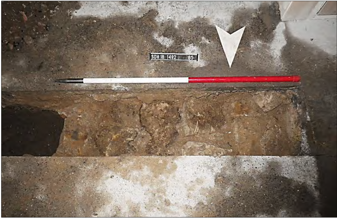
Plate 127: upper surface of culvert 65 directly beneath the concrete floor surface in the passage between the central stables and south block.
