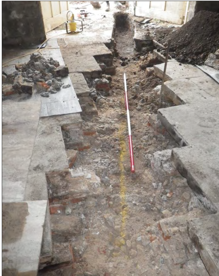
Plate 126: interior of the Carriage House after removal of flagstone floor 169 and brick supports 170, with the service trench cutting courtyard soil 168 in the doorway.
