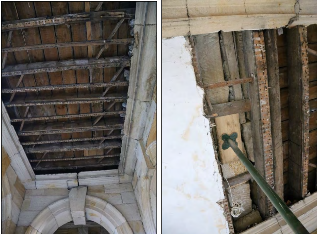
Plates 48, 49: (left) ceiling configuration on the north side of the arcade with secondary timbers and braces, and (right) arrangement on the south side without secondary supports.
