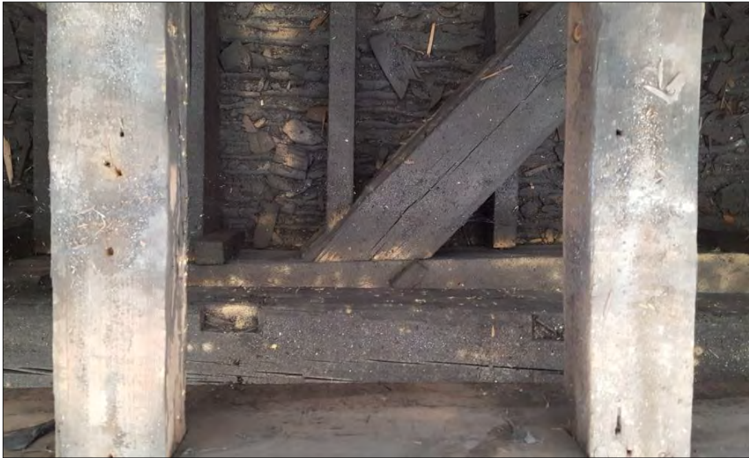
Plate 24: evidence of timber reuse or reconfiguration visible on the joist running below the central ridge of roof 122.
