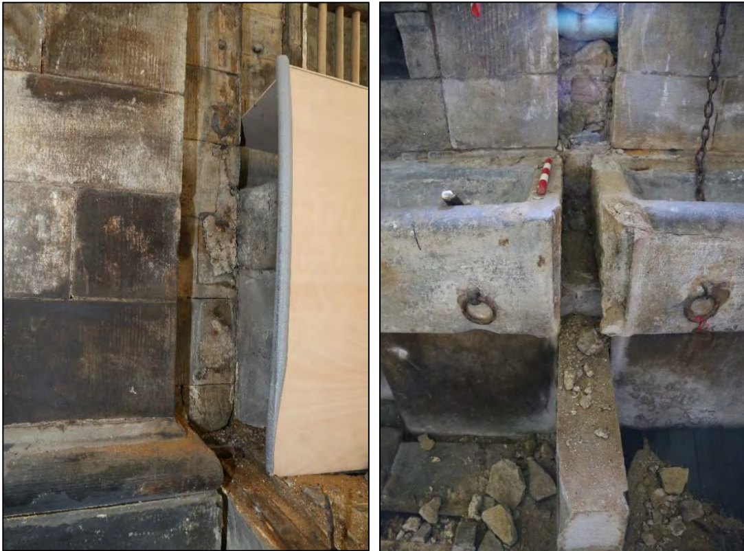
Plates 139, 140: (left) lead-filled notched in wall of divider S10; (right) troughs on either side of divider S09.
