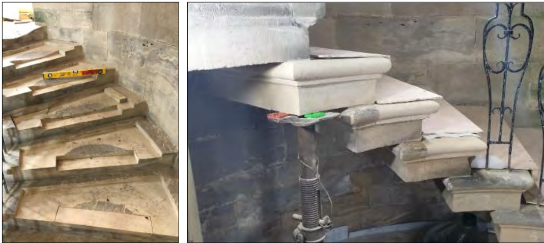
Plate 108: primary and secondary indents in west stairs. Image provided by HPR.
