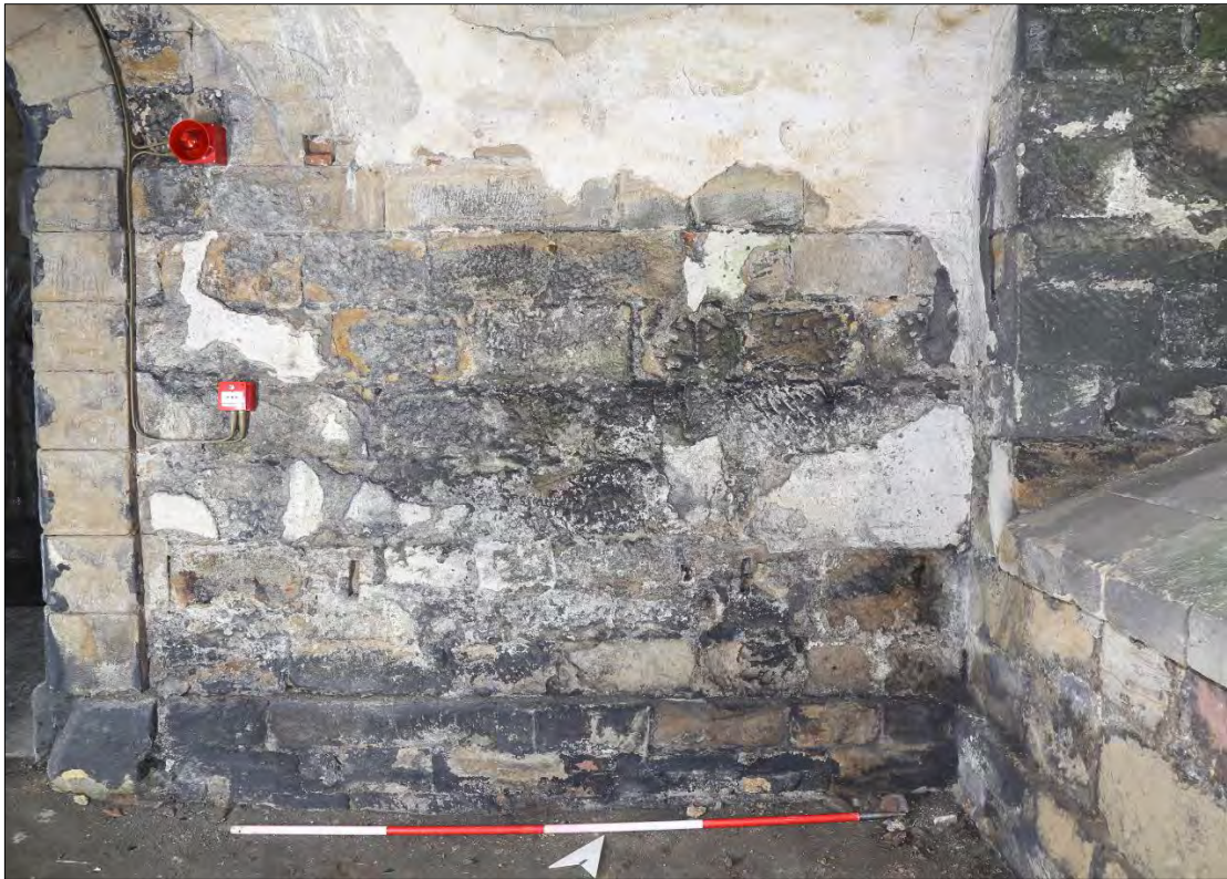
Plate 71: plaster (s201) preserved on the north wall of the pantry (B03).
