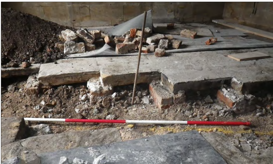
Plate 125: Carriage House floor structure; looking north-west.
