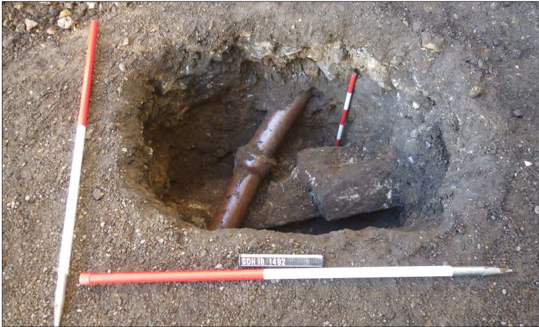
Plate 65: drain 32 with salt-glazed drain insertion.
