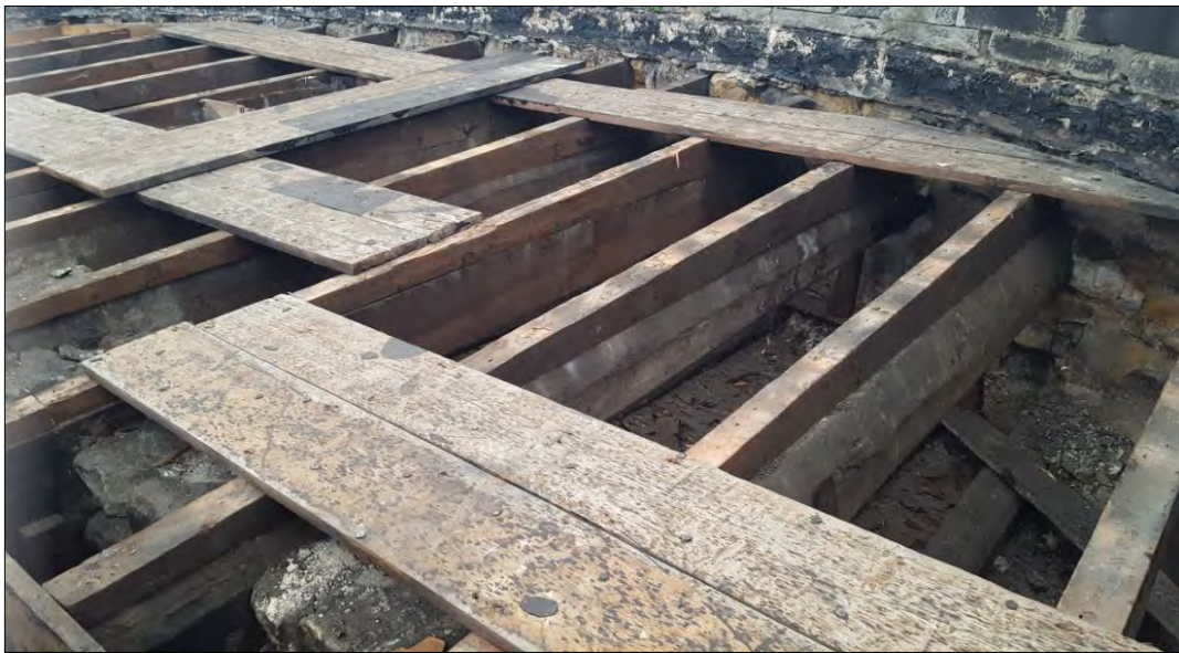
Plate 31: timber rafters associated with the apsidal bay (123). Later timbers have been added to the earlier rafters to increase the rake.
