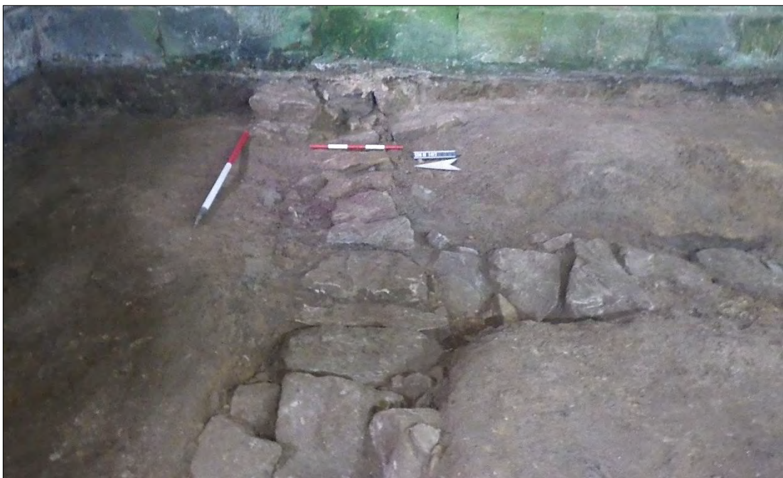
Plate 99: drain 136 and damage to the east wall caused during construction.
