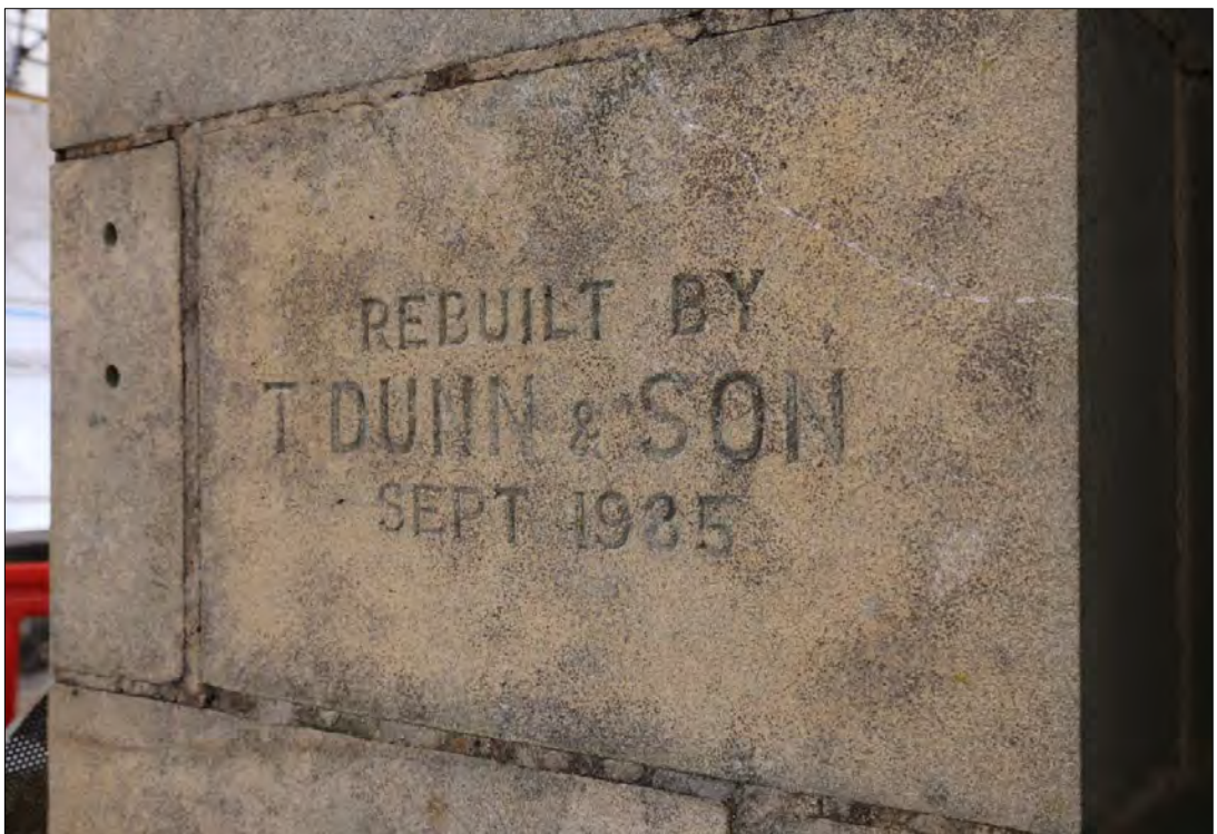
Plate 5: date stone referencing the restoration of the main south stack 103.
