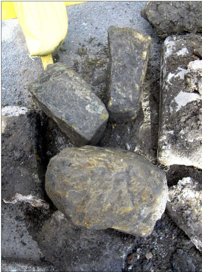
Yarm Bridge: displaced masonry from bridge repairs
