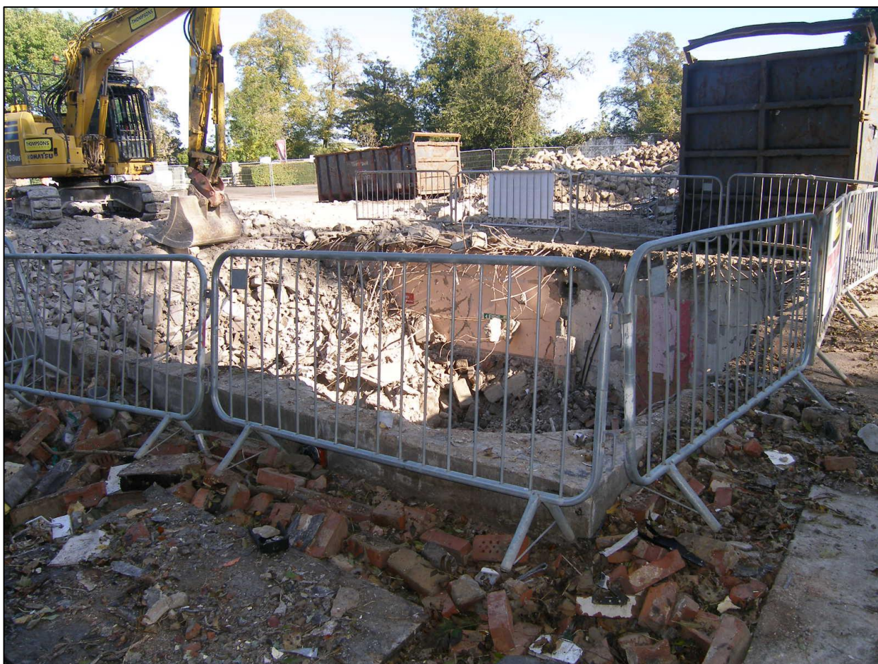
Plate 4: Infilling of the c.1970s cellar.
