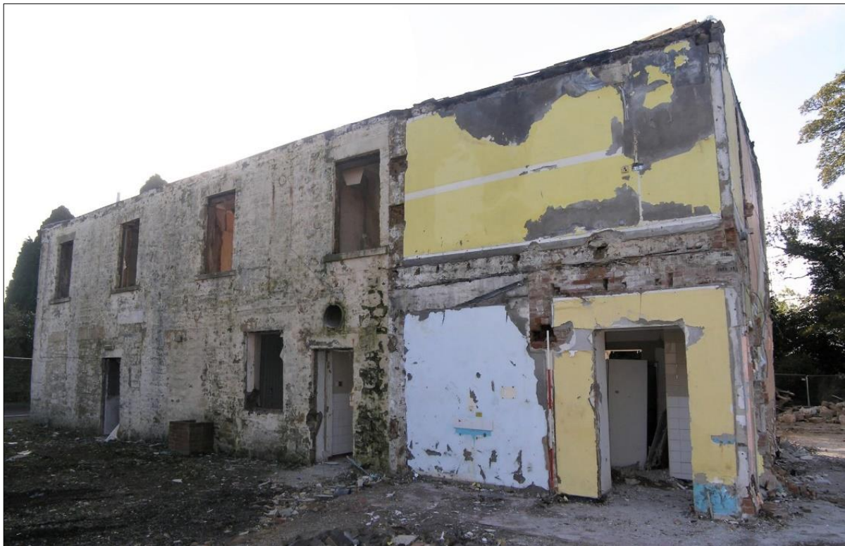
Plate 3: North-facing elevation of the 18th-century range after removal of later structures.
