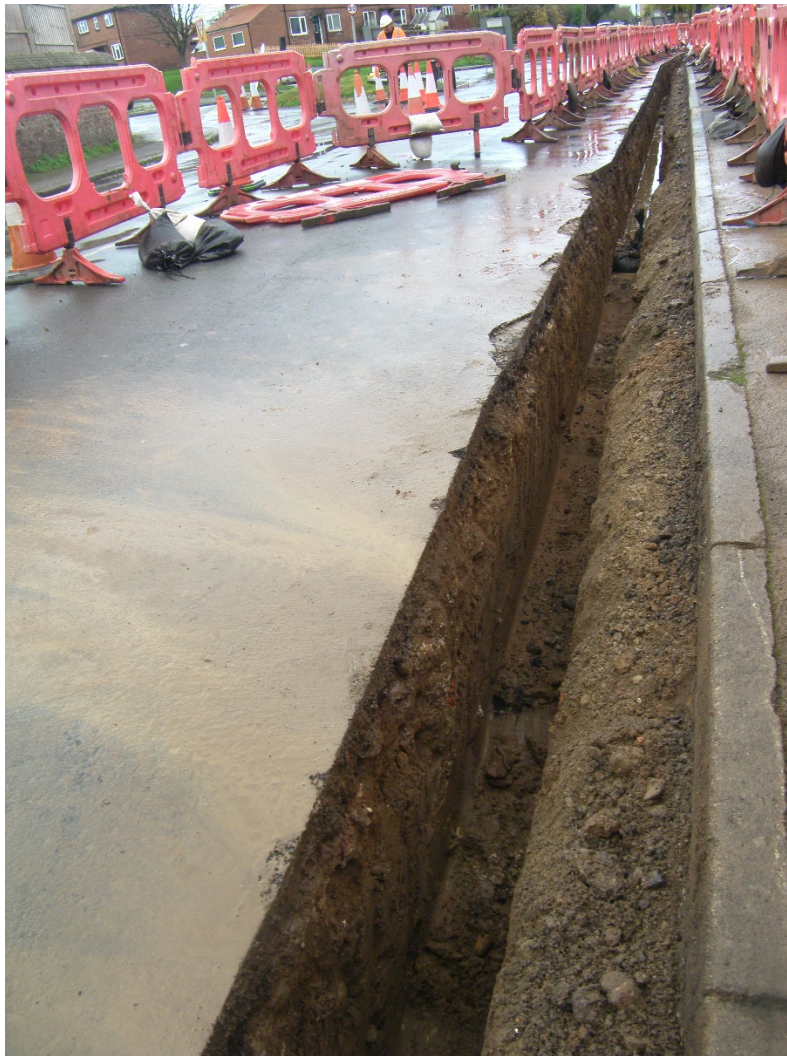
Plate 1: New Road pipeline trench, photo taken looking north-west.
