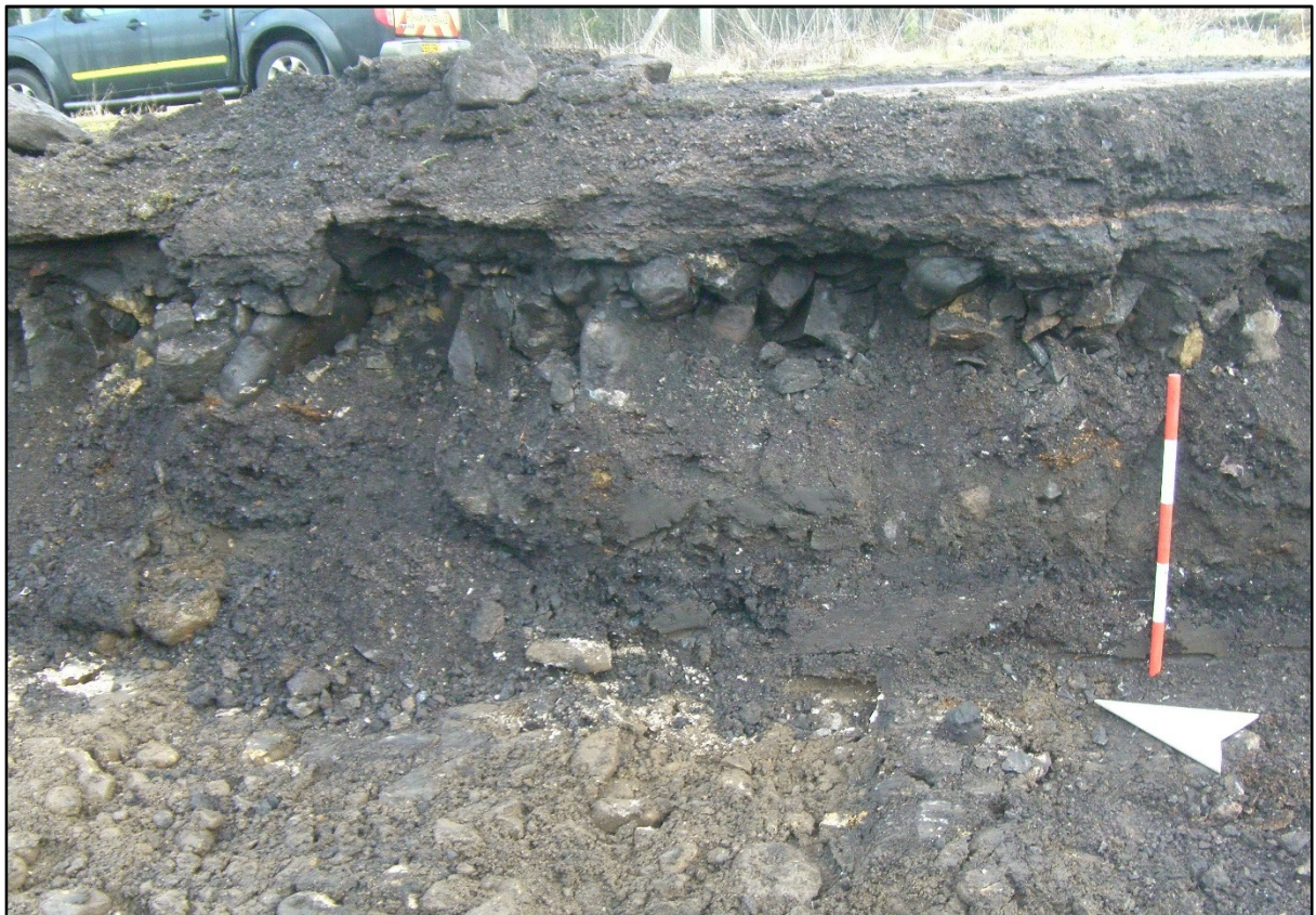
Plate 1: Representative section showing the natural alluvial stony silt 01 , thick refuse deposit 02 , stone setts 03 and tarmac surface 04 .
