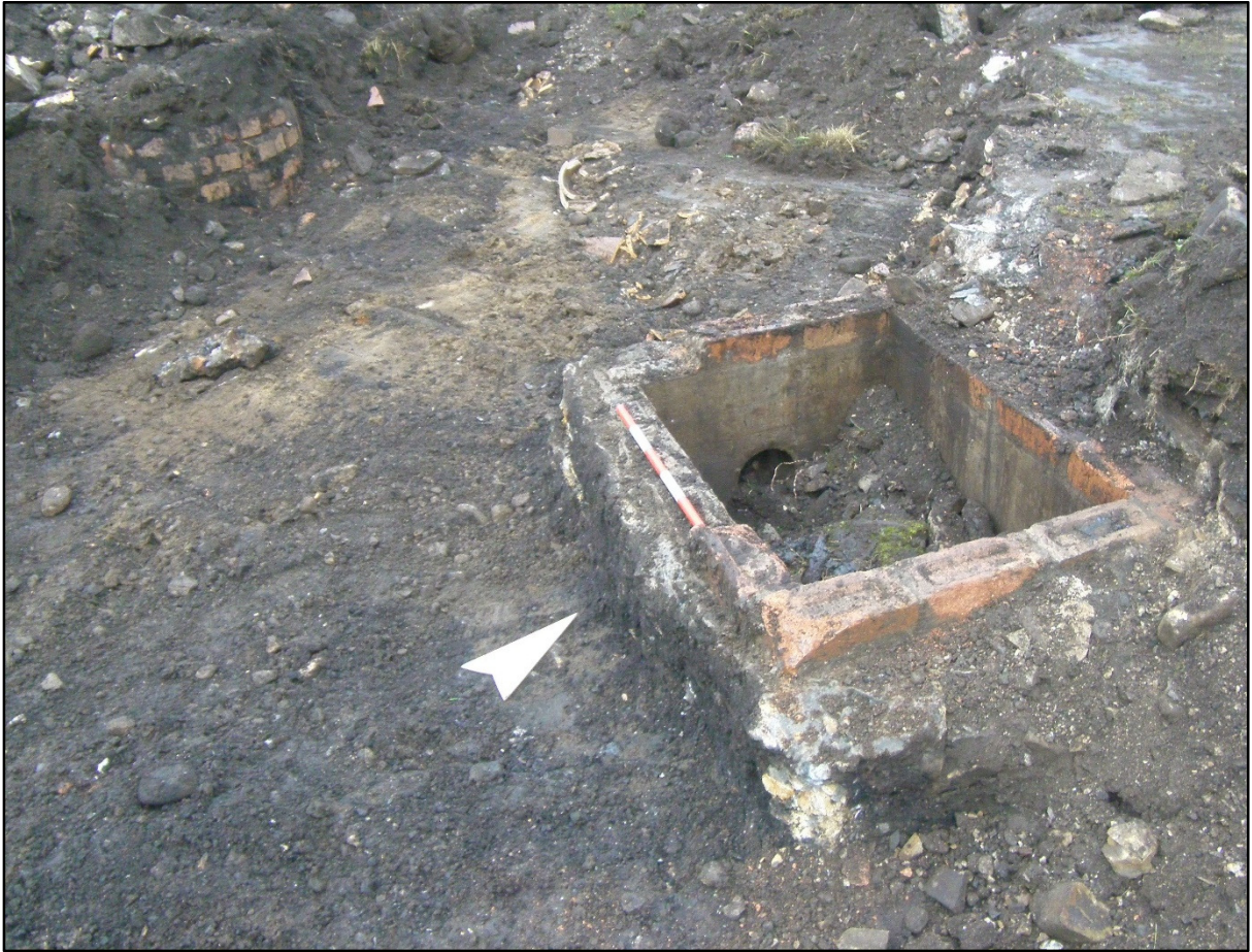
Plate 2: Modern brick and concrete inspection chamber and ceramic drains (09).
