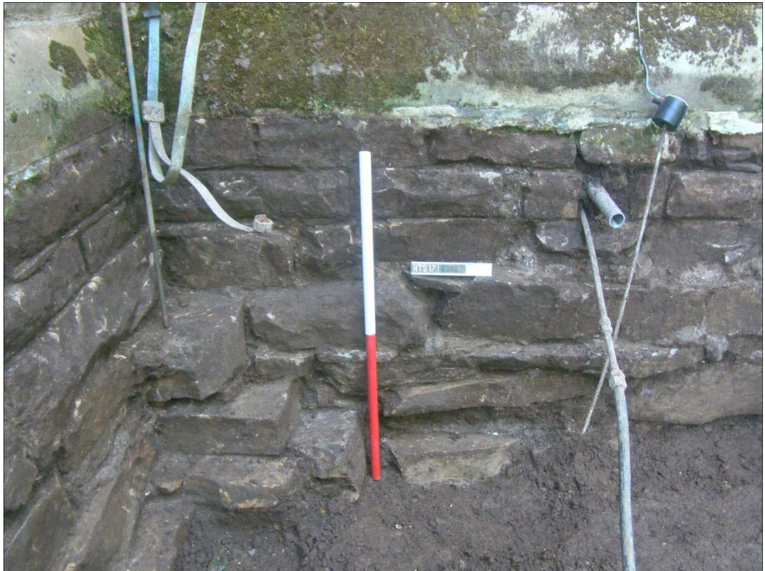
Plate 1. Church foundations overlying irregular masonry, possibly of medieval date
