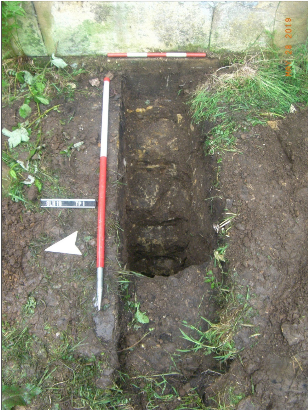
Plate 1: Trial Pit 1, showing wall foundation 5.
