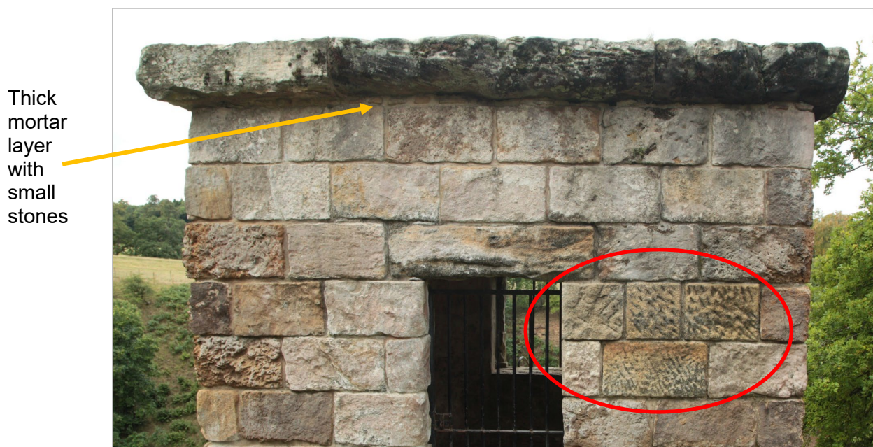
Plate 16: detail showing the inserted blocks (outlined in red) and the layer of mortar with stones.
