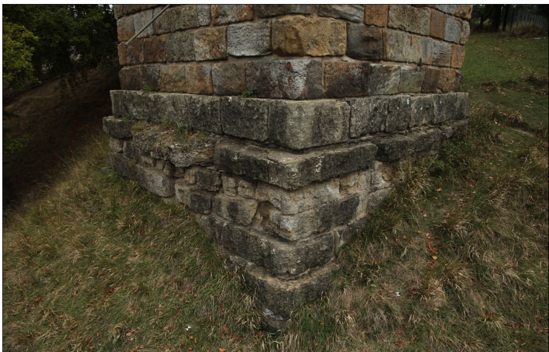
Plate 14: detail of the platform, showing how it is built into the steep slope.
