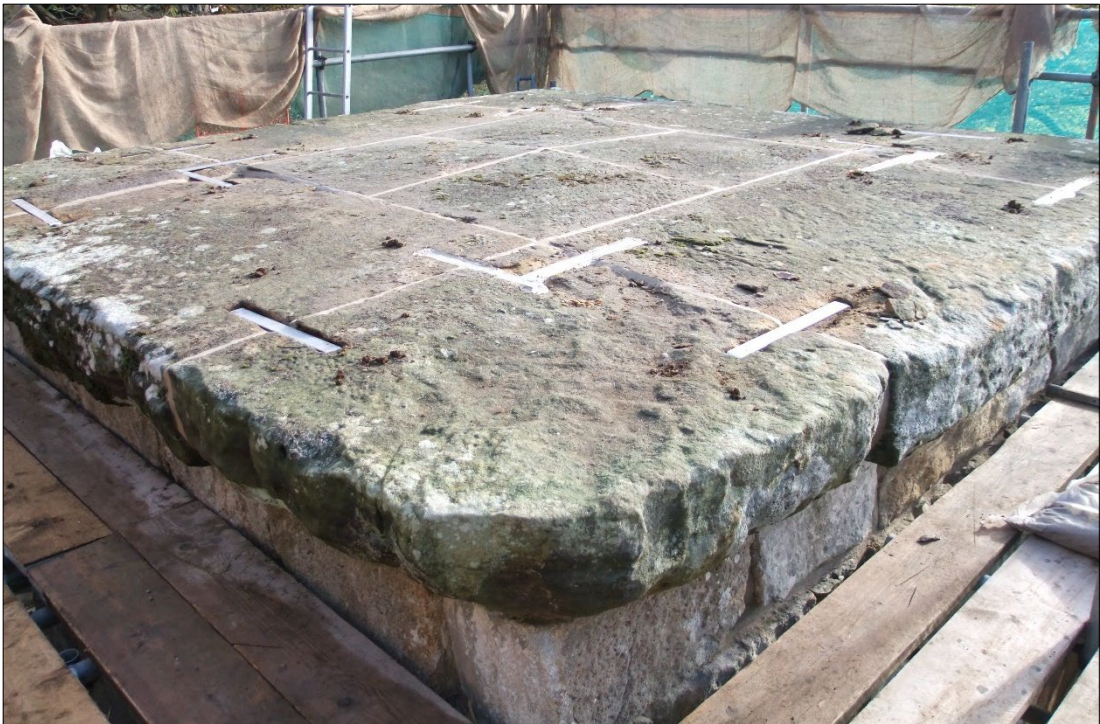
Plate 24: view of the roof during conservation work
