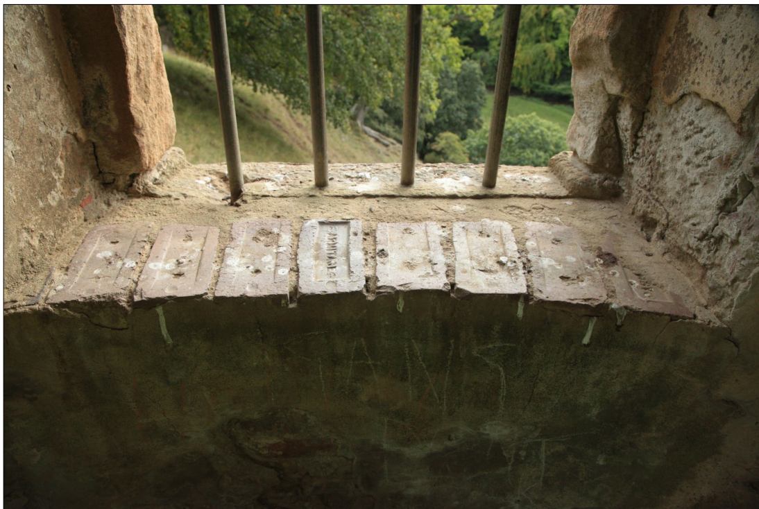
Plate 30: detail showing the repaired south-facing windowsill.
