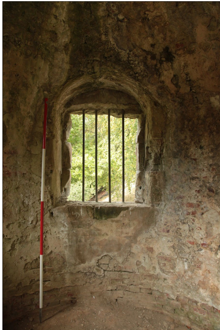
Plate 35: the north-facing window.
