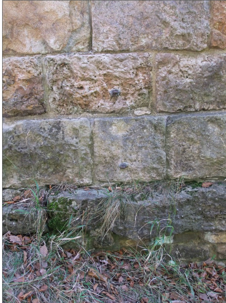
Plate 21: detail showing the metal the metal fence attachments.
