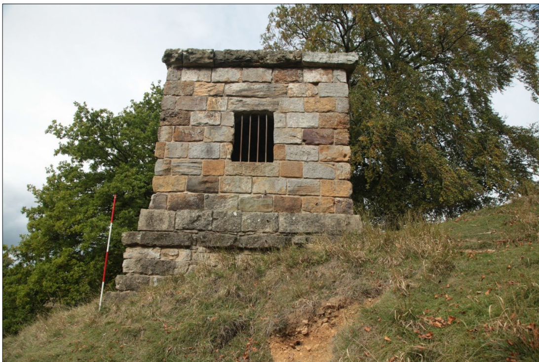
Plate 17: the south-facing elevation.
