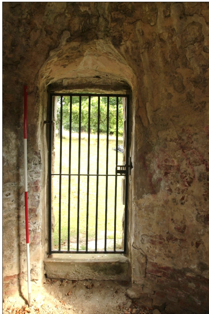
Plate 25: view of the doorway internally showing the threshold stone and the curved entrance ceiling.
