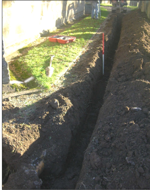
Plate 2 drain trench excavated past west end of church
