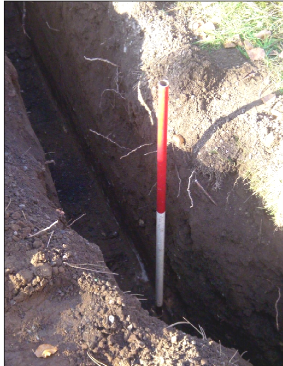
Plate 4 typical churchyard soil profile, at bend in drain trench
