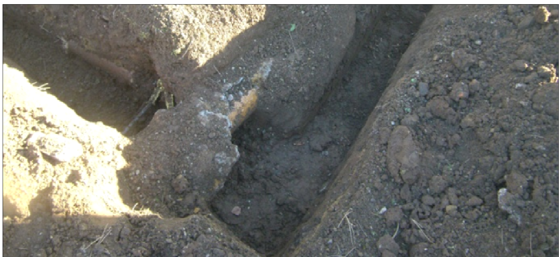
Plate 1 drain trench showing existing draining and services
