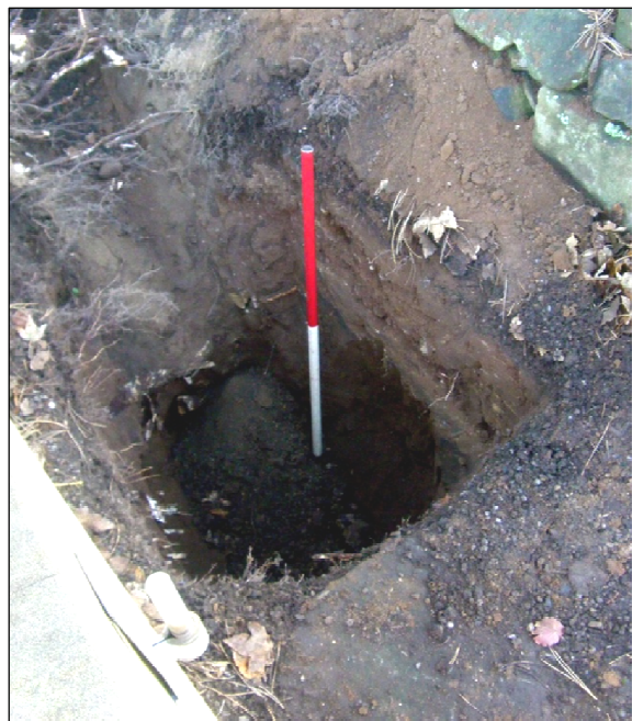
Plate 5 manhole excavation soil profile
