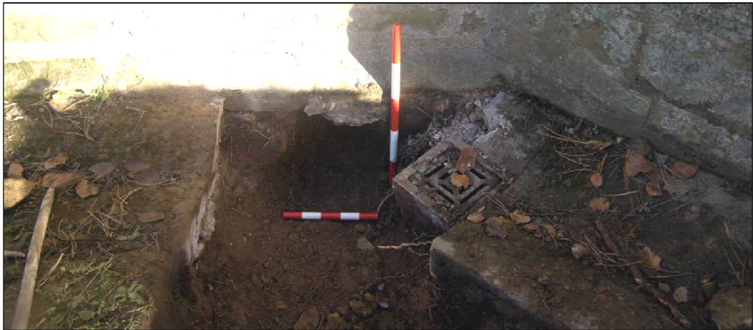
Plate 6 hole cut through west nave wall
