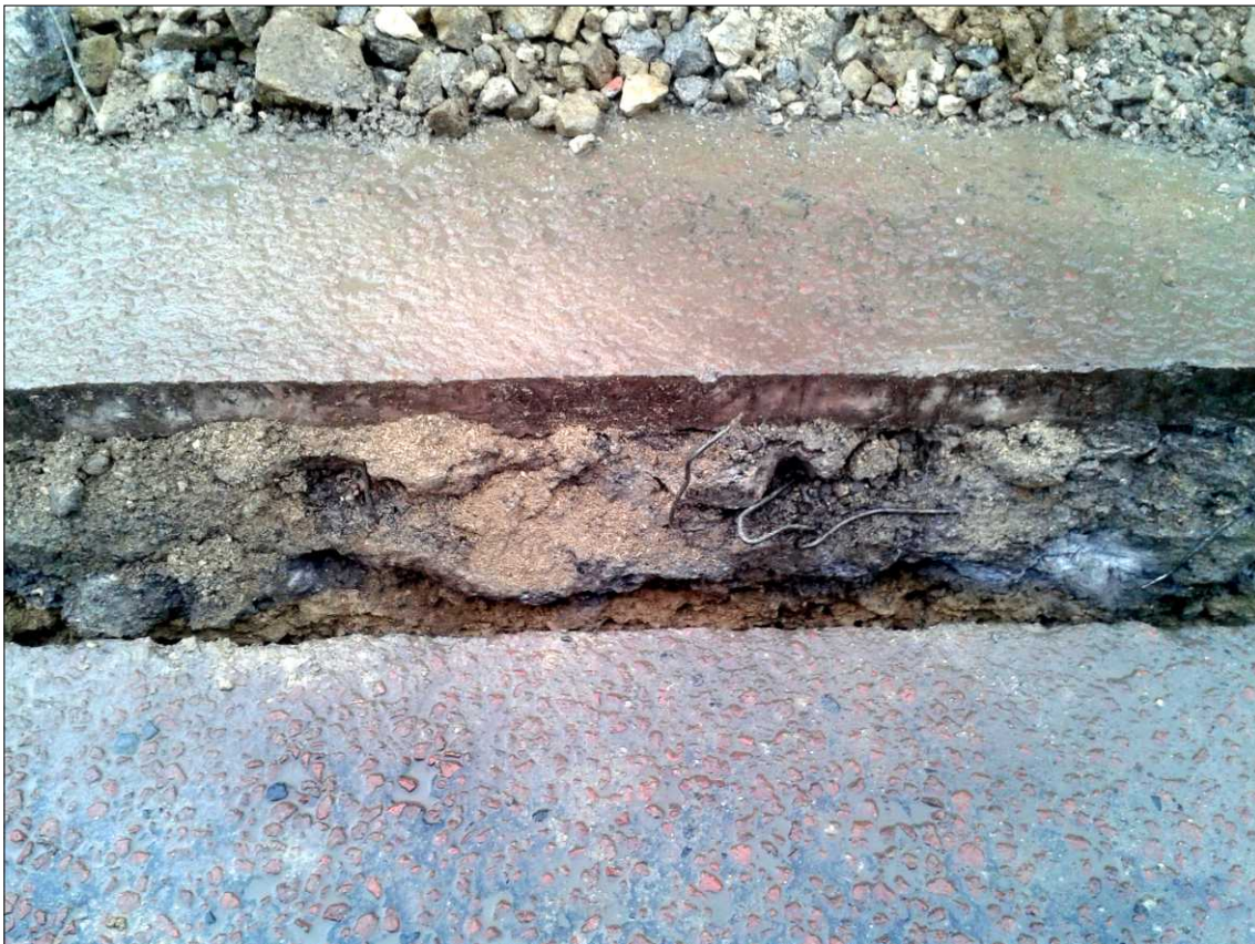
Linden Way, Gateshead: close up showing concrete below tarmac Plate 2
