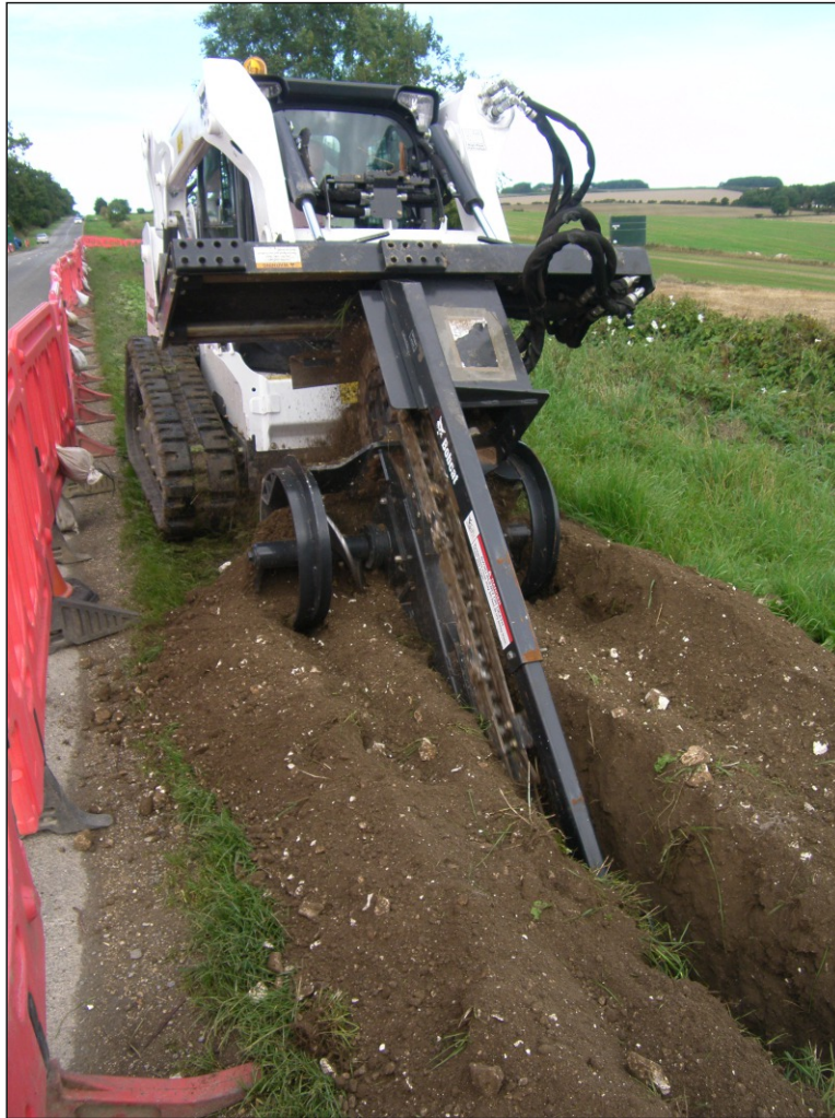
Huggate: trenching machine in action
