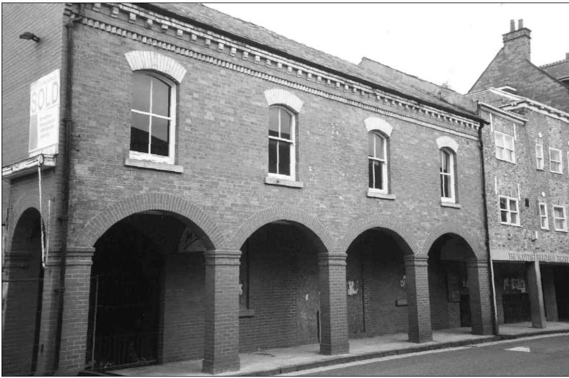
Figure 10 Elevation of 17 Skeldergate (looking east, June 1999)
