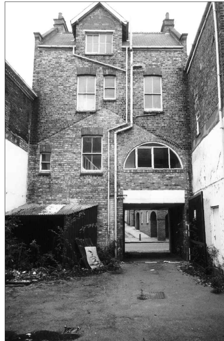
Figure 13 Yard-facing elevation of 19 Skeldergate (2 x 2 m scales, looking south-west, August 1999)
