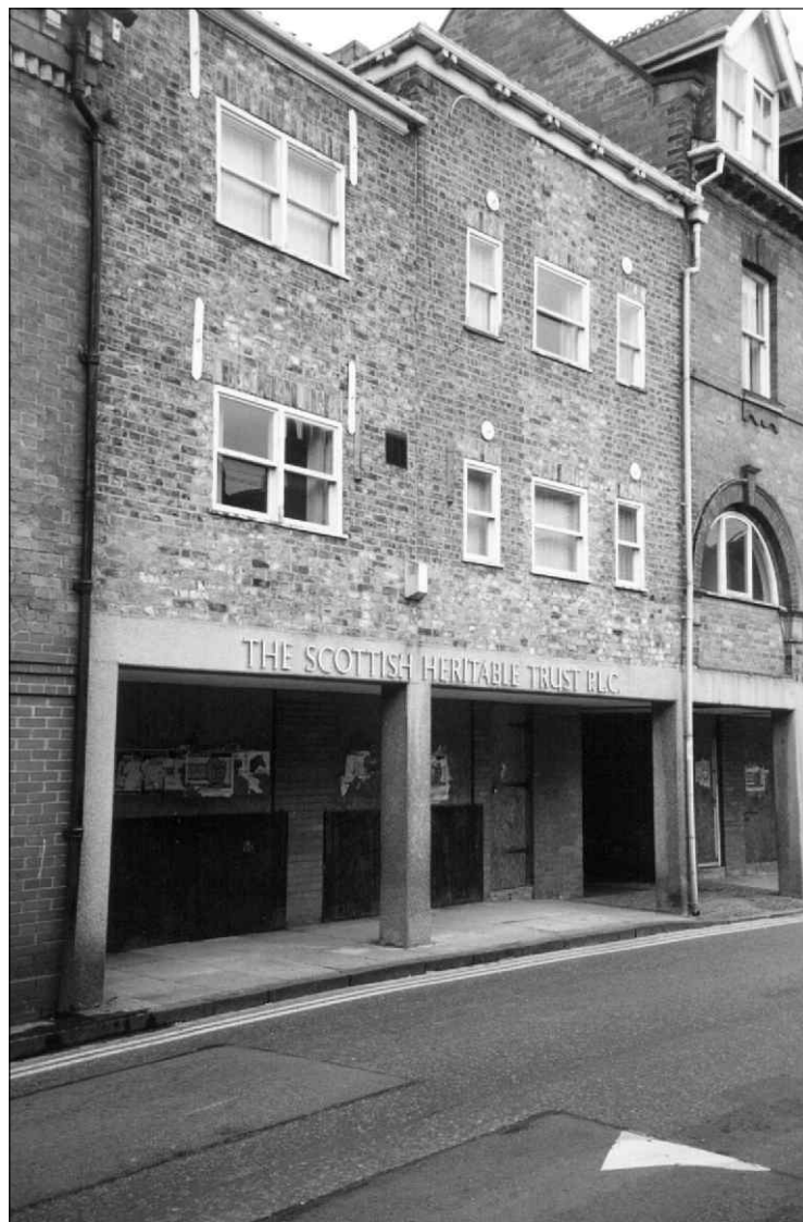
Figure 11 Elevation of 18 Skeldergate (looking east, June 1999)
