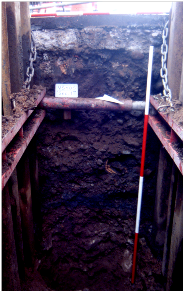
Plate 4 Micklegate, York: north-east facing section of Trench 1 showing complete sequence of road surfaces.
