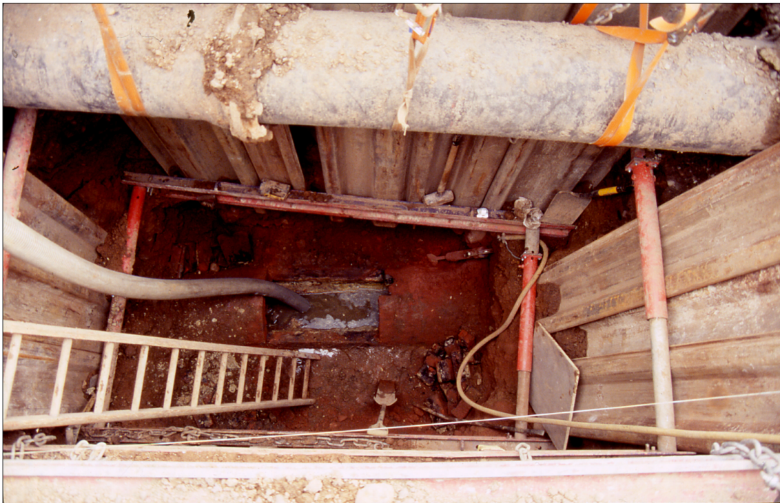
Plate 6 Micklegate, York: the Victorian tunnelled sewer in the base of Trench 2.
