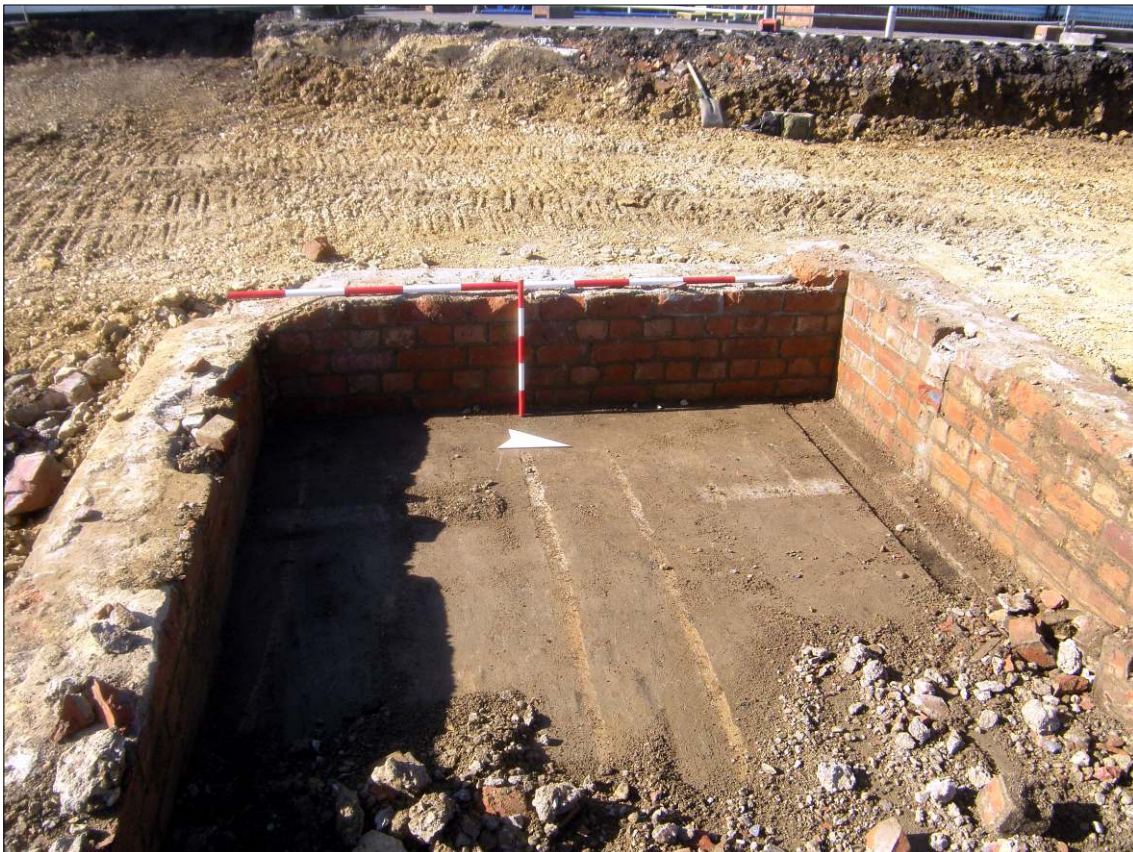
Kirk Merrington Primary School: air-raid shelter showing concrete floor, scar of interior wall and drain
