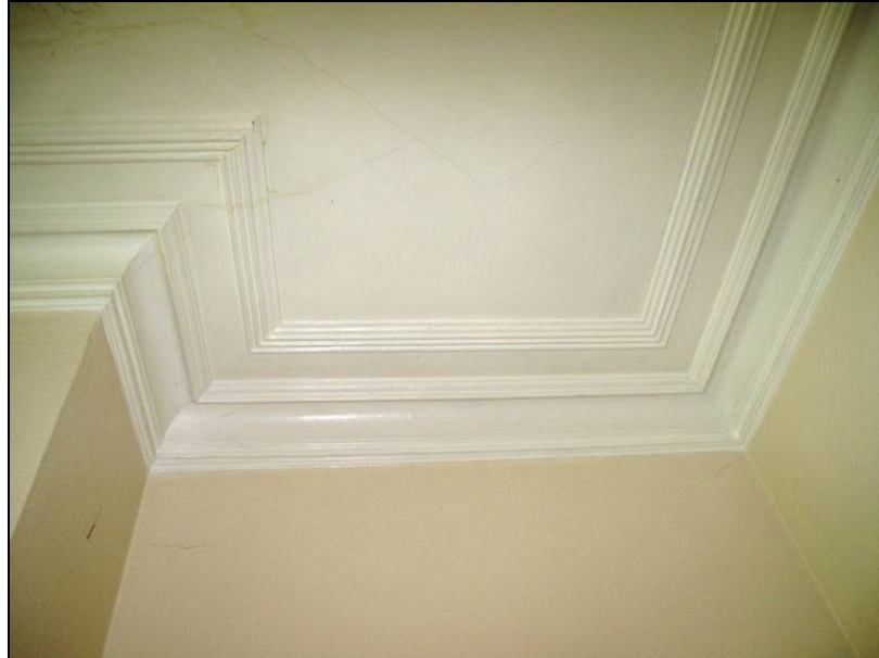
Plate 19: detail of coving, Room 1
