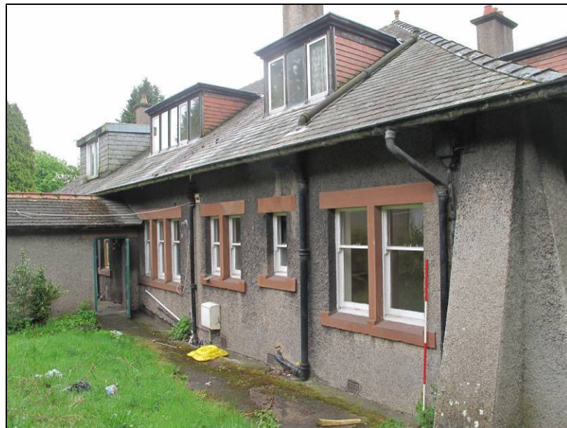
Plate 11: the windows in the north-east facing elevation
