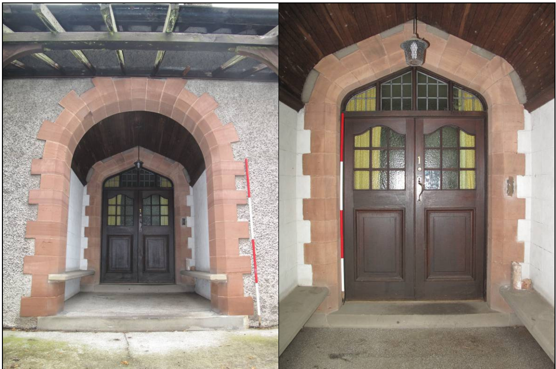
Plate 8: the porch and front door, facing north-west
