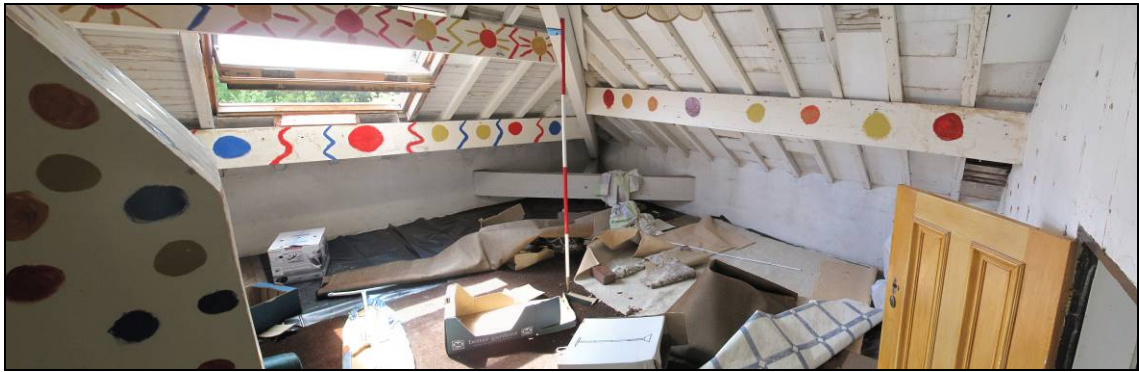
Plate 27: Room 20, facing west
