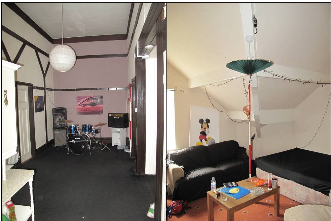
Plate 26: exposed beams on the landing (left) and in Room 23 (right)
