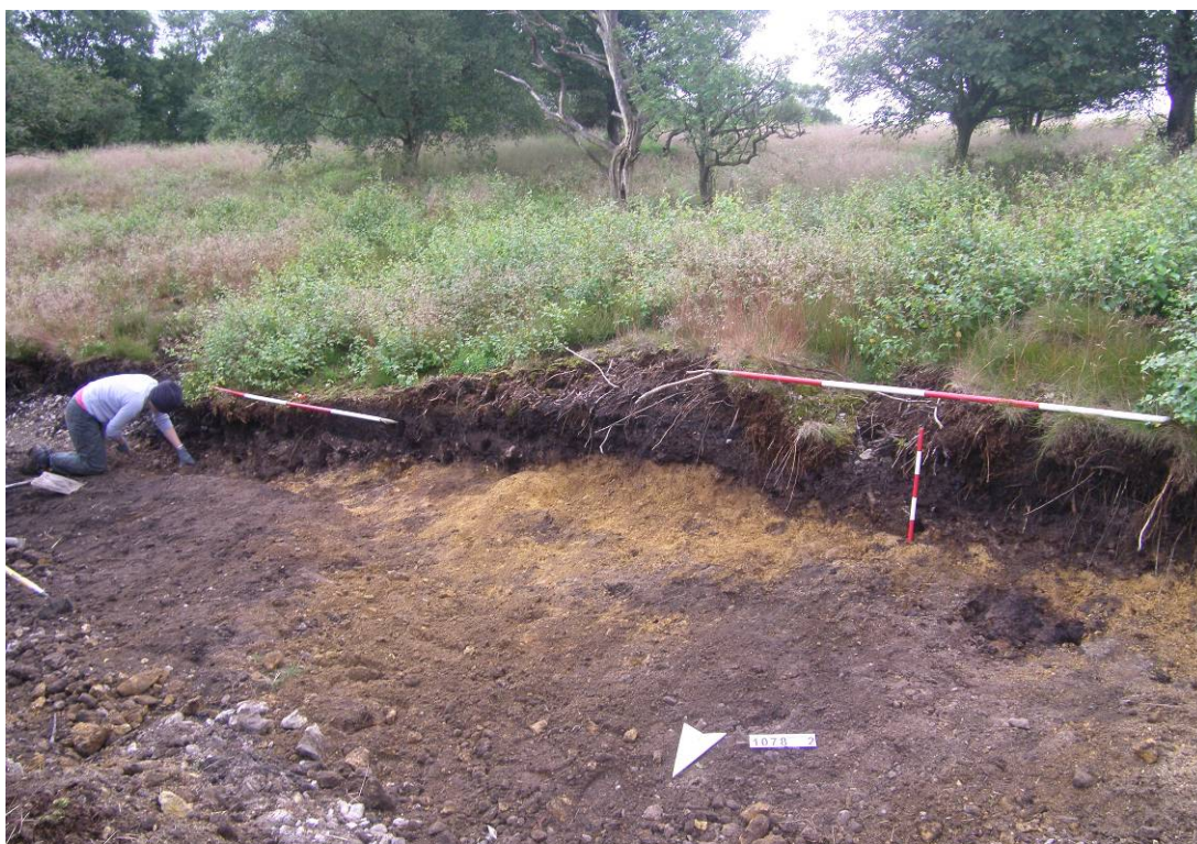
Plate 6: Section 2, facing south-east.
