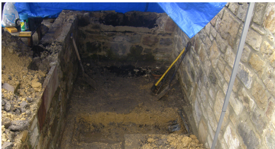
Plate 2: East facing view showing location of foundation trench and depth of levelling gravel (101)
