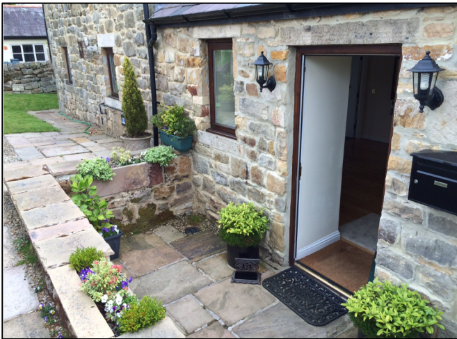
Plate 1: Halton Barn - view of existing door and area of new porch with drain in far corner between the house and retaining wall
