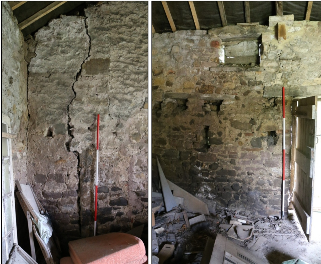
Plates 15 and 16: the wall scar in the north-west wall of Bay 3, where the internal wall of the Phase 1 building was extended southward in the late 19th century, and the in-built timber and joist holes demonstrating the position of a former loft level in Bay 3
