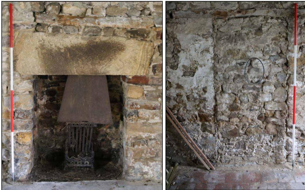
Plates 10 and 11: the fireplace in the south-eastern wall of 1G, and the blocked original doorway in the north-western wall of the same room, showing the tiled flooring in this area
