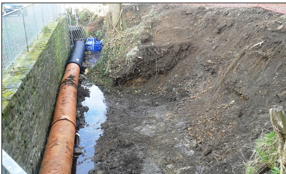
Plate 4: excavated sections of bank edge to accommodate trash screen, facing south
