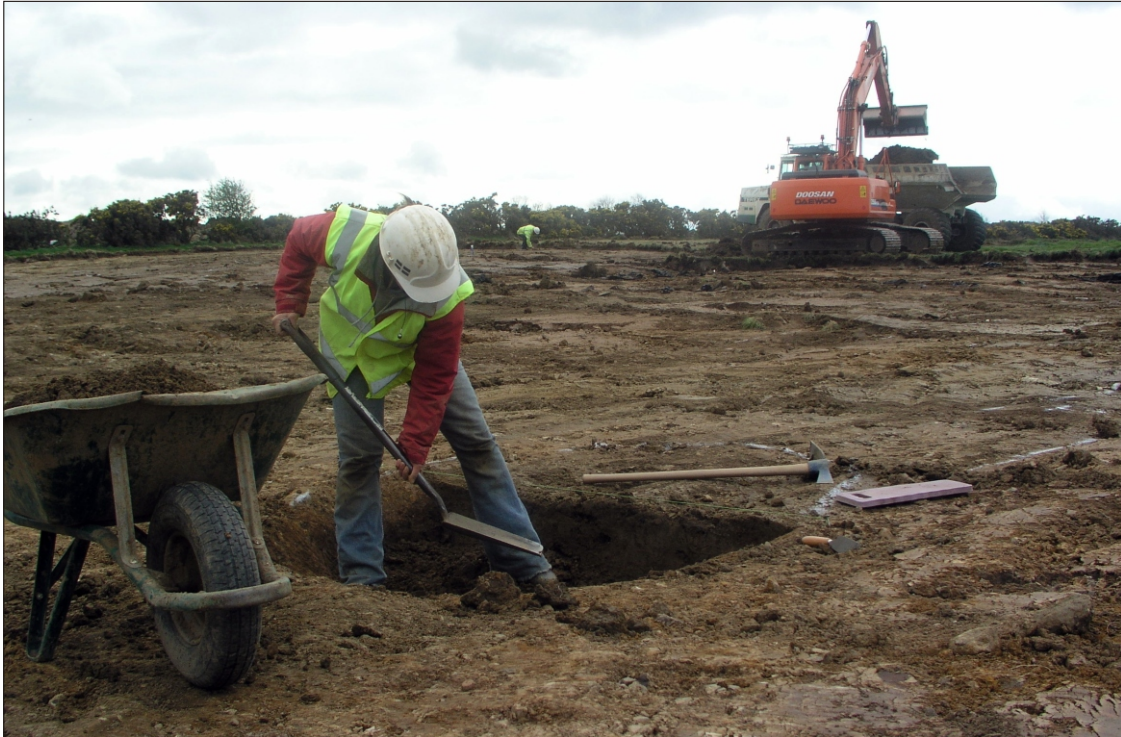
Plate 1 North Stobswood, Northumberland: hand excavation of feature with machine stripping in the background
