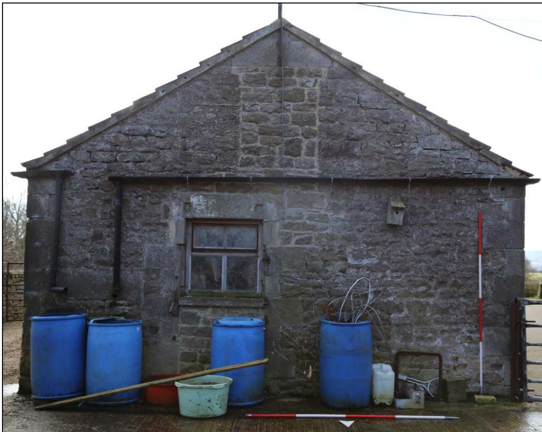
Plate 5: North elevation of the cart shed
