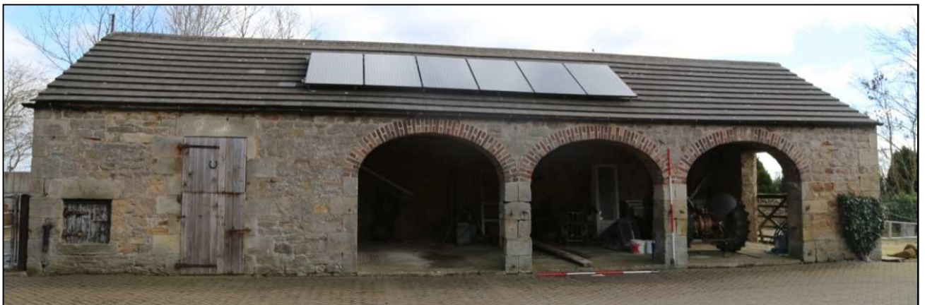
Plate 11: West elevation of the cart shed
