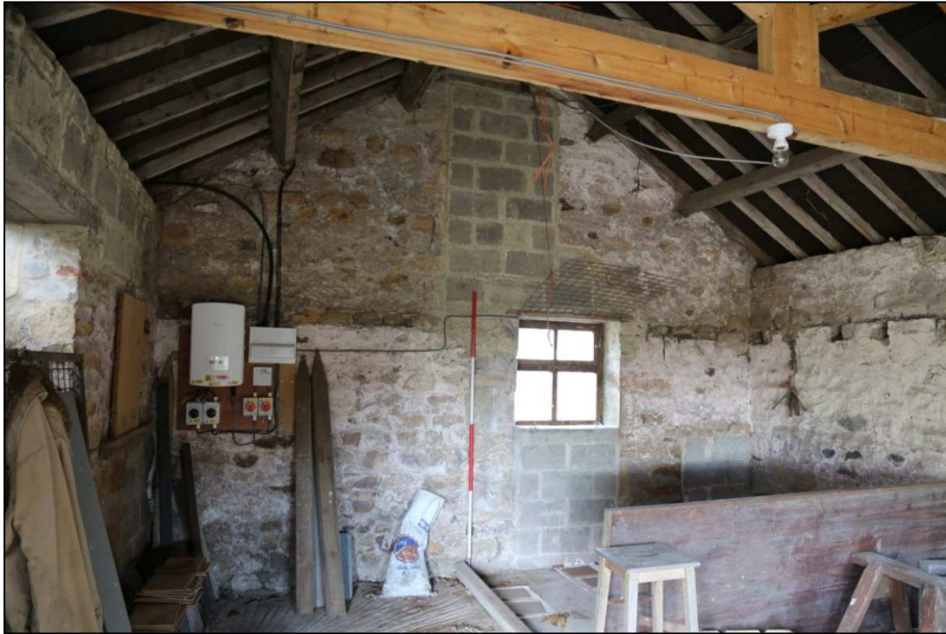
Plate 13: Internal north wall of the cart shed
