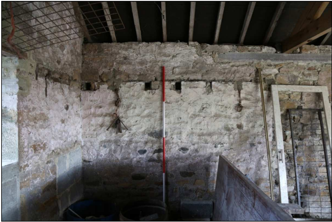
Plate 14: Evidence of a former loft in the north-east corner
