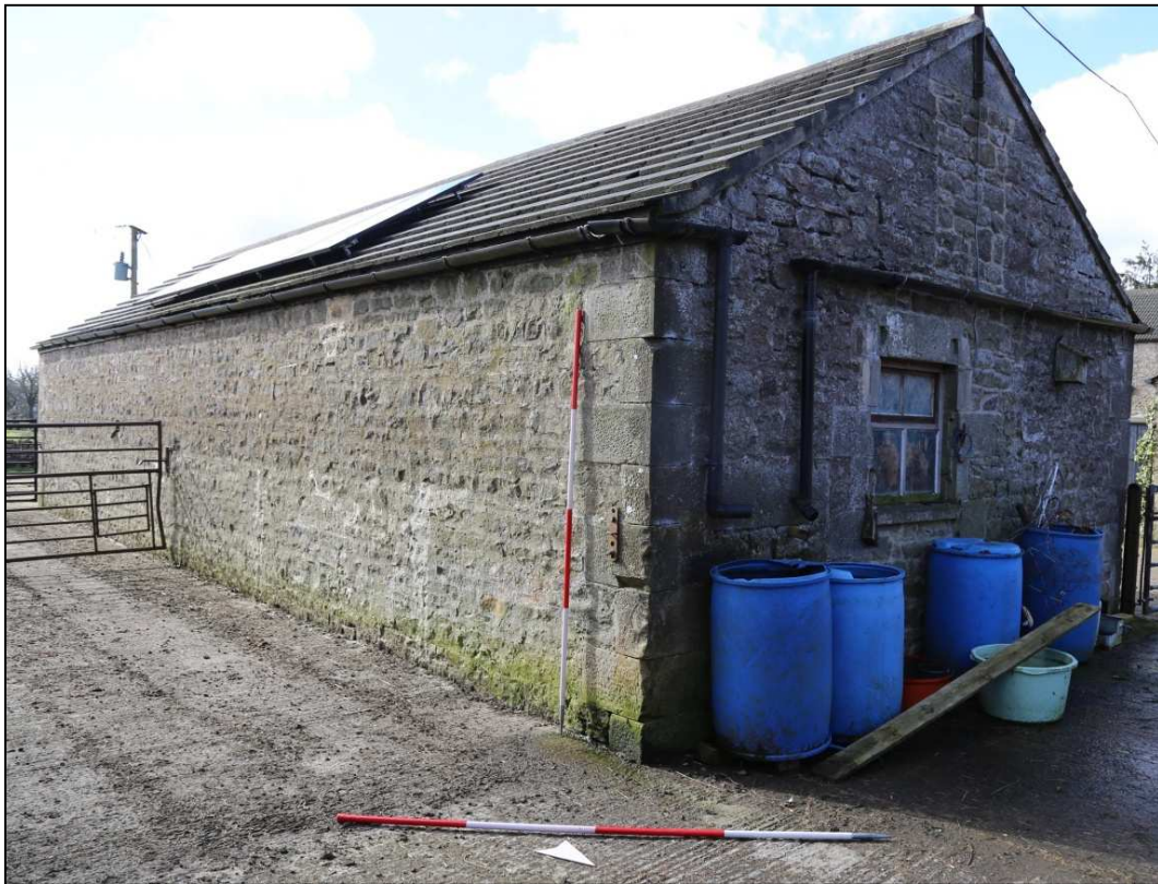
Plate 6: Oblique view of the east elevation of the cart shed, looking south-west, with the north elevation to the right
