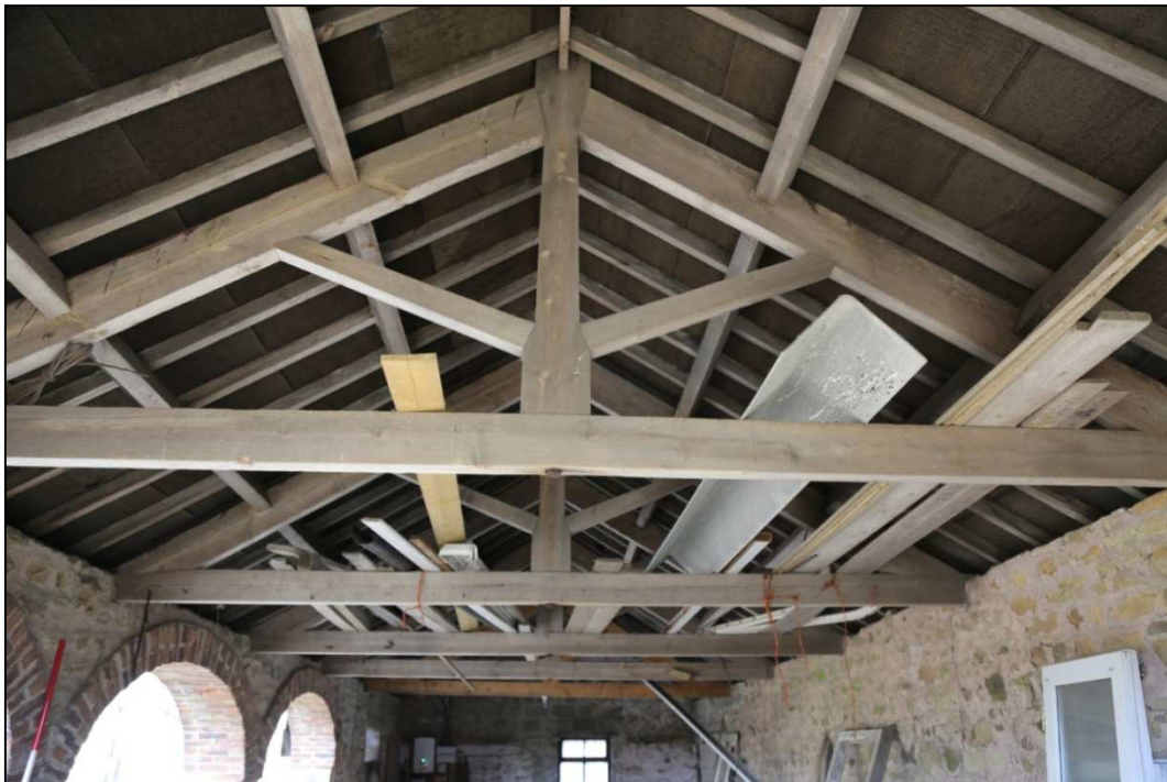
Plate 12: Modern timber roof structure, looking north
