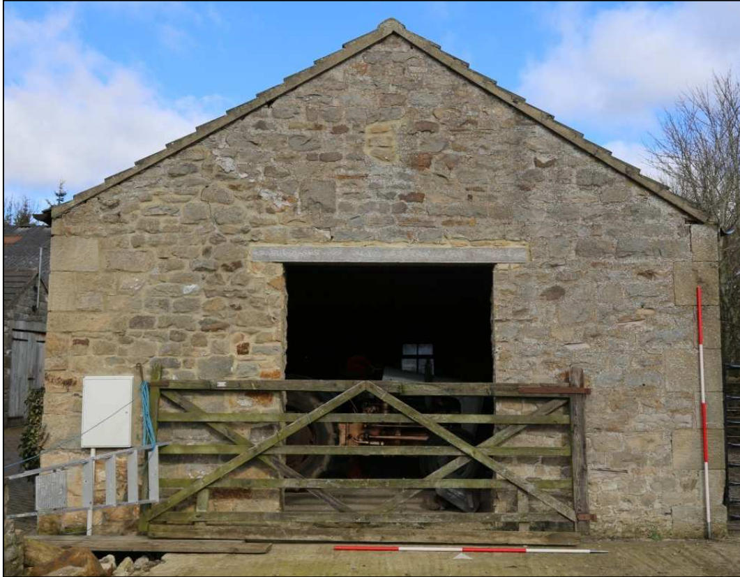
Plate 8: South gable of the cart shed
