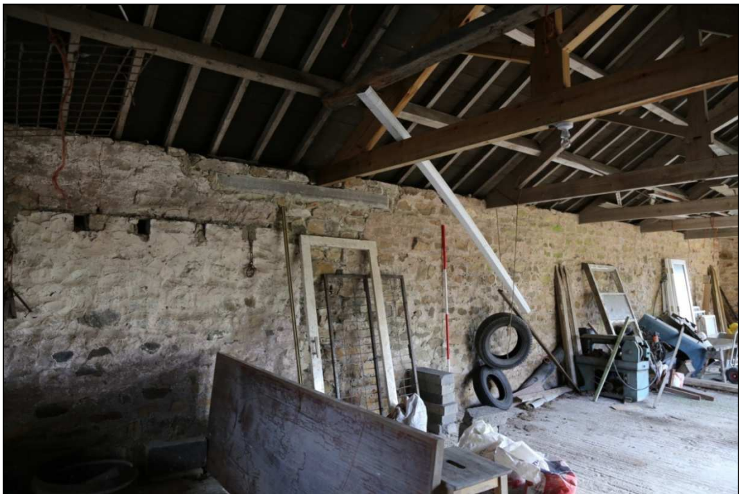
Plate 15: East wall of the cart shed, looking south-east
