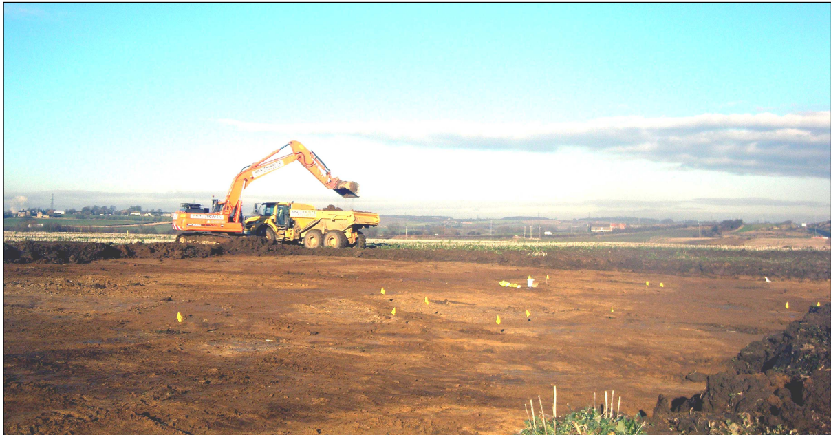
Plate 1: General view of site during the monitoring of soil stripping
