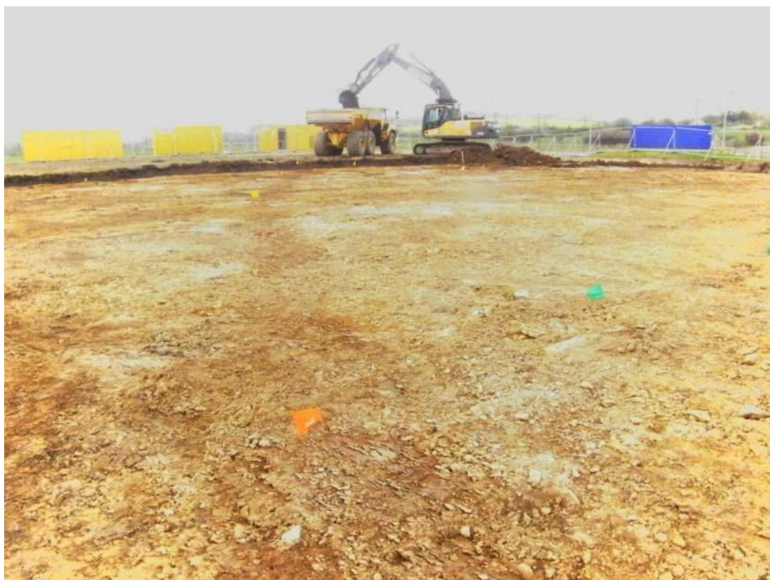
Plate 9: View of ditch 65 during stripping (looking west)
