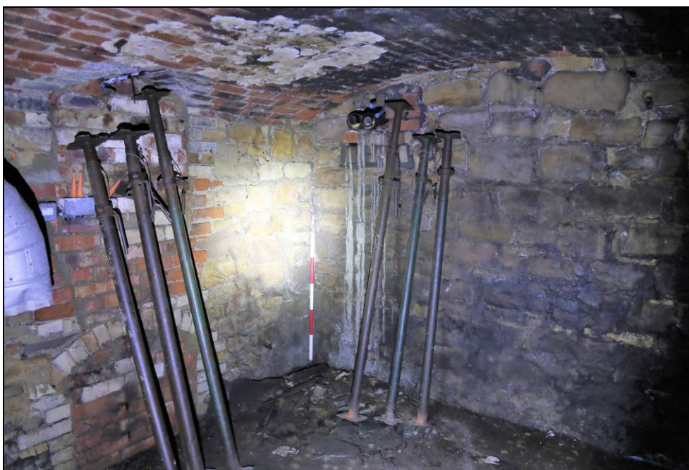
Plate 15: boiler room, with blocked firemouth and later alteration above
