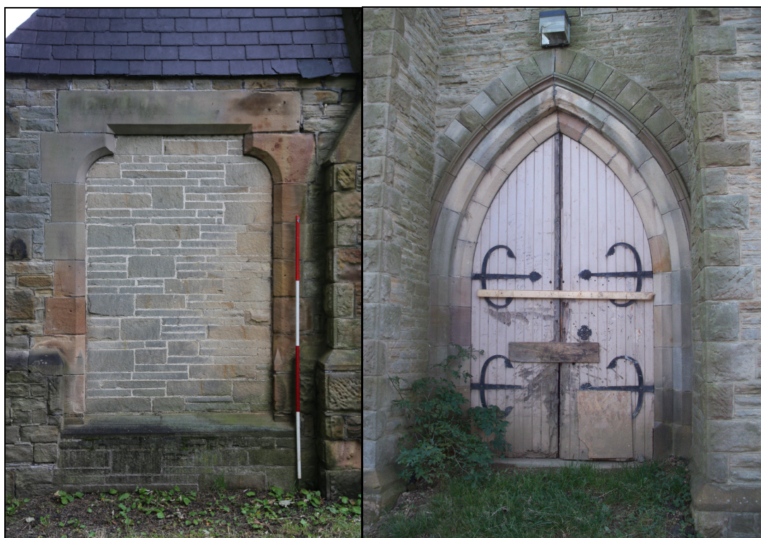
Plate 19: blocked doorway to narthex (left) and doorway into church tower lobby (right) (© Stubbs Family 8 )
