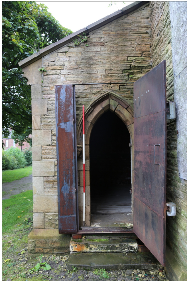
Plate 20: external doorway into north transept
