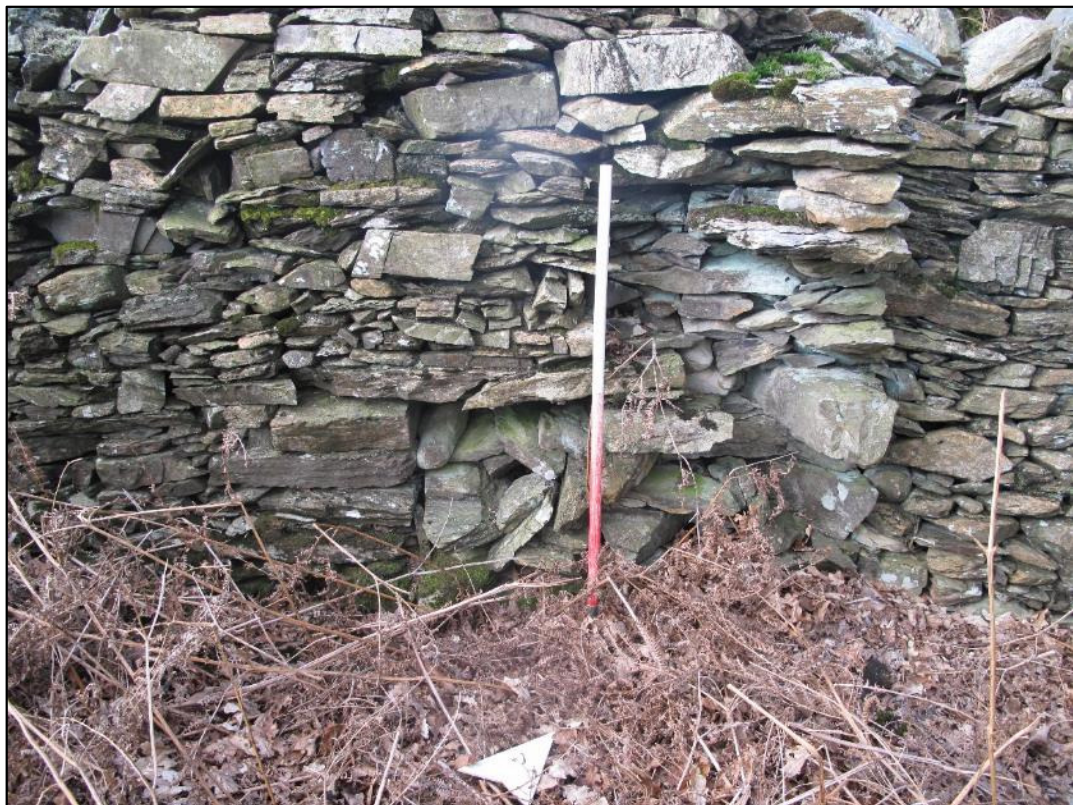
Plate 72: blocked hogg hole leading out to Bethocar Moor and vertical seam (right) of two adjoining walls in possible former sheepfold (16/014).
