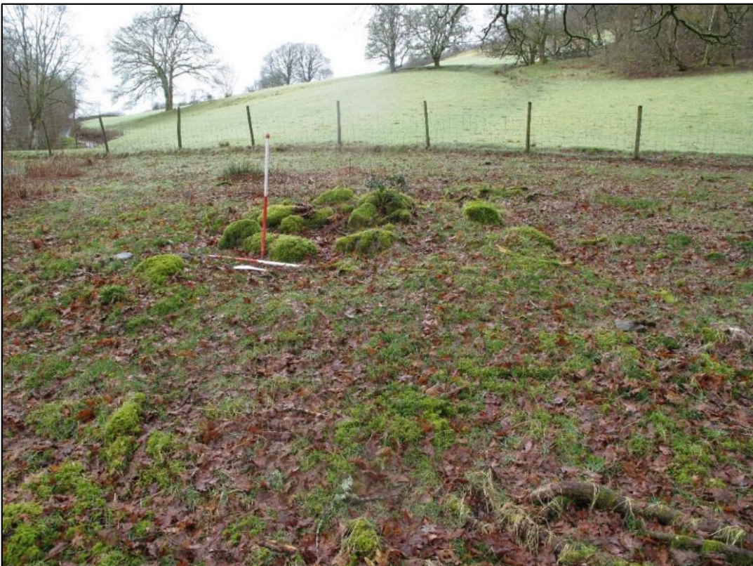
Plate 67: a circular, single-celled hut with turf wall foundations and a stone hearth structure (18/046)
