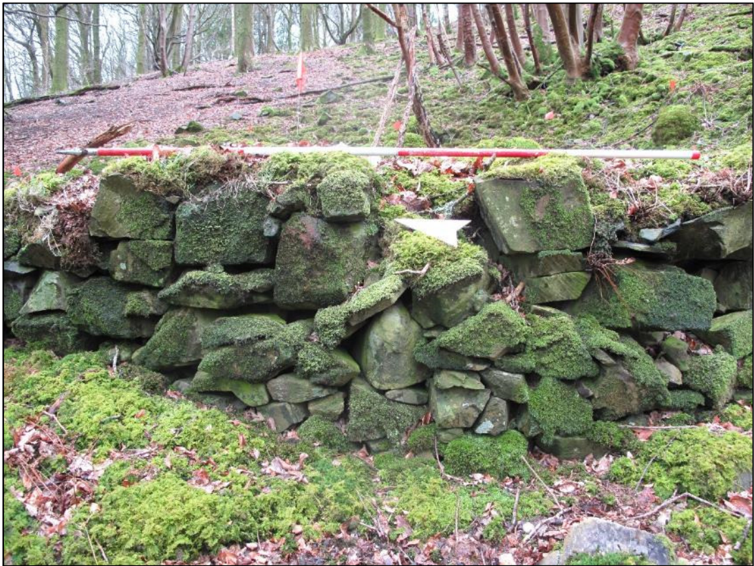
Plate 55: the well-constructed revetment wall of pitstead 25/002 in Near Plantation wood.
