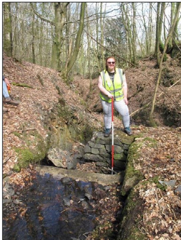
Plate 75: the pair of dams and associated concrete platform (right) that are likely to be a post-medieval sheep dip (27/023).
