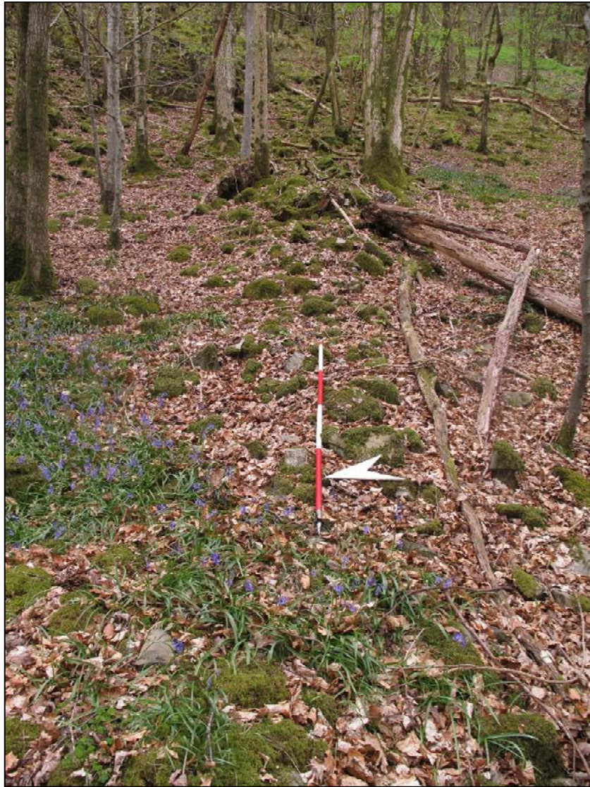
Plate 84: a collapsed and moss-covered wall in High Wood (5/062). Further investigation into the nature of these boundaries could reveal evidence of woodland ownership or management regimes.
