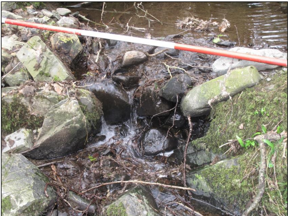
Plate 71: the dam that made up part of the water management system (24/022) in Towers Wood
