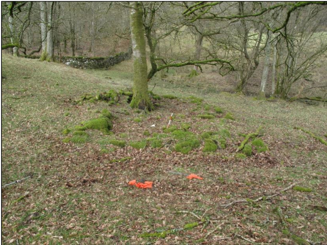
Plate 74: the ruinous structure (19/008) identified in Tom Parrocks wood that was likely a small field barn.
