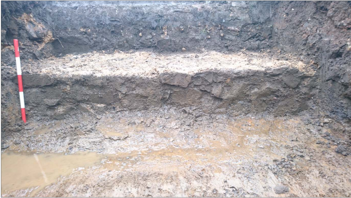
Plate 3: Lower site, Test Pit 1. West-facing elevation of wall 18 showing irregular coursing of Whinstone blocks.
