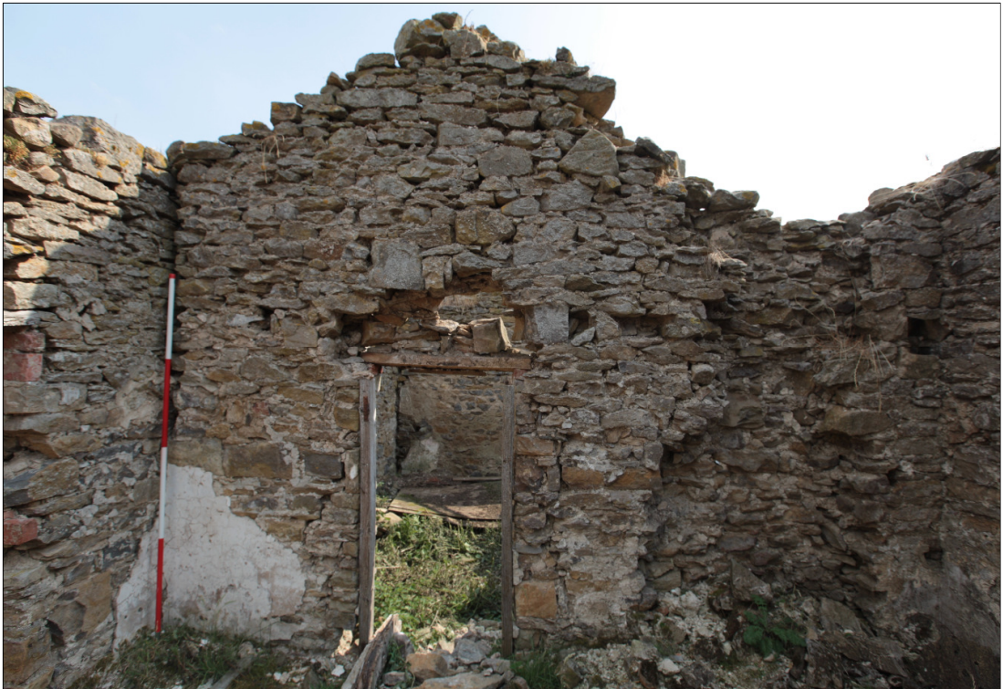
Plate 15: south wall of the north-central room (2200) showing door (2231), remains of internal wall plaster (2233), and possible remains of a fireplace (2234); this area may have formerly been sub-divided from the barn as part of the domestic living space.
