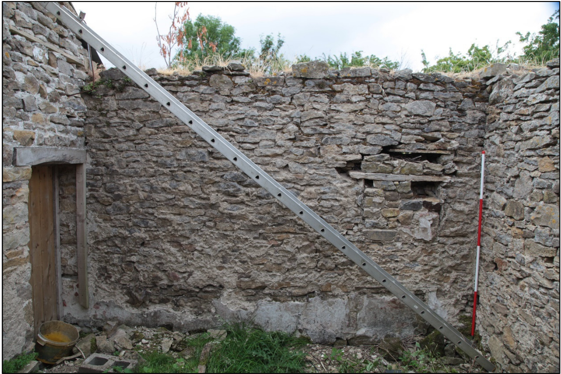
Plate 17: west wall of the south-central room with the blocked window (2421) visible above a square scar in the plaster.
