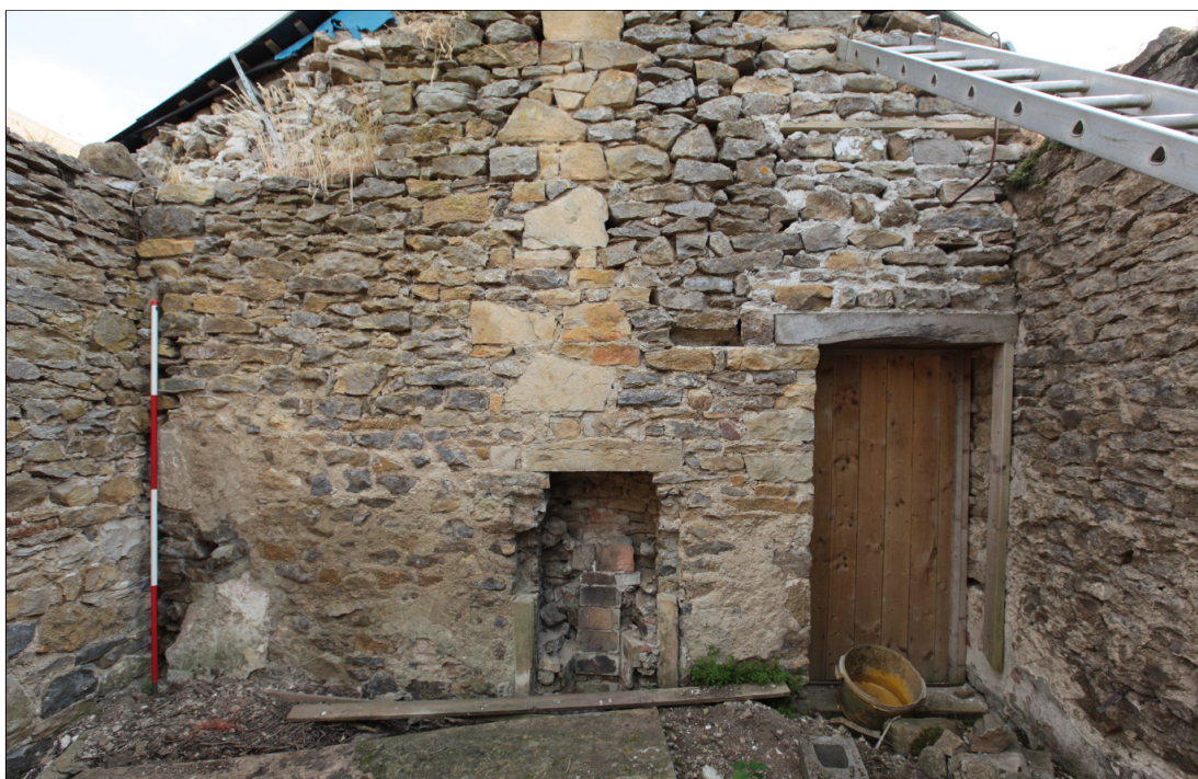
Plate 16: south wall of south-central room (2400) showing fireplace (2432), flue scar (repaired) and door (2431).
