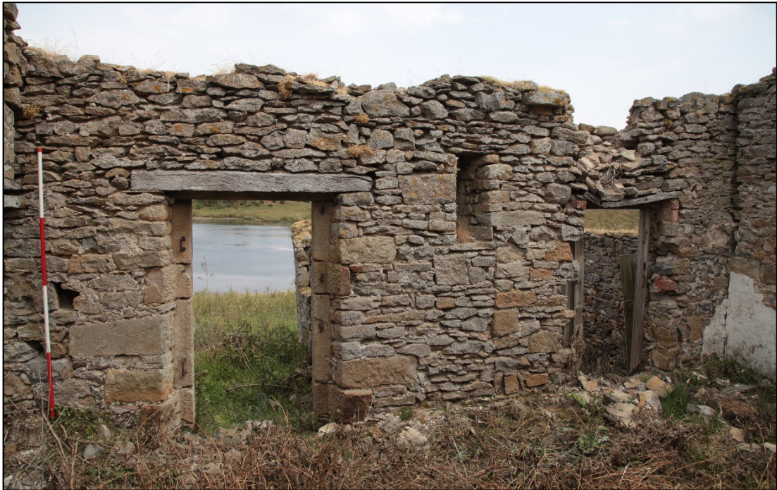
Plate 13: east wall of north-central room showing (from right to left) the exterior door, ventilation slit, wall scar and interior door to the eastern addition.
