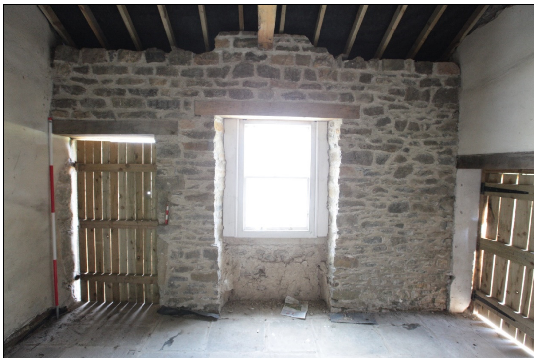
Plate 18: east wall of the southern room (2500). Wall scars are visible in the plaster of the north and south walls. Beside the main door is a small niche, indicated by the 0.25m ranging rod.
