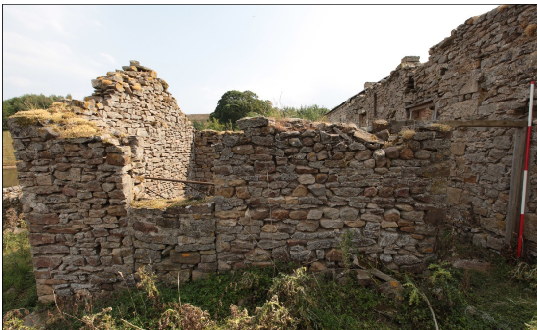
Plate 9: north elevation of east projecting wing (2300) showing the existing door (1311) and a blocked doorway (1111), now a window.
