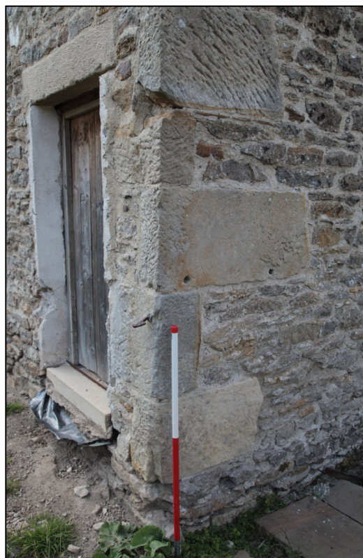
Plates 7 and 8: setting for gatepost (1406) and square settings in quoins (1407).
