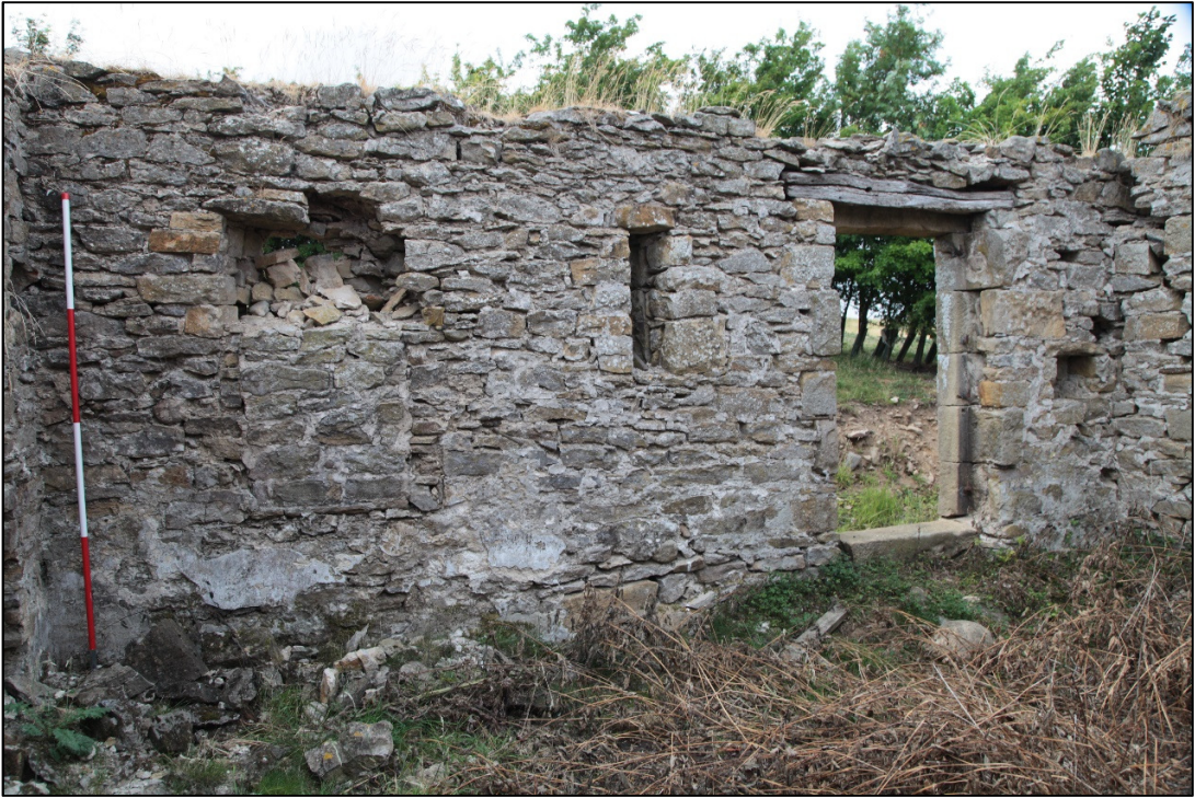
Plate 14: oblique view of the west wall of the barn showing (from right to left) several niches, the exterior door, ventilation slit, and blocked window.
